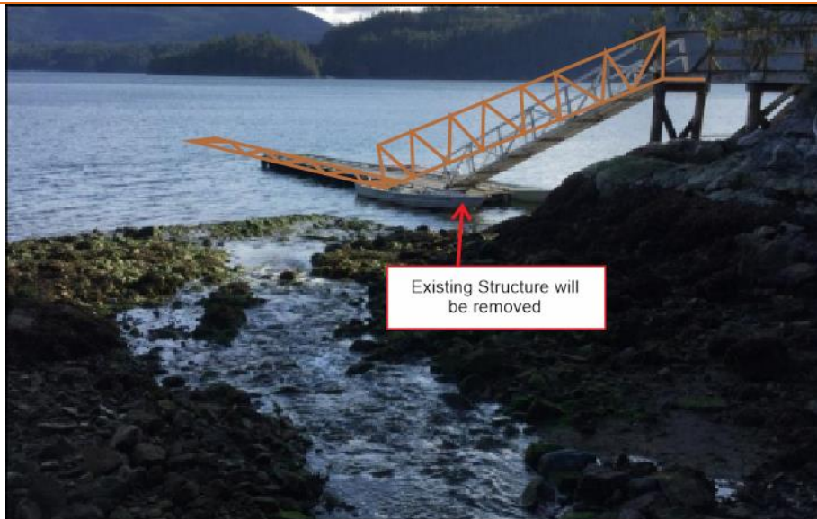
Figure 4: Schematic drawing showing the proposed dock. The height of the dock at lowest tide will be 0.5 m above the sea floor.
