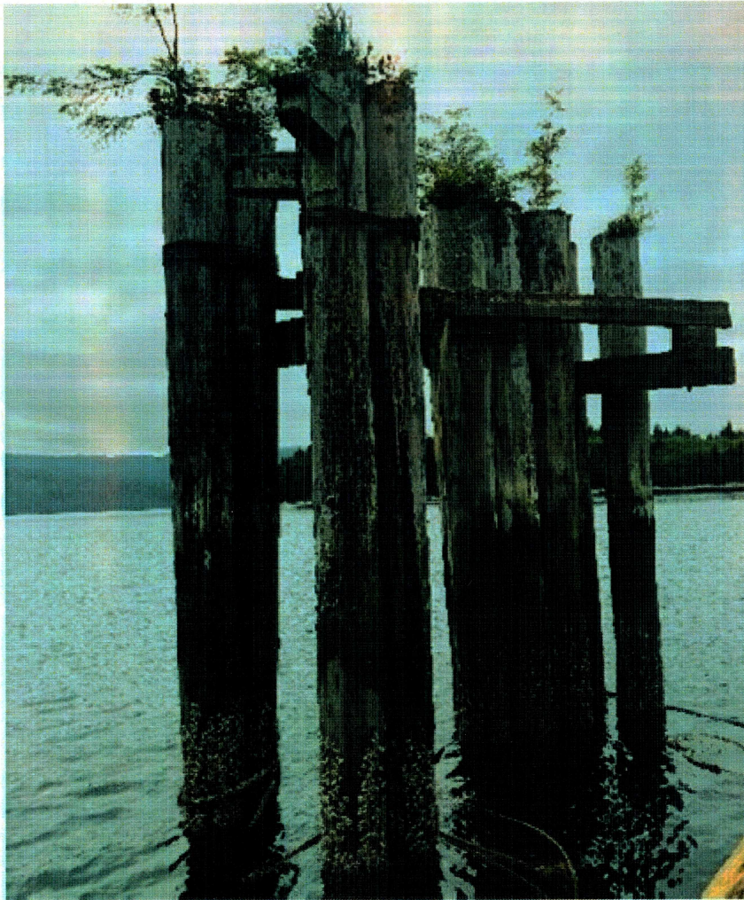
Photo 45 – South Mooring Dolphin
