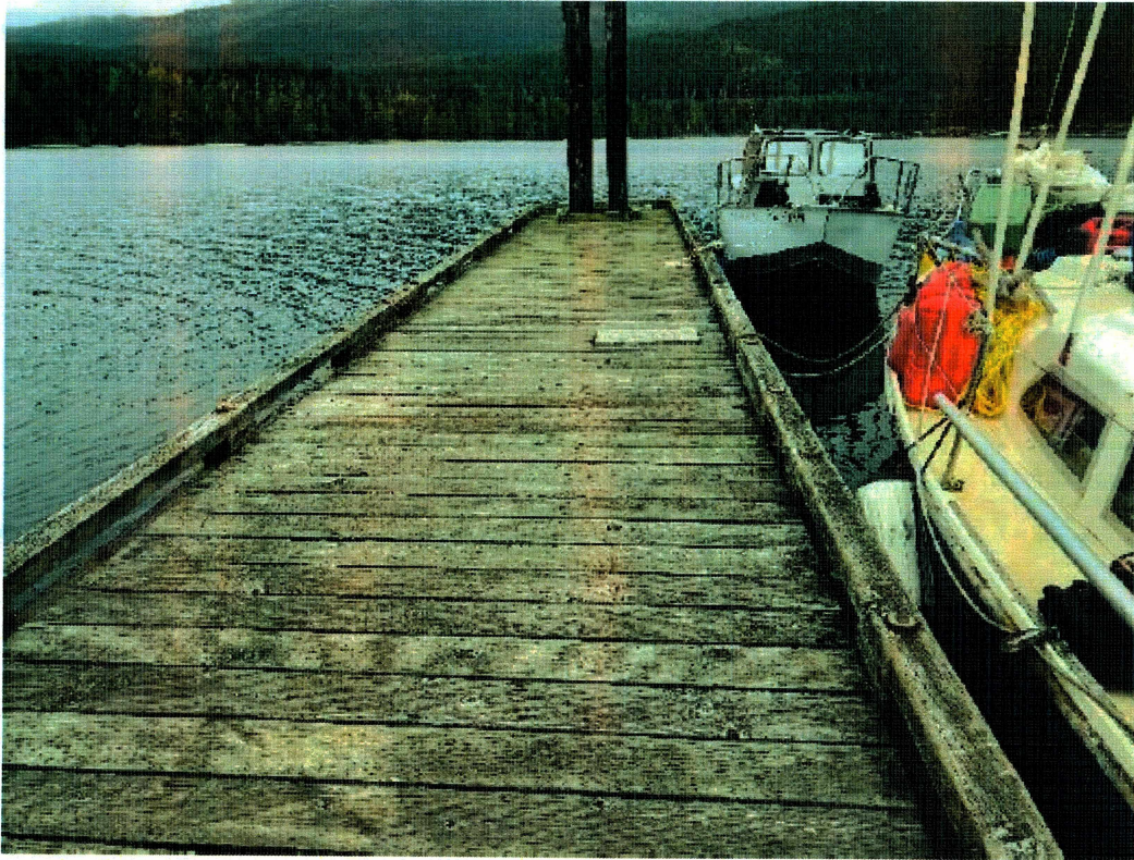
Photo 37 – General view of Float B
