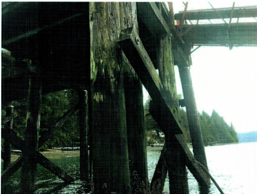
Photo 30 – Cross Bracing at Bent 15
