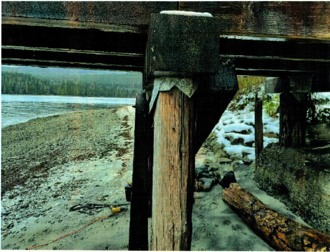
Photo 13 – Typical Timber Pile Cap End Grain
