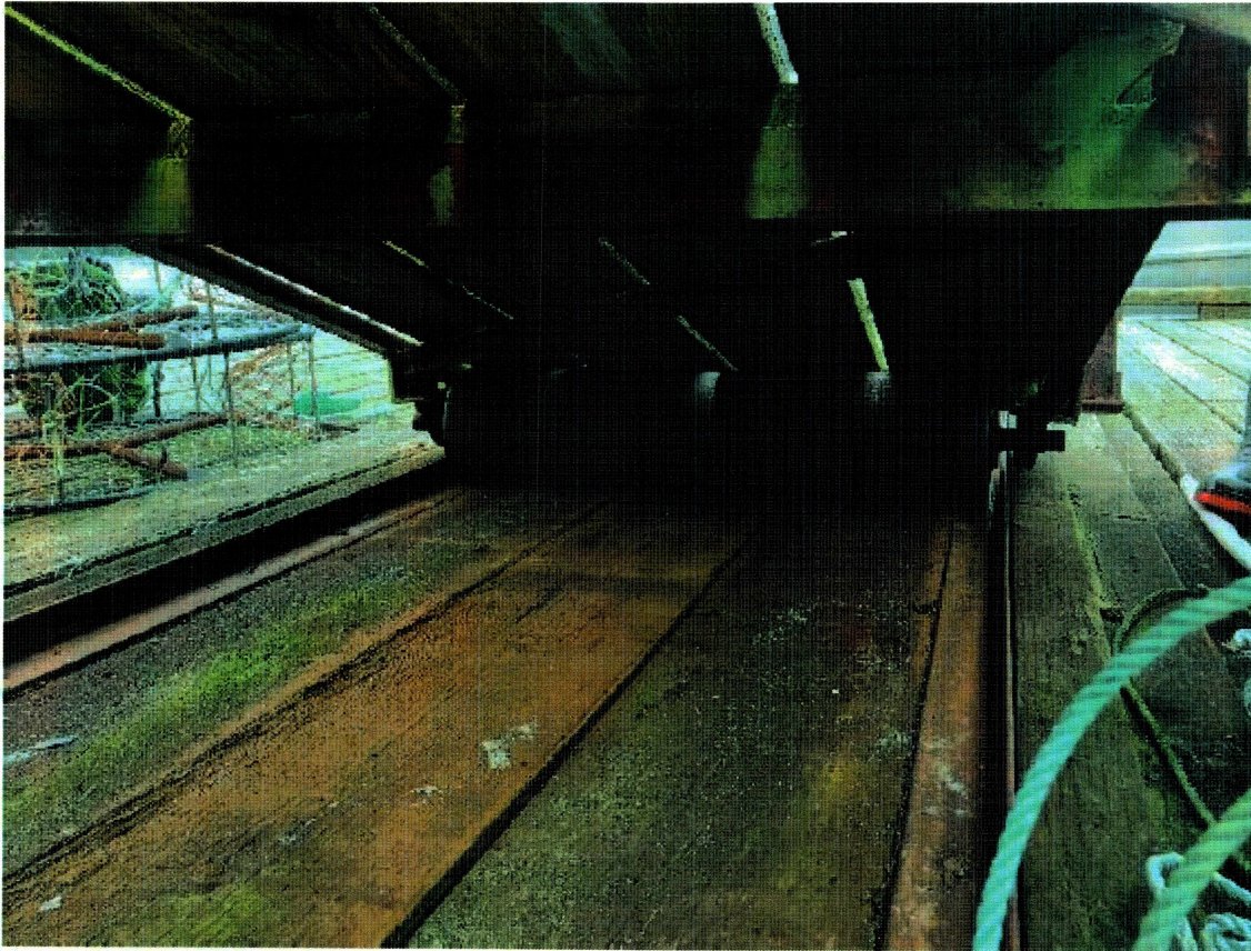
Photo 33 – Gangway Timber Slider Plate and Roller
