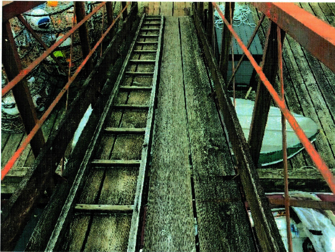
Photo 34 – Gangway Timber Deck Planks
