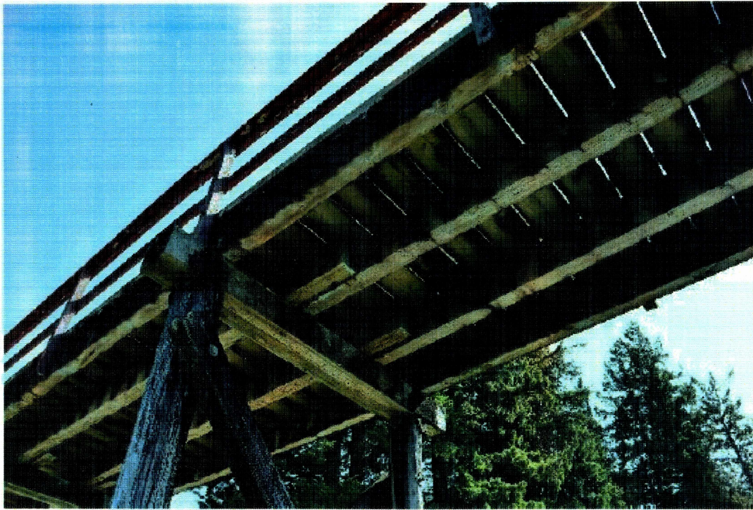
Photo 11 – Typical View of Timber Stringers
