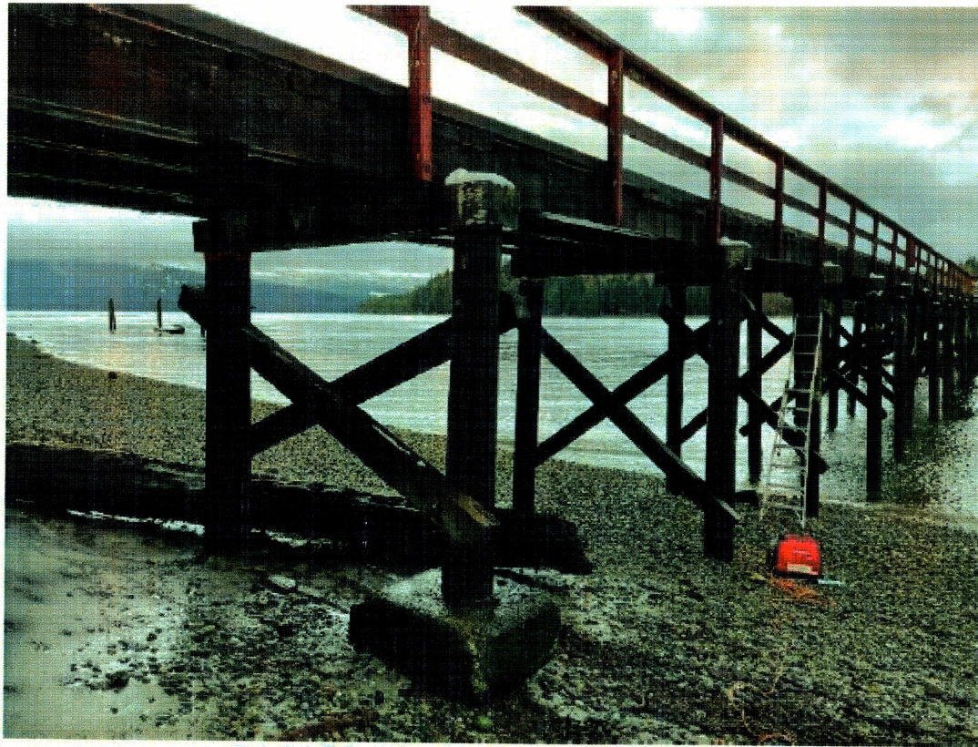
Photo 17 – Pile 4B concrete footing
