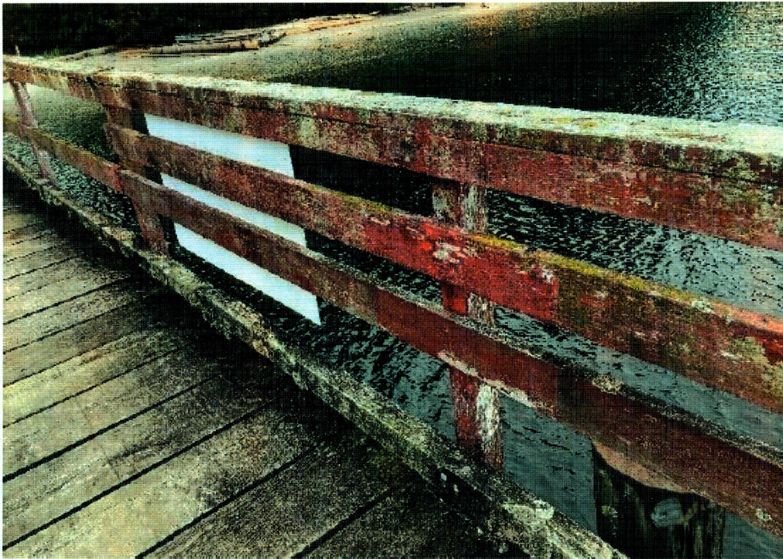
Photo 3 – Pier Structure Handrails
