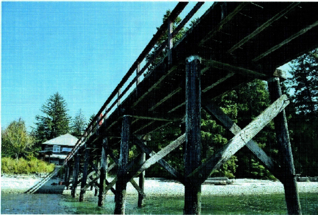
Photo 12 – General View of Timber Pile Cap Bents
