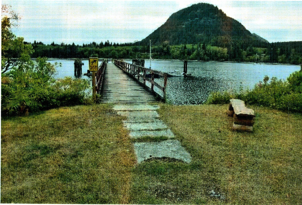
Photo 1 – Pier Approach Area
