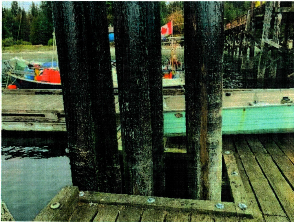
Photo 43 – Float A North Mooring Piles
