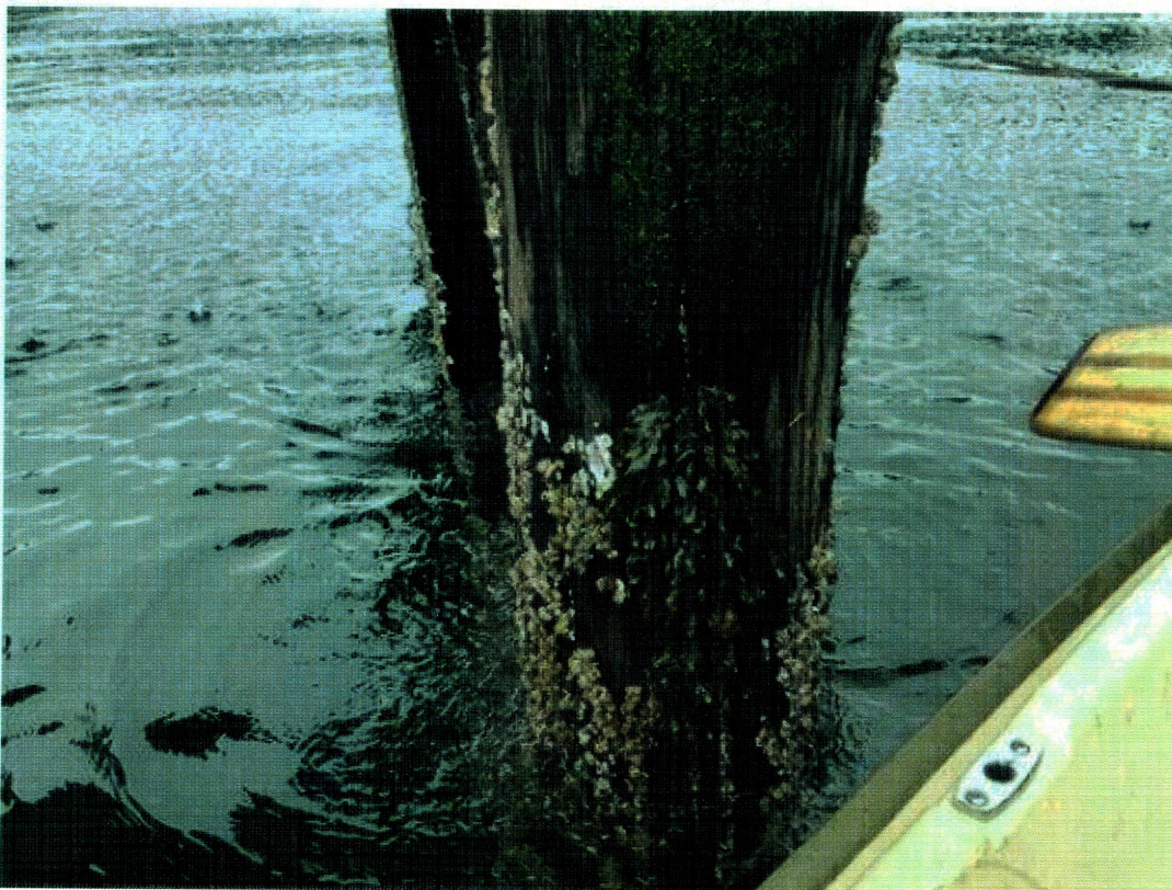
Photo 26 – Fender Pile 14A
