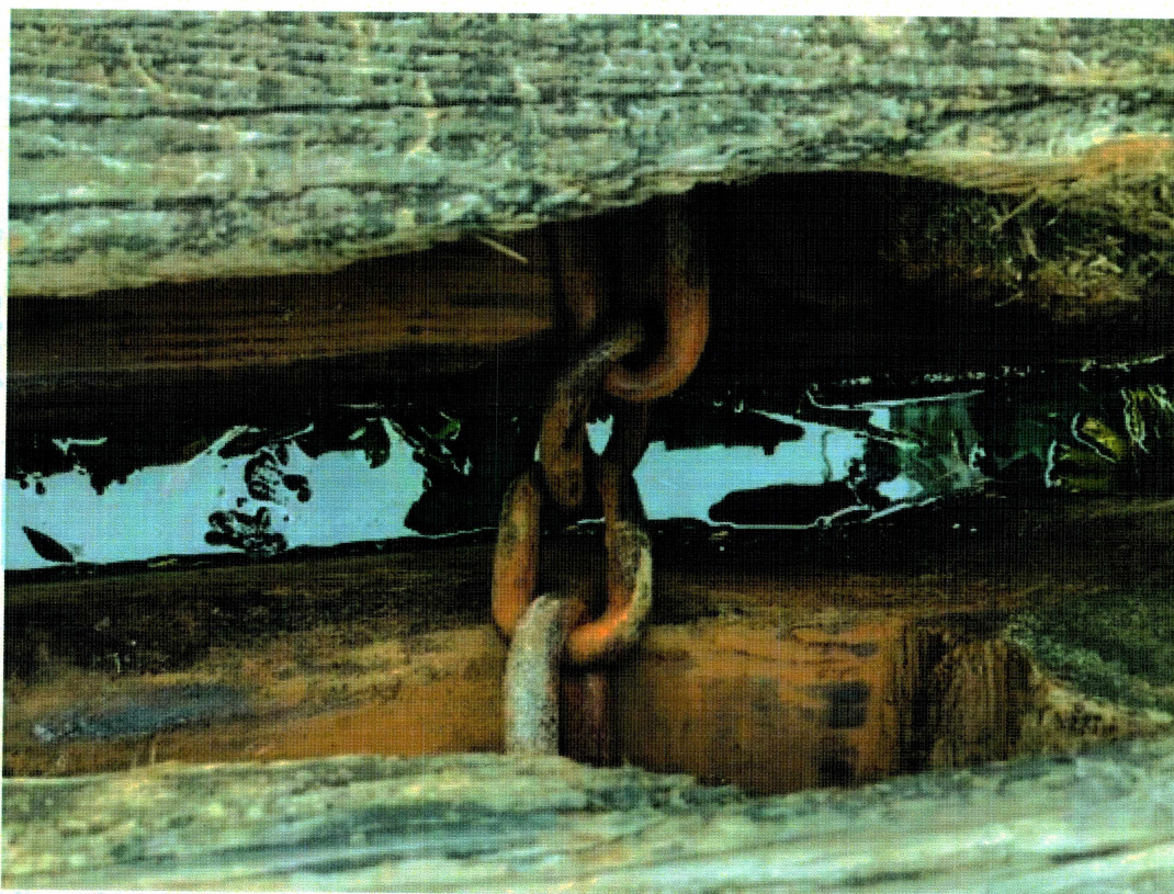
Photo 40 – Chain Connection to Float B
