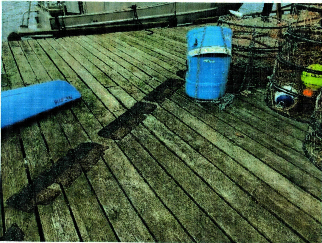
Photo 36 – General view of Float A
