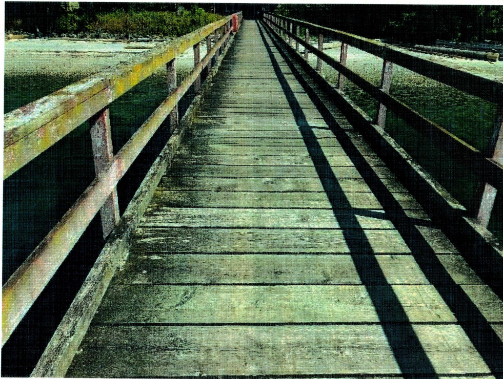
Photo 2 – Pier Structure Topsides
