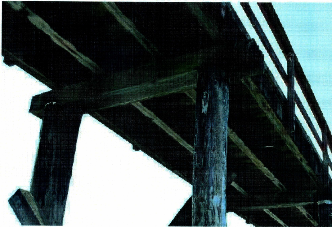
Photo 14 – Timber Pile Cap at Bent 12
