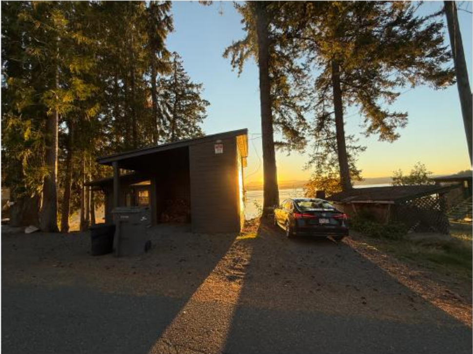
Photograph 5 - View of the front of the renovated structure and right side of the property.
