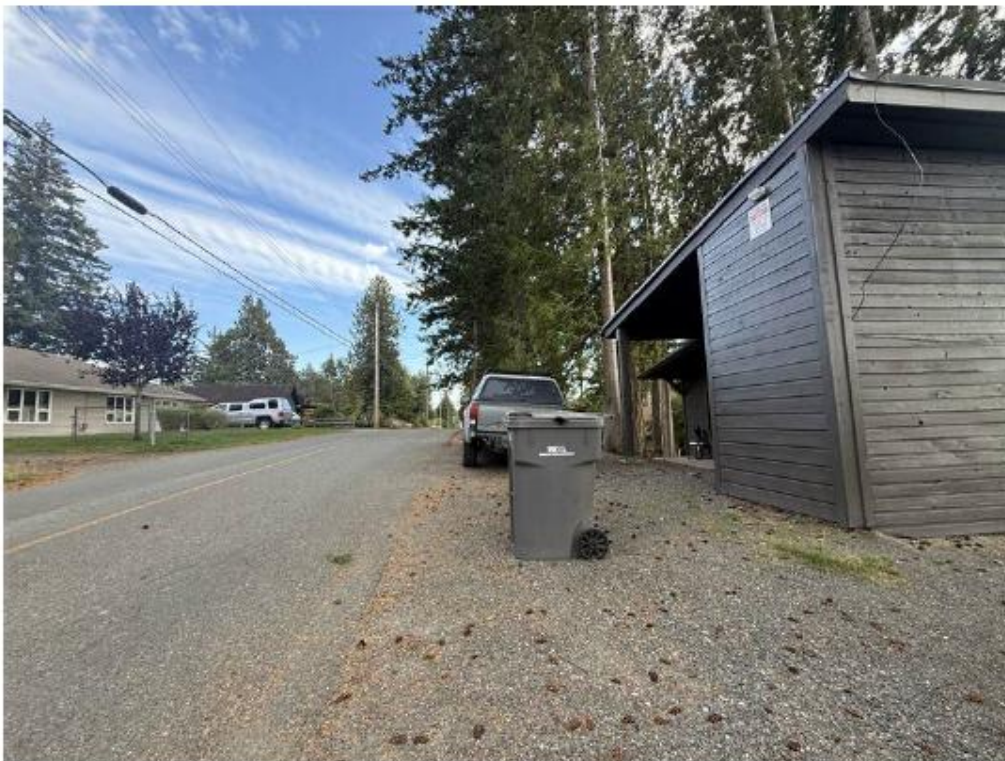
Photograph 1 – View of the front of 703 Green Road facing south.
