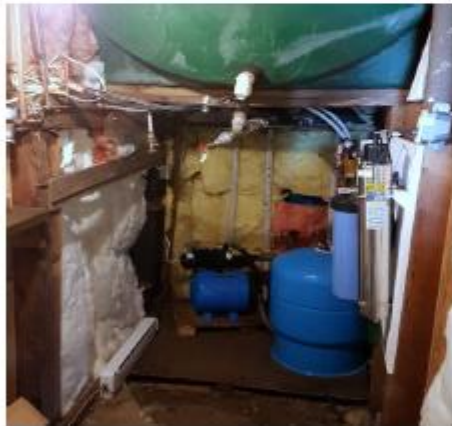
View under 1000 gal storage tank
