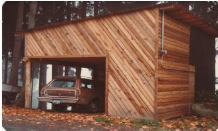
Completed Water Storage Building 1979
