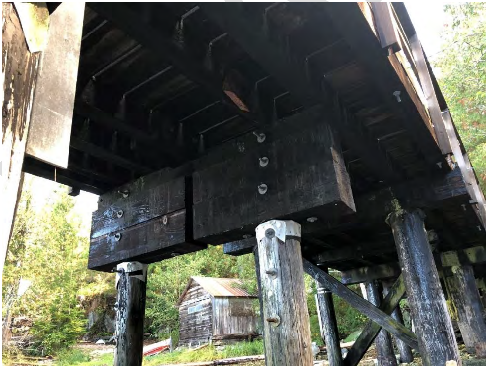
Photo 14 - Pile cap at Bent 6 and corbels
