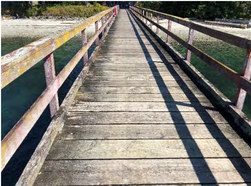
Photo 2 – Pier Structure Topsides
