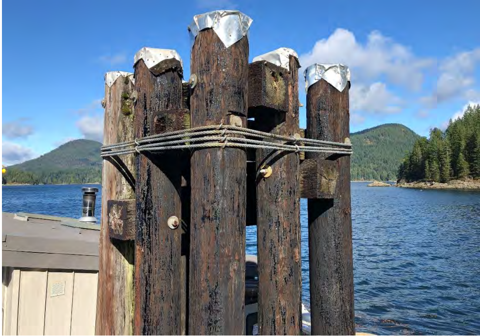
Photo 51 - East end Mooring Piles
