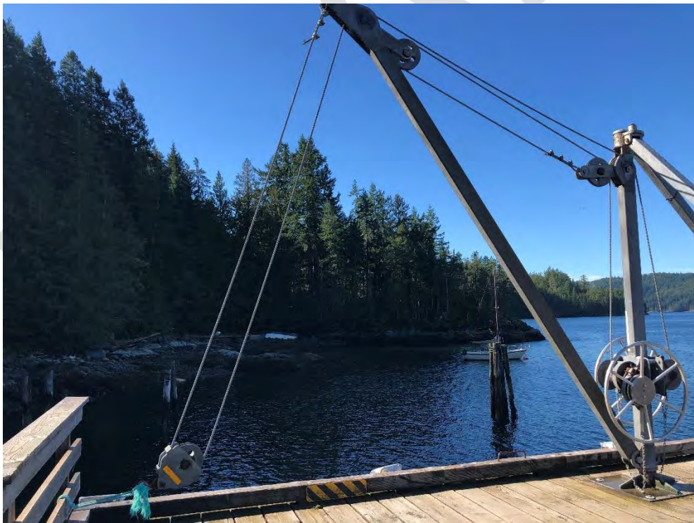
Photo 36 - Derrick Loading Crane
