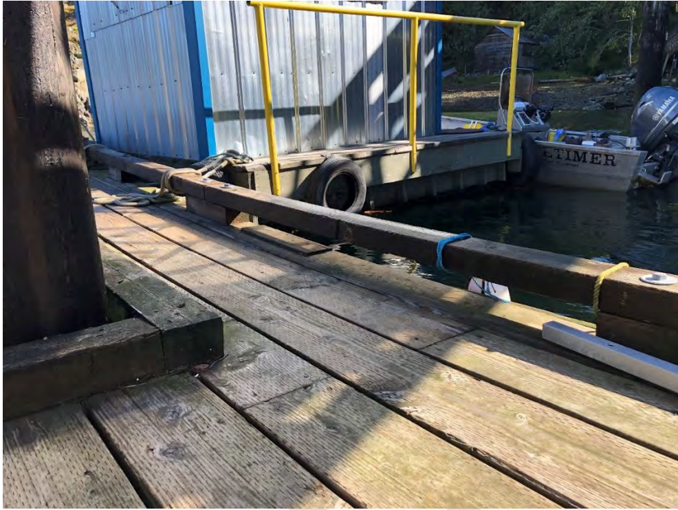
Photo 47 - Flotation loss at centre of the Main Float on the east end
