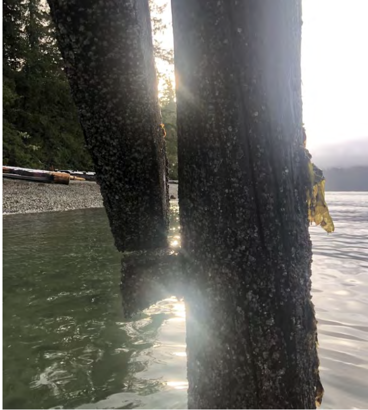
Photo 29 – Cross Bracing at Bent 8
