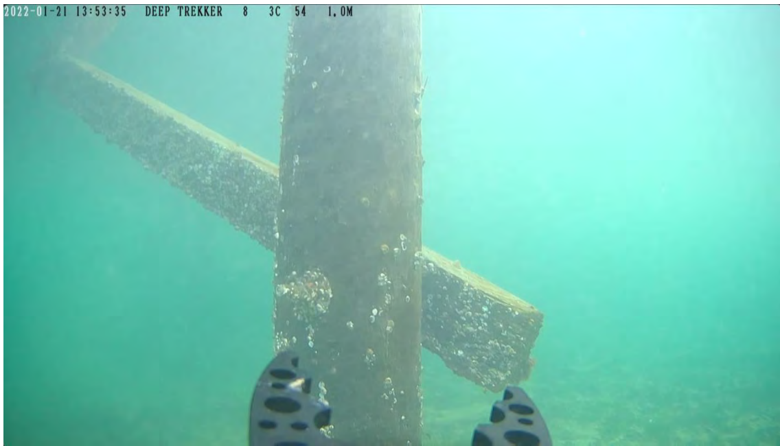
Photo 20 - Typical condition of underwater cross-bracing
