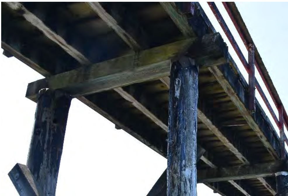
Photo 14 – Timber Pile Cap at Bent 12
