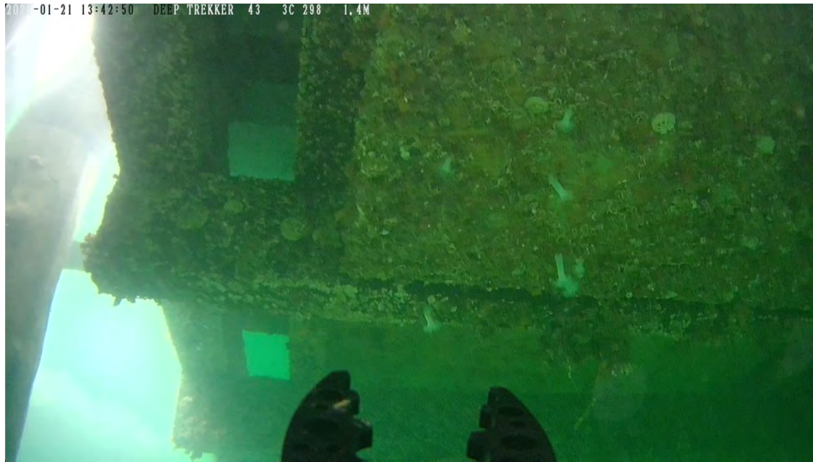
Photo 35 - Typical condition under the south end of the float
