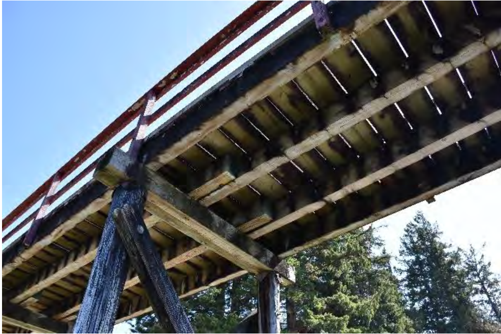
Photo 11 – Typical View of Timber Stringers
