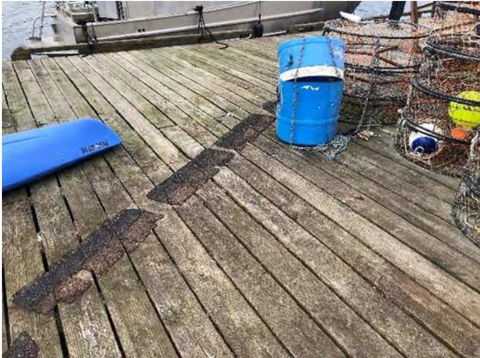
Photo 36 – General view of Float A
