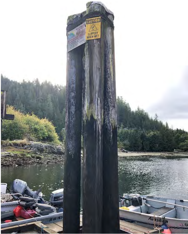
Photo 27 - South Mooring Piles
