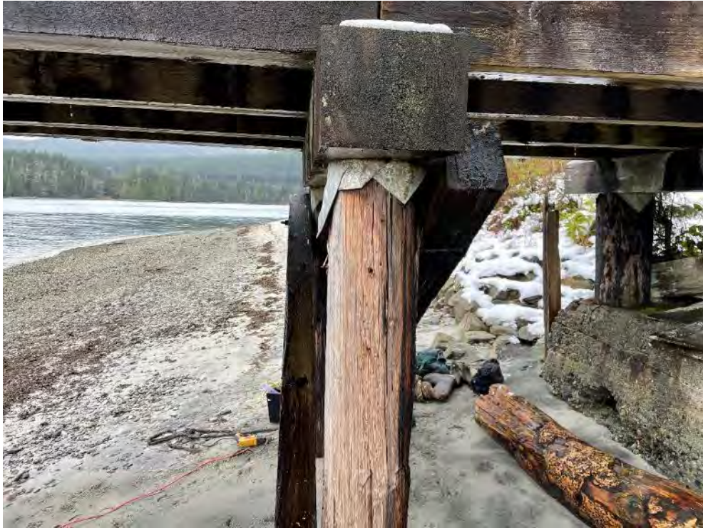
Photo 13 – Typical Timber Pile Cap End Grain
