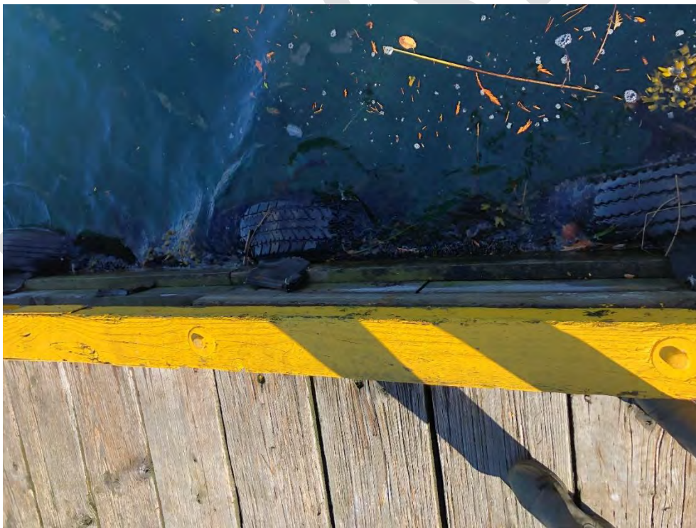
Photo 60 - Typical condition of the timber bull rails, fascia board and rubber tire fendering on the Seaplane Float
