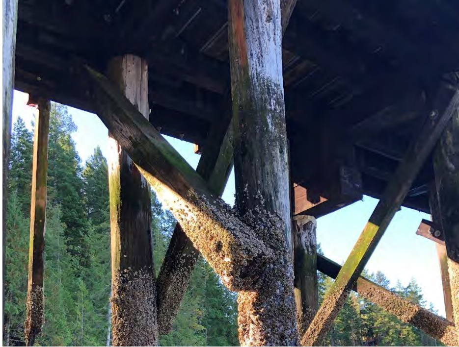
Photo 31 - General condition of the Cross Bracing
