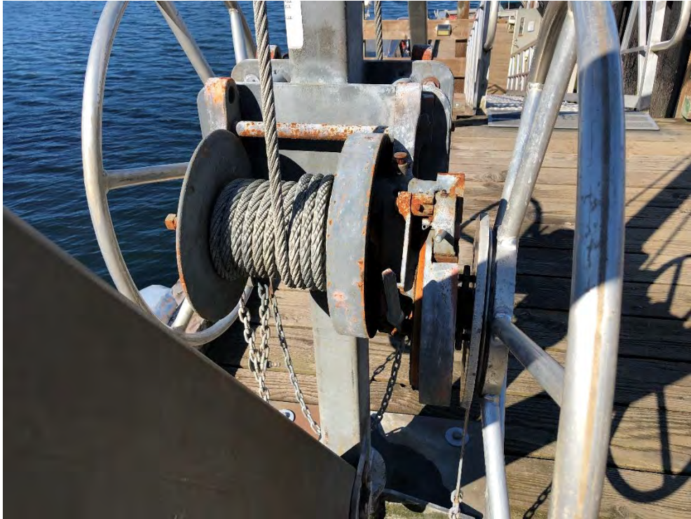
Photo 37 - Derrick Loading Crane
