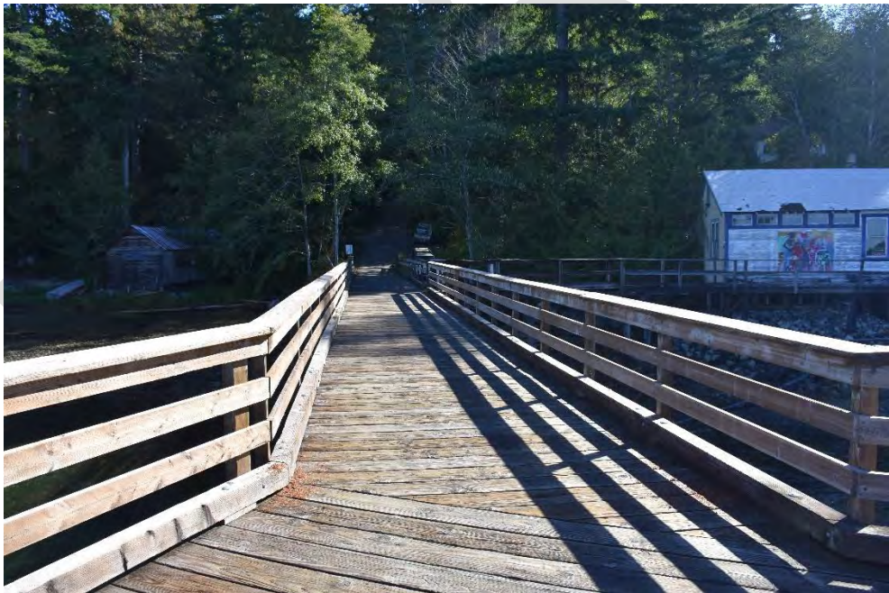
Photo 4 - Wharf Structure Handrails
