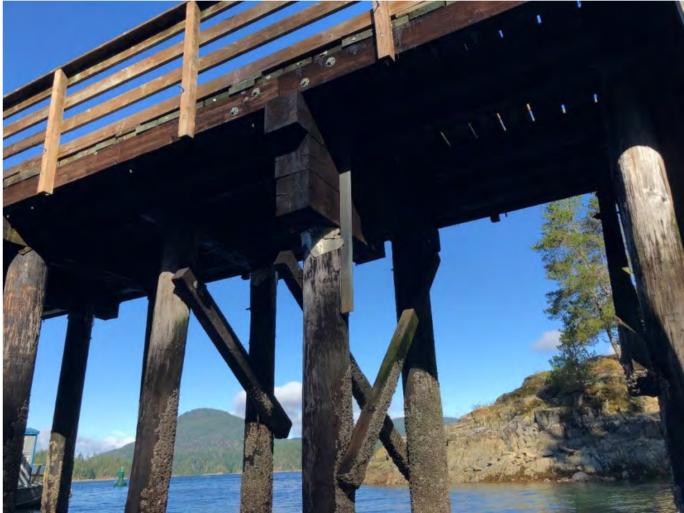
Photo 21 - Pile cap at Bent 13 with corbels
