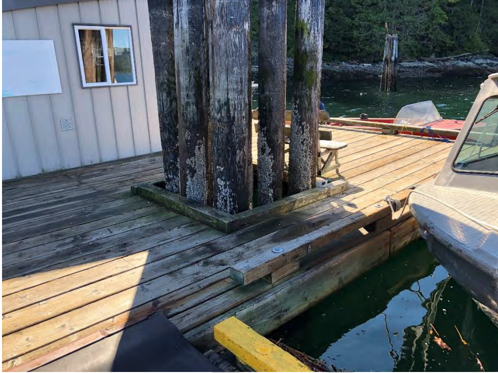
Photo 53 - West end Mooring Piles
