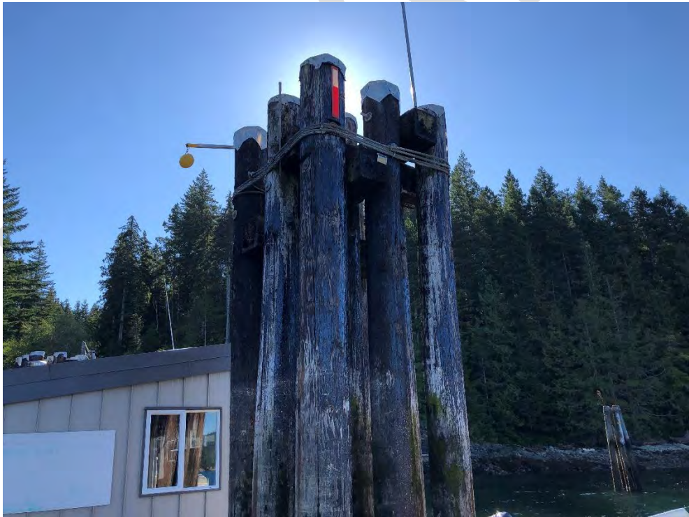
Photo 54 - West end Mooring Piles
