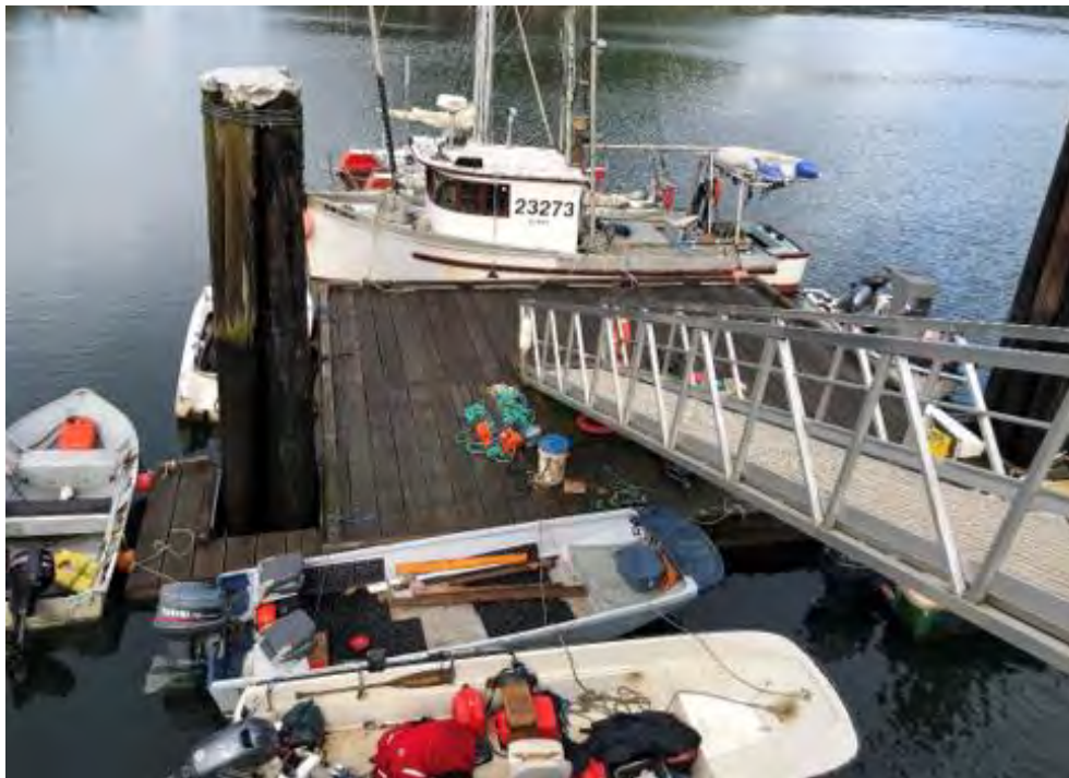
Photo 24 - General View of the float
