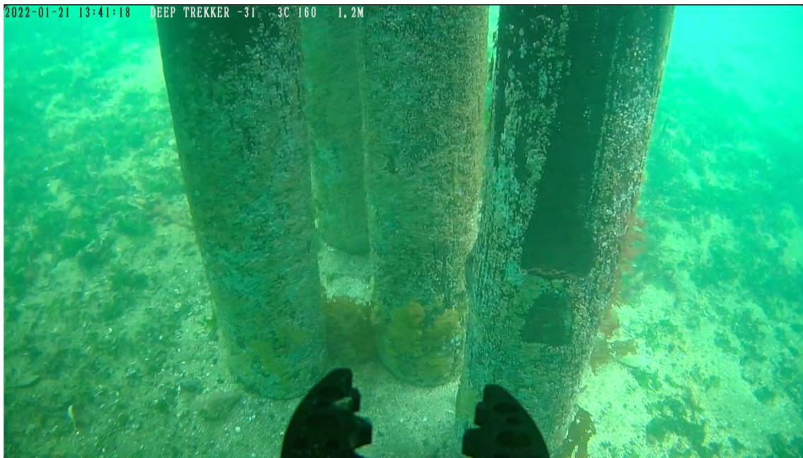
Photo 30 - South Mooring Piles
