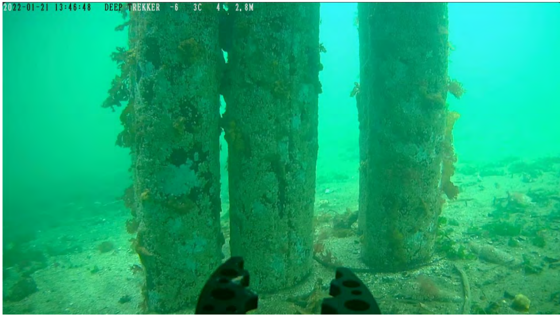
Photo 31 - North Mooring Piles
