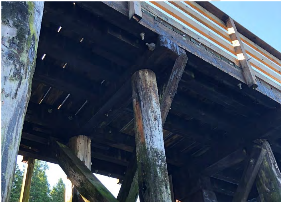
Photo 20 - Pile cap at Bent 12
