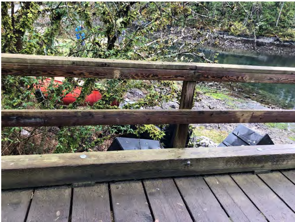
Photo 4 - General View of the Handrails
