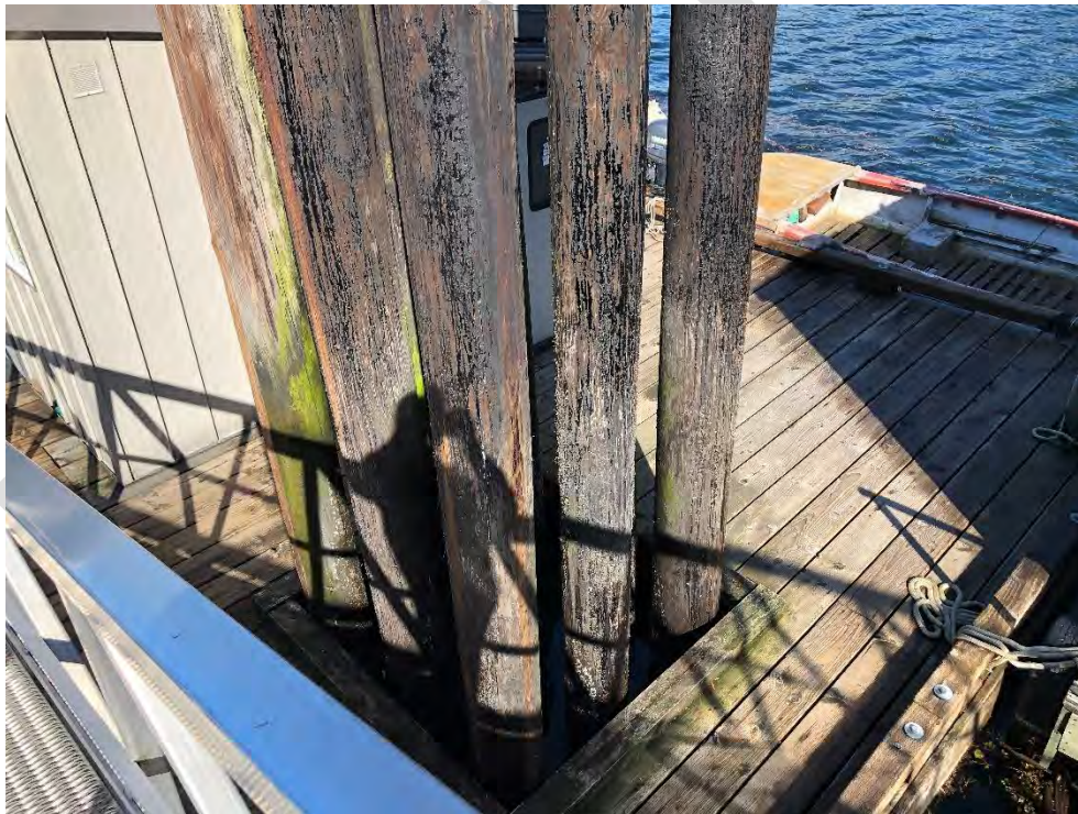
Photo 50 - East end Mooring Piles
