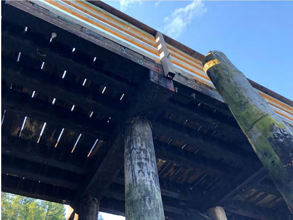
Photo 19 - Pile cap at Bent 11
