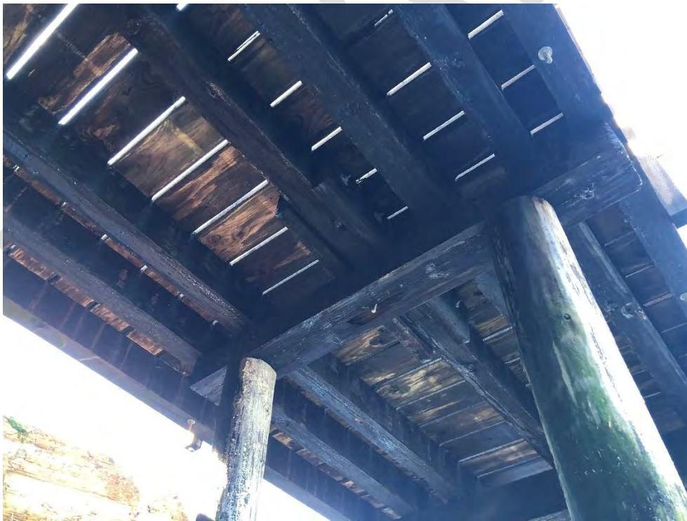
Photo 8 - Typical View of Timber Stringers
