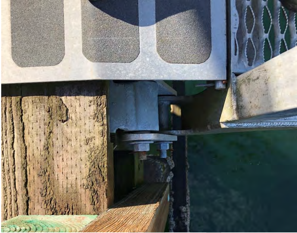
Photo 41 - Gangway Upper Hinge Connection
