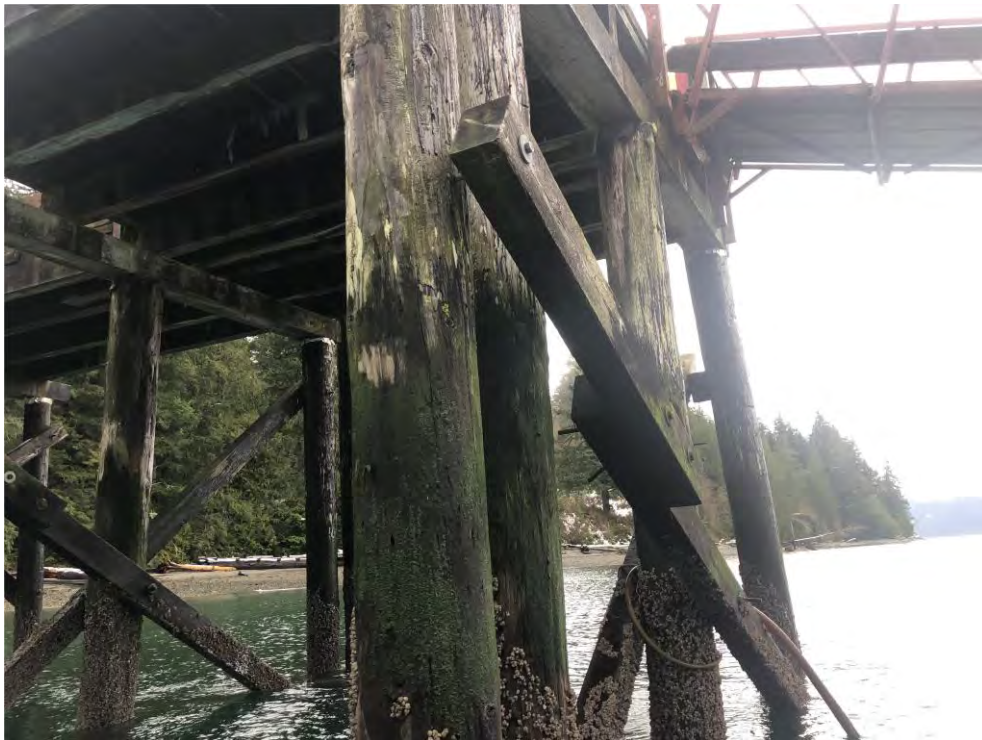
Photo 30 – Cross Bracing at Bent 15
