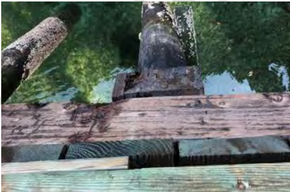
Photo 22 - Pile cap at Bent 14
