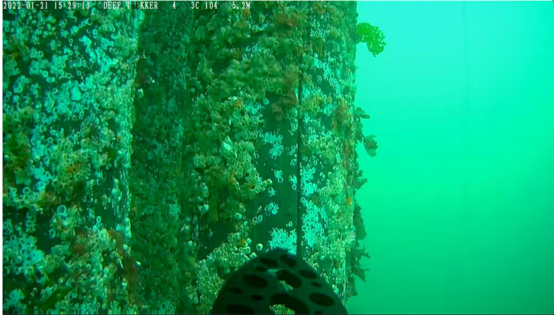
Photo 57 - West end Mooring Piles
