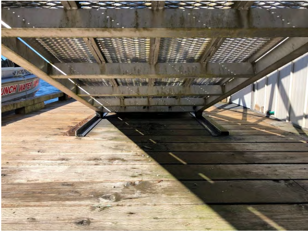
Photo 40 - Gangway slider plate and rollers
