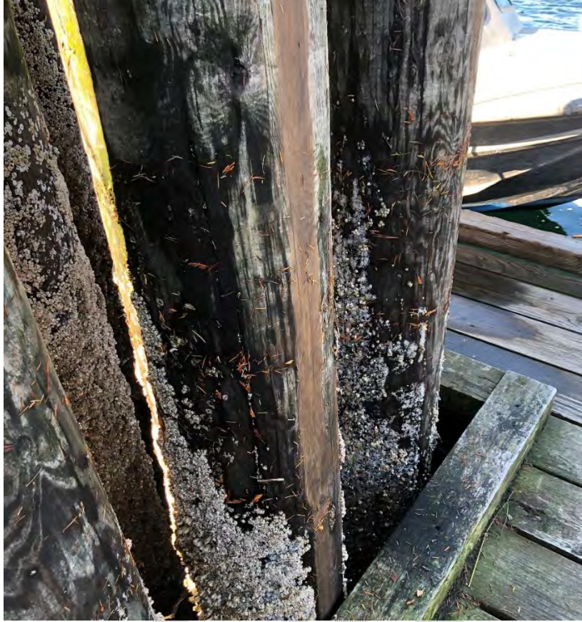
Photo 55 - West end Mooring Piles – up to 10% CSL
