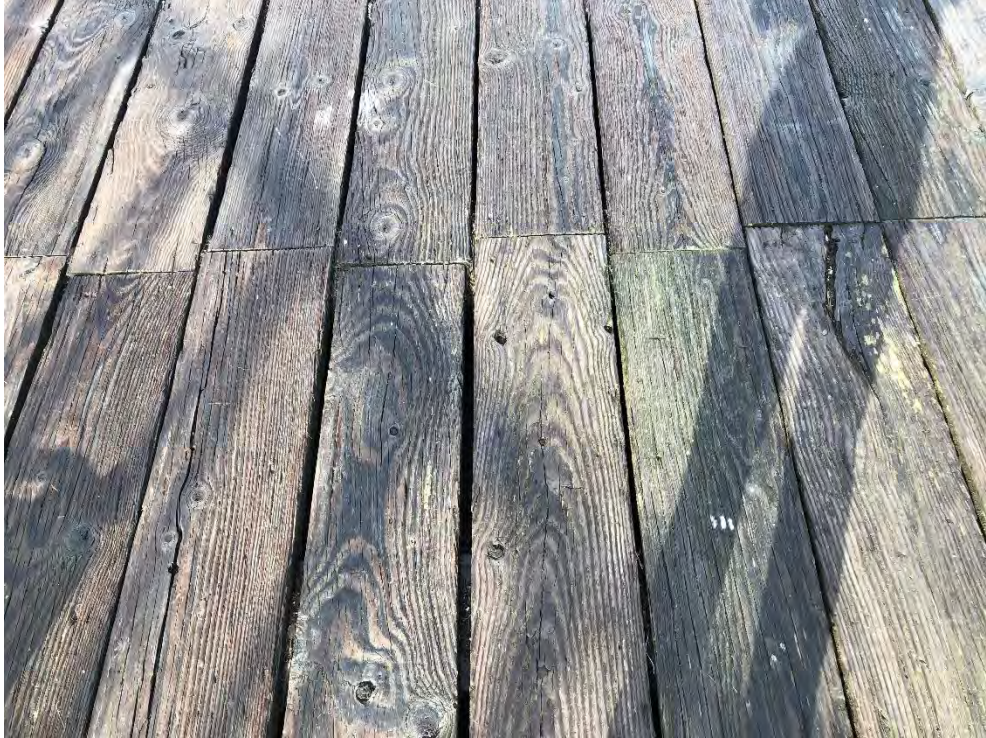
Photo 25 - Typical condition of the timber decking
