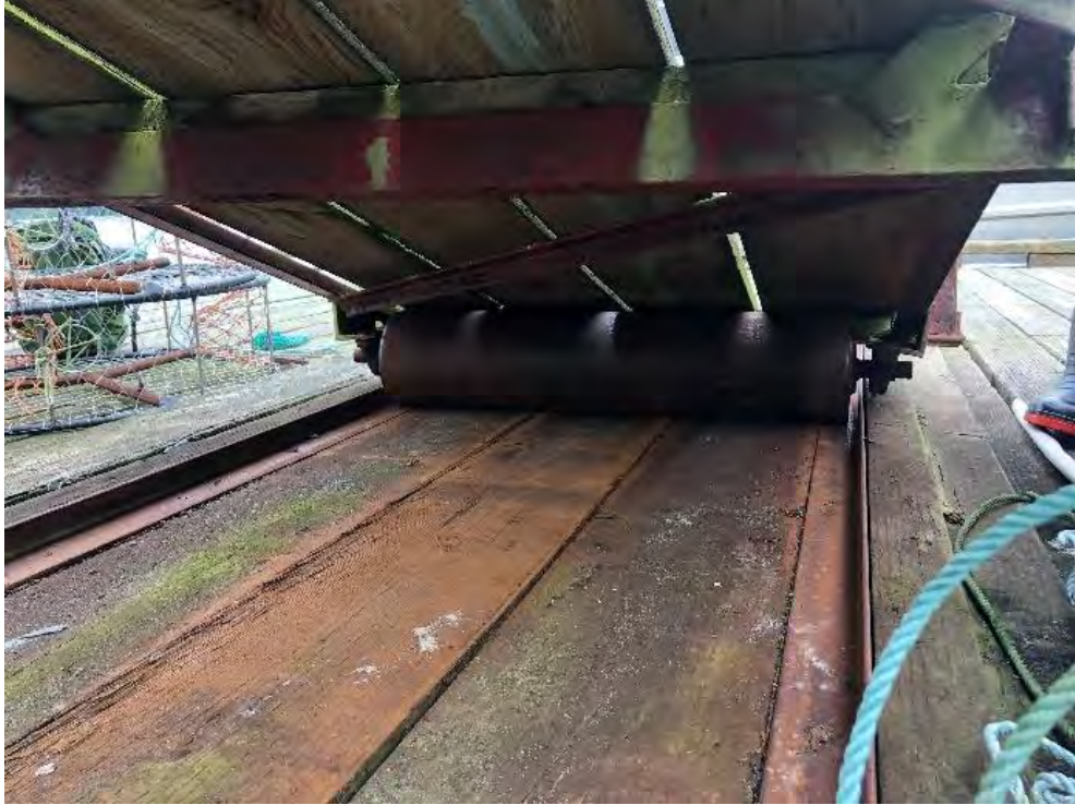
Photo 33 – Gangway Timber Slider Plate and Roller
