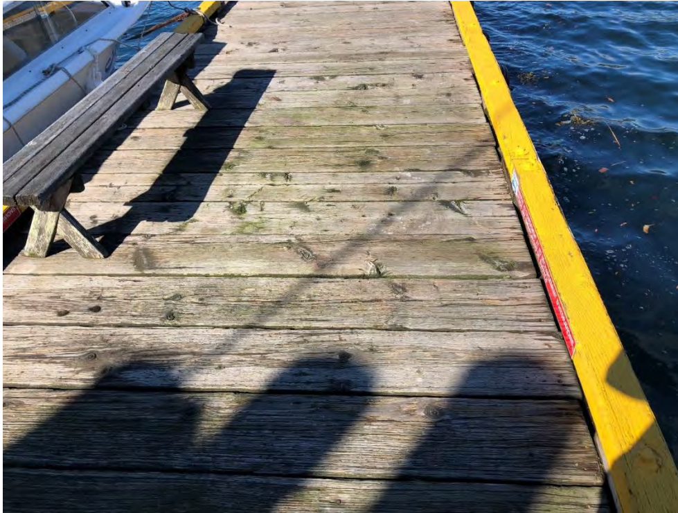
Photo 59 - Typical condition of the Seaplane Float deck
