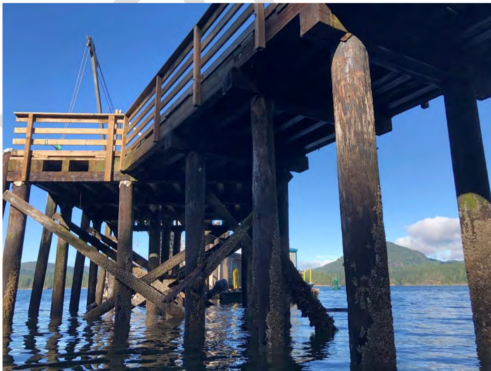
Photo 34 - Log resting on the Cross Bracing
