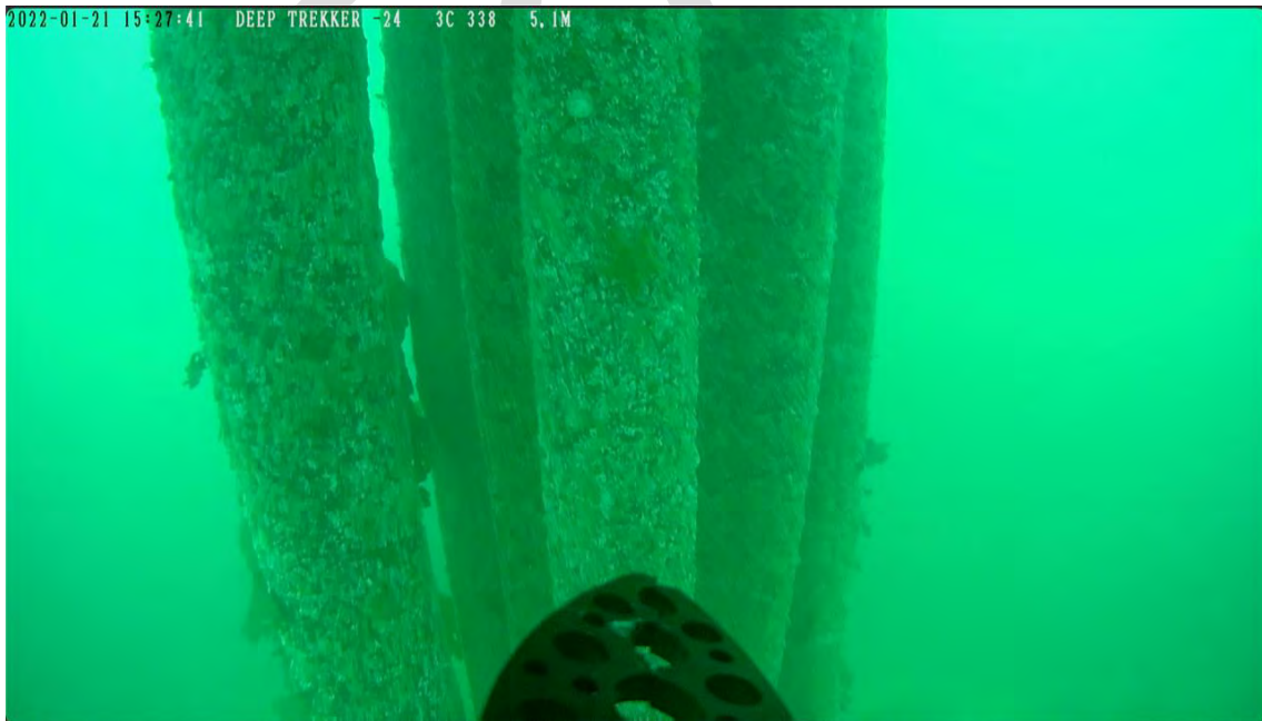
Photo 56 - West end Mooring Piles
