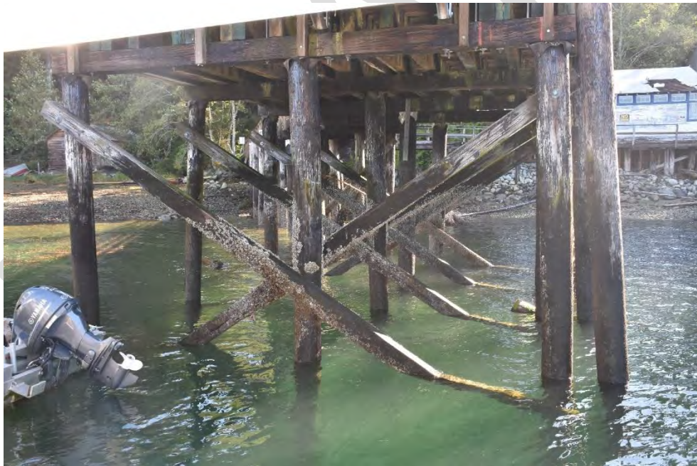
Photo 32 - General view of Cross Bracing
