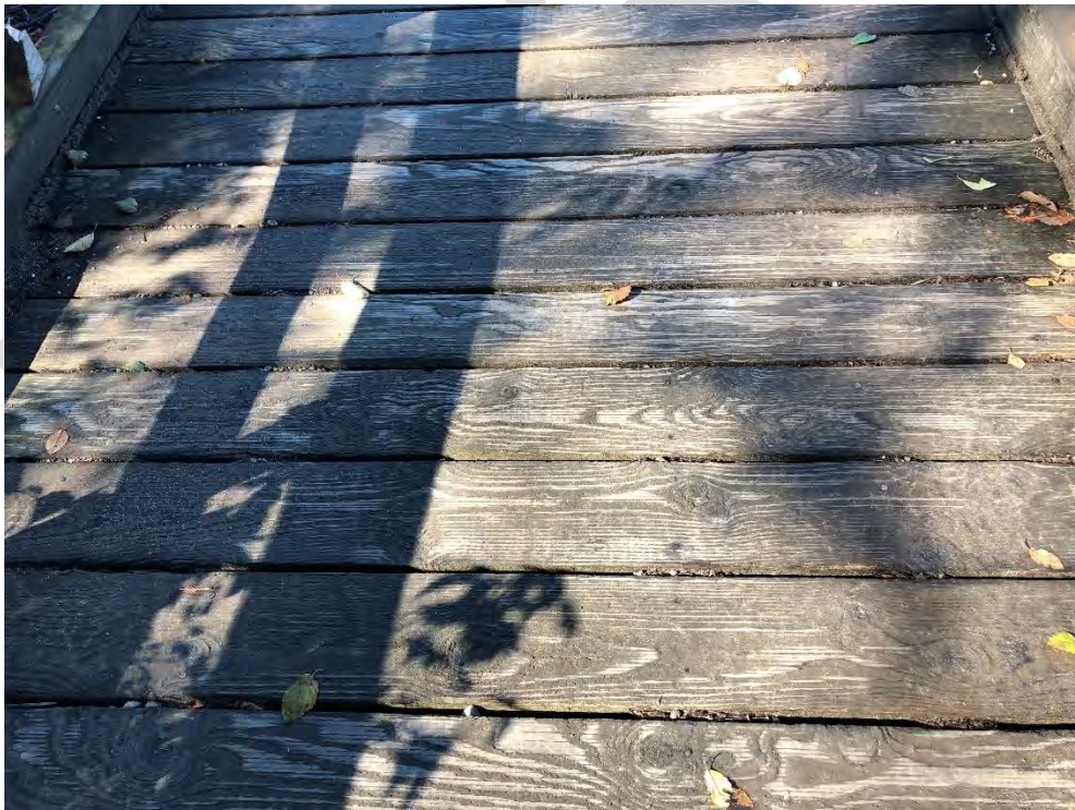
Photo 6 - Wharf Structure Decking
