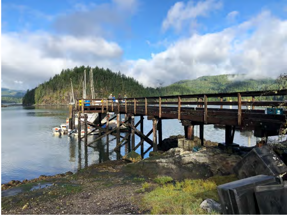
Photo 1 - General View facing West
