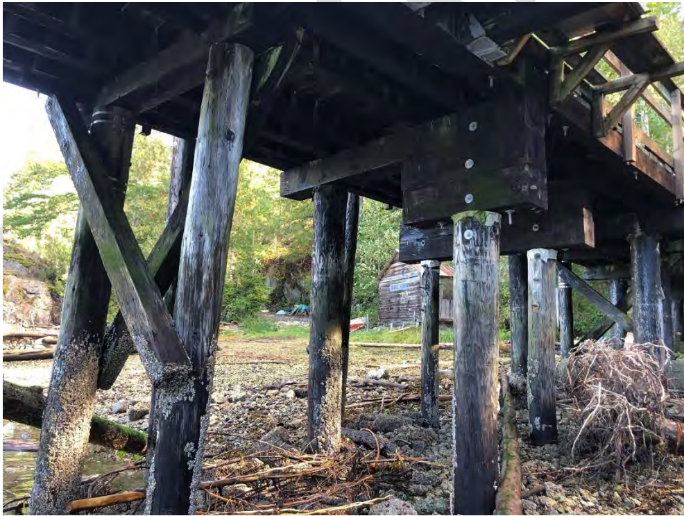
Photo 16 - Pile cap at Bent 7 and corbels
