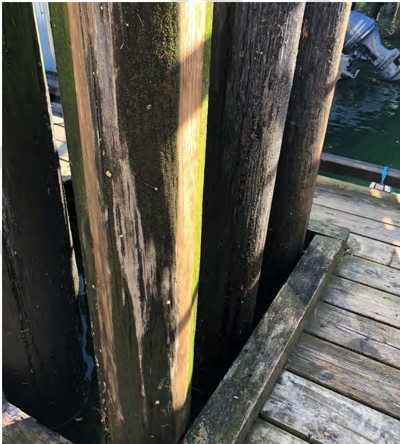
Photo 52 - East end Mooring Piles
