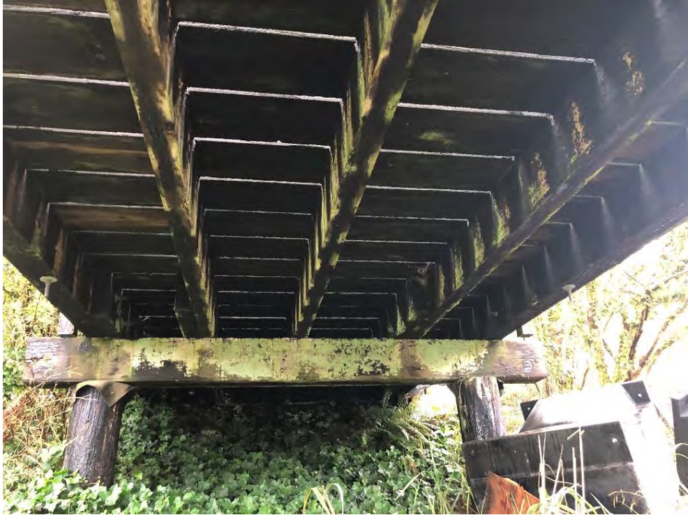
Photo 5 - General view of the Stringers
