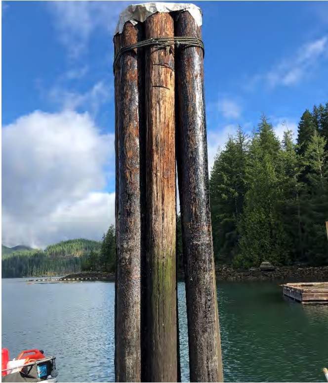
Photo 28 - North Mooring Piles
