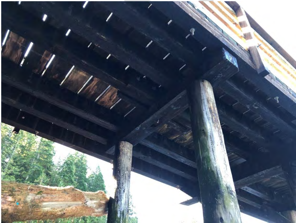
Photo 18 - Pile cap at Bent 10
