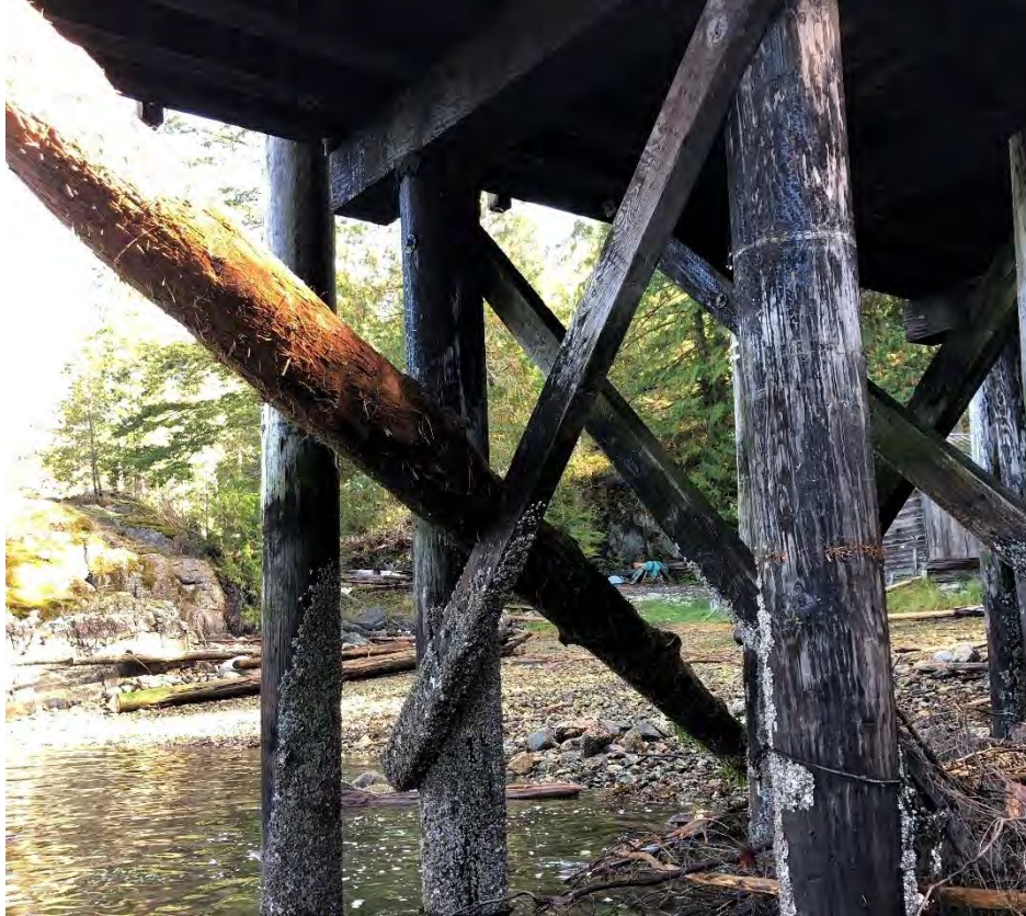
Photo 33 - Log resting on the Cross Bracing
