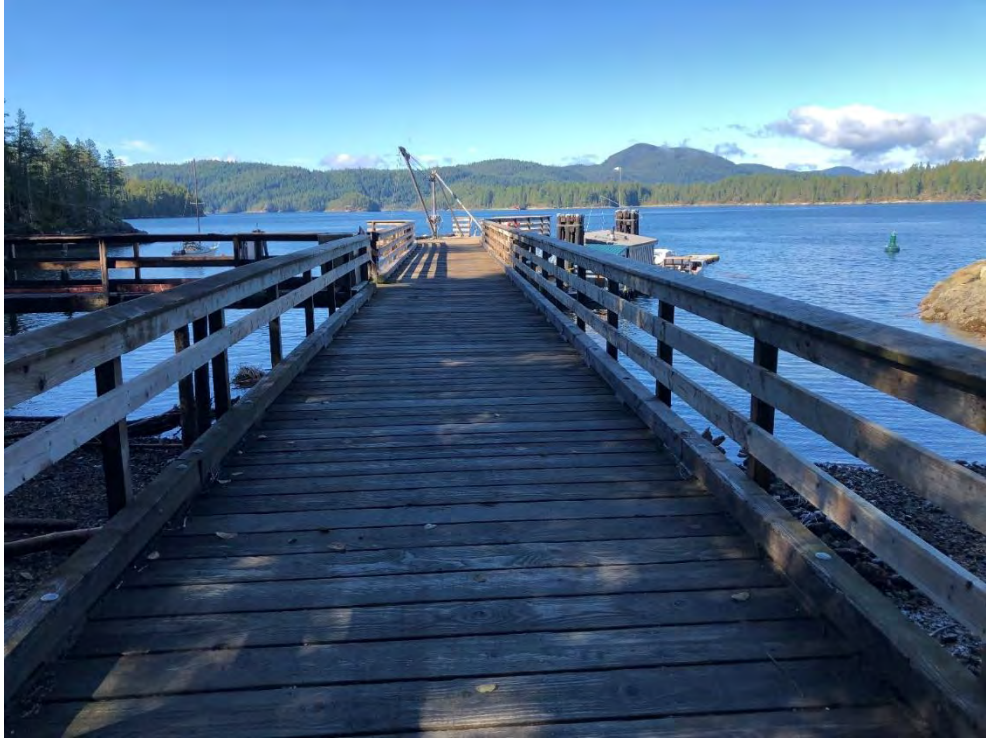
Photo 3 - Wharf Structure Topsides
