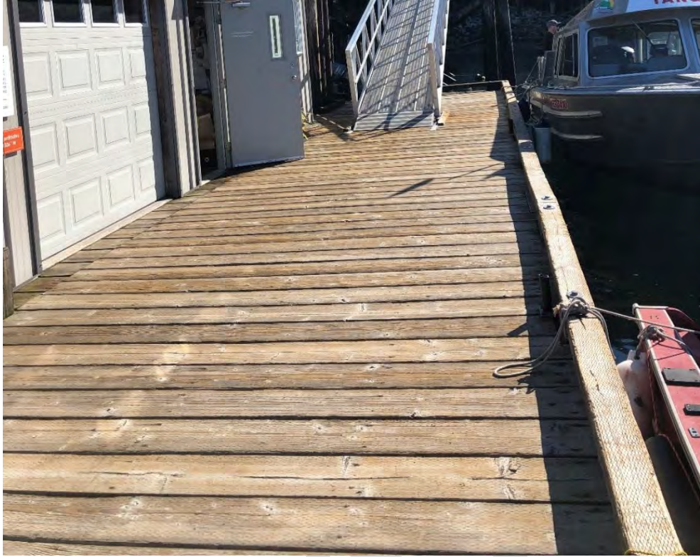
Photo 43 - Typical condition of the Main Float deck
