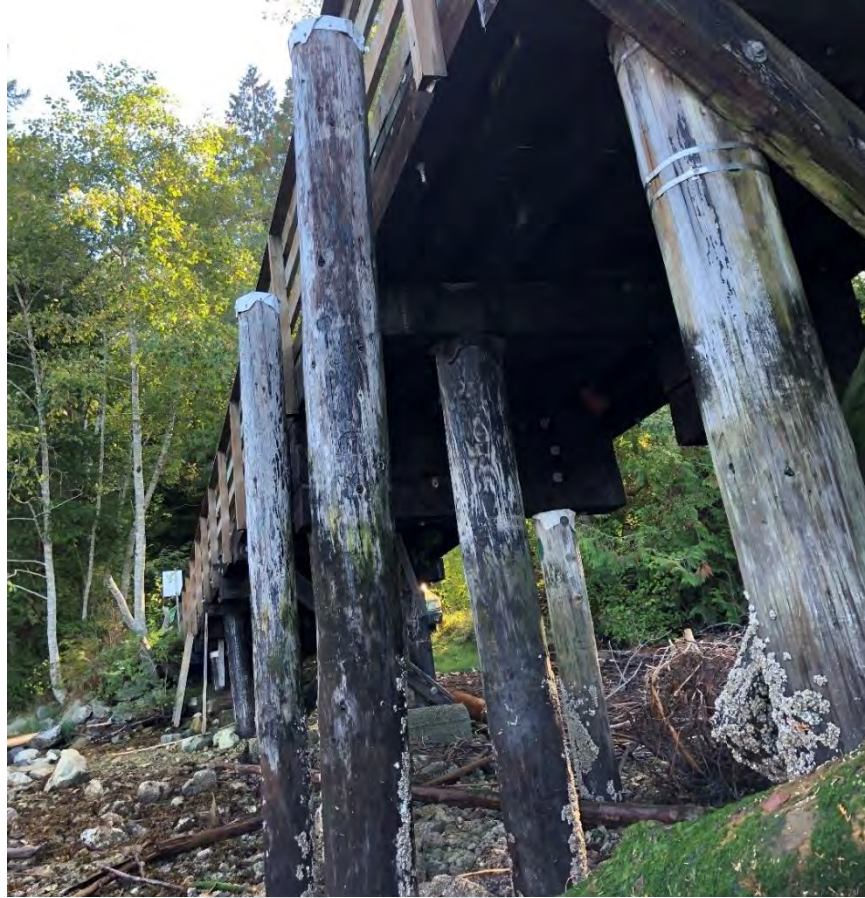
Photo 29 - North end fender piles
