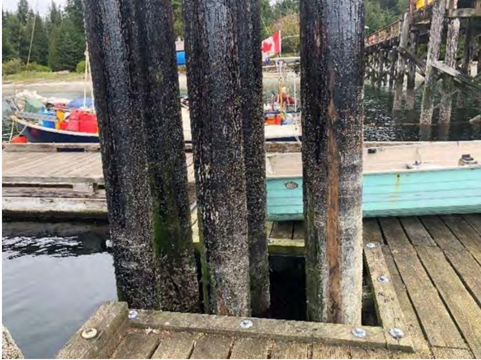
Photo 43 – Float A North Mooring Piles
