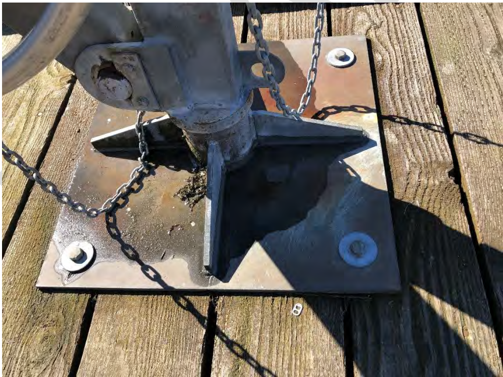
Photo 38 - Derrick Loading Crane
