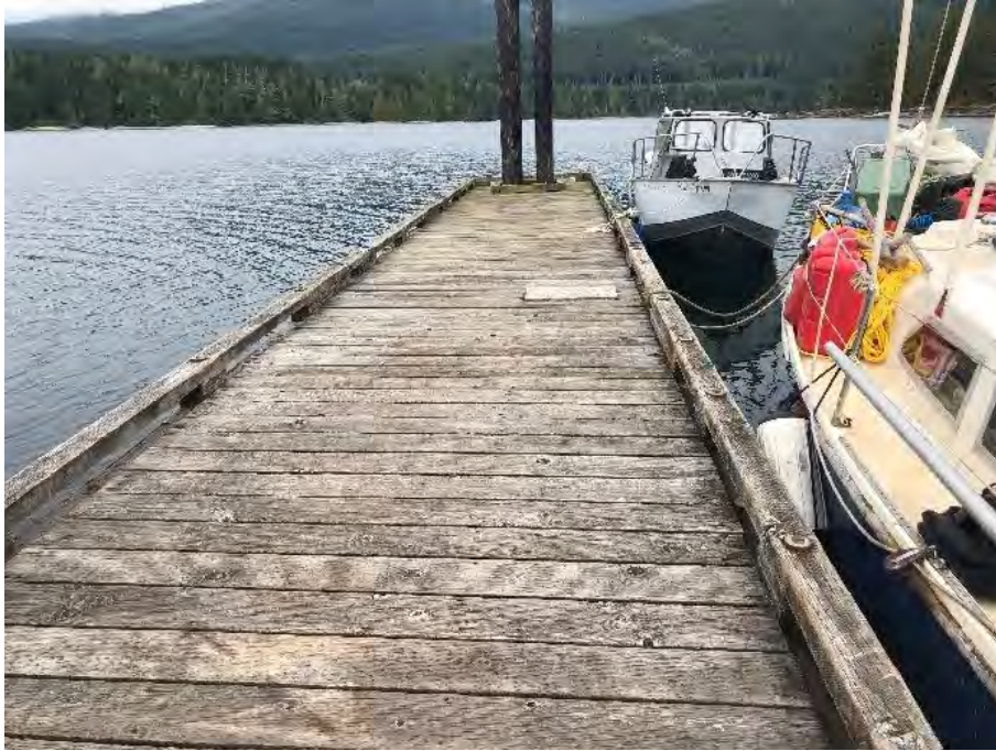
Photo 37 – General view of Float B
