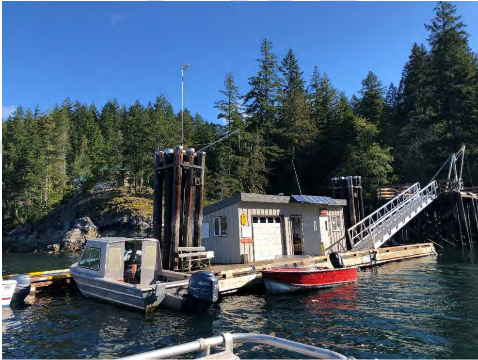
Photo 42 - General View of the Main Float
