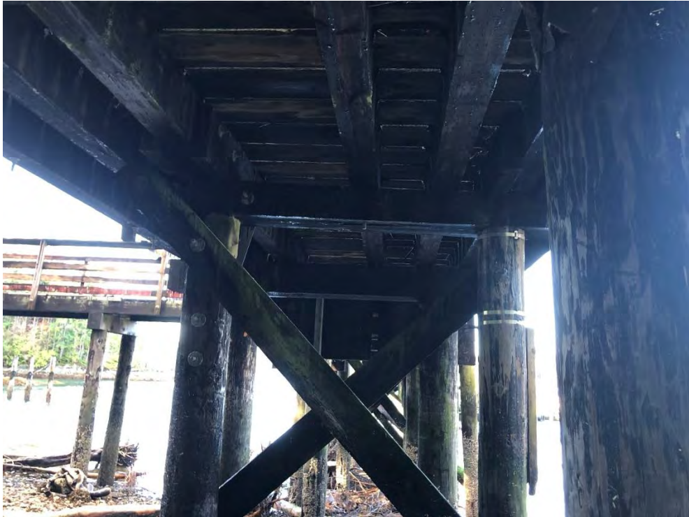
Photo 13 - Pile cap at Bent 4
