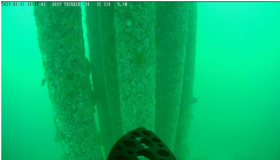
Photo 56 - West end Mooring Piles
