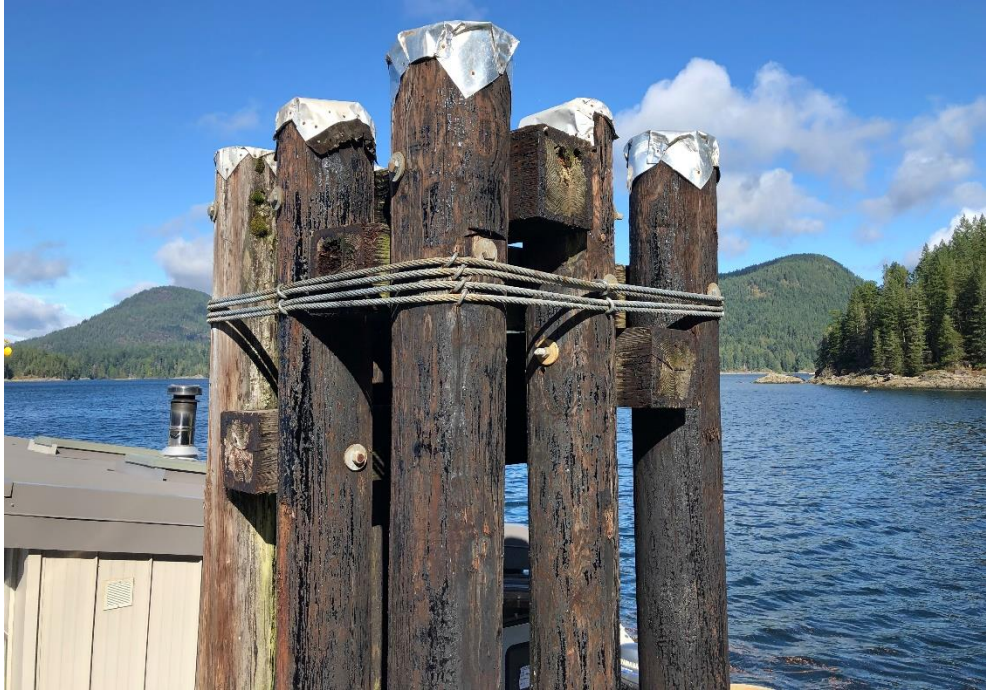
Photo 51 - East end Mooring Piles
