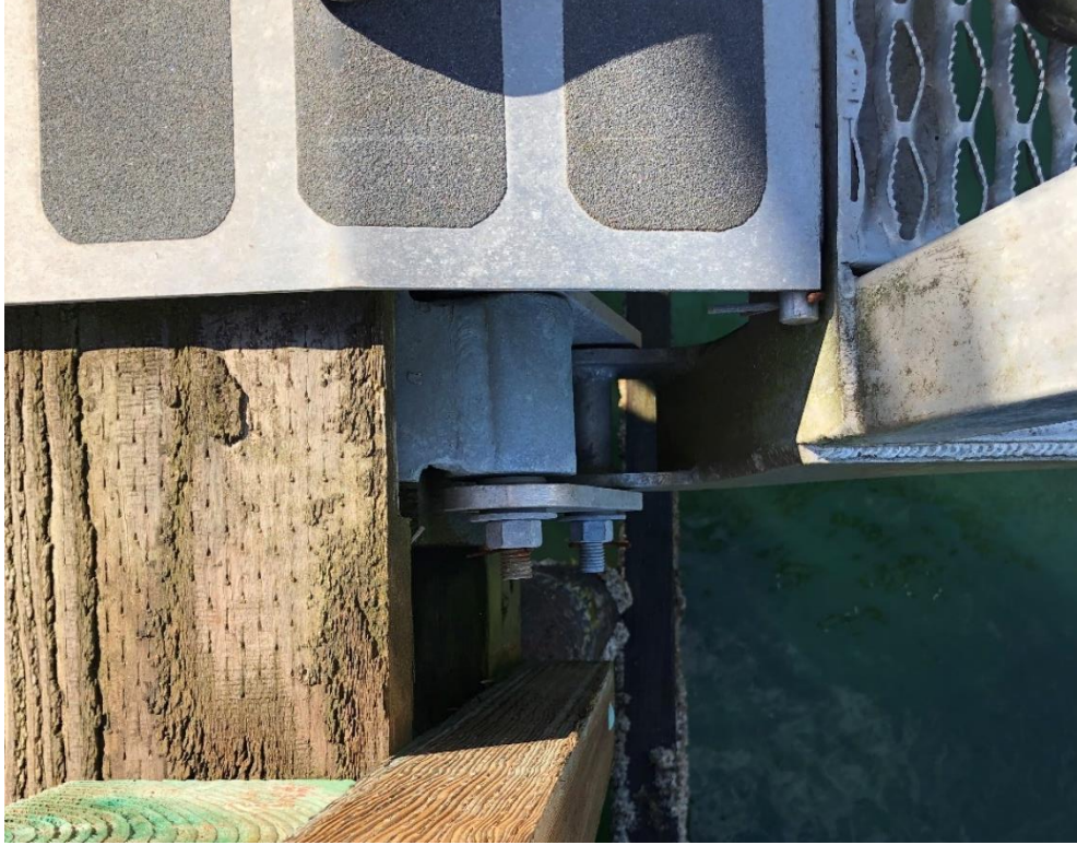
Photo 41 - Gangway Upper Hinge Connection
