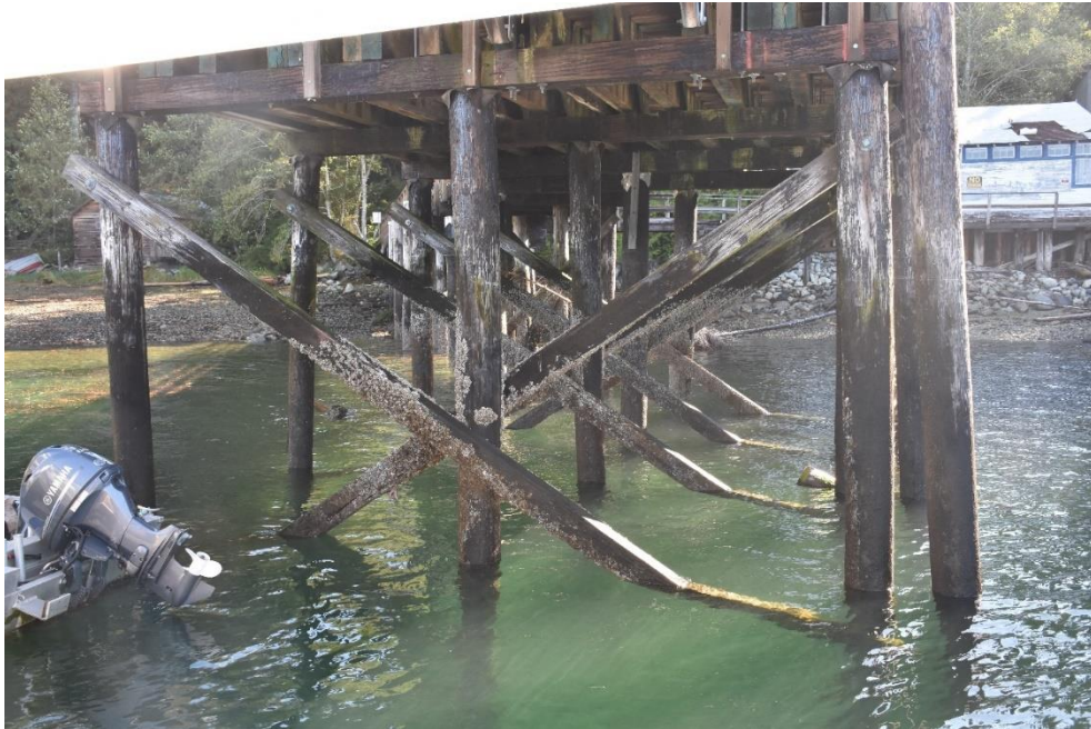
Photo 32 - General view of Cross Bracing
