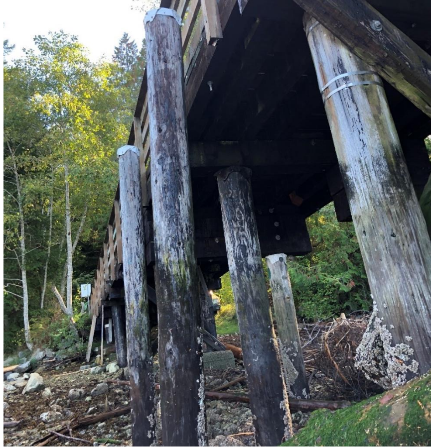
Photo 29 - North end fender piles
