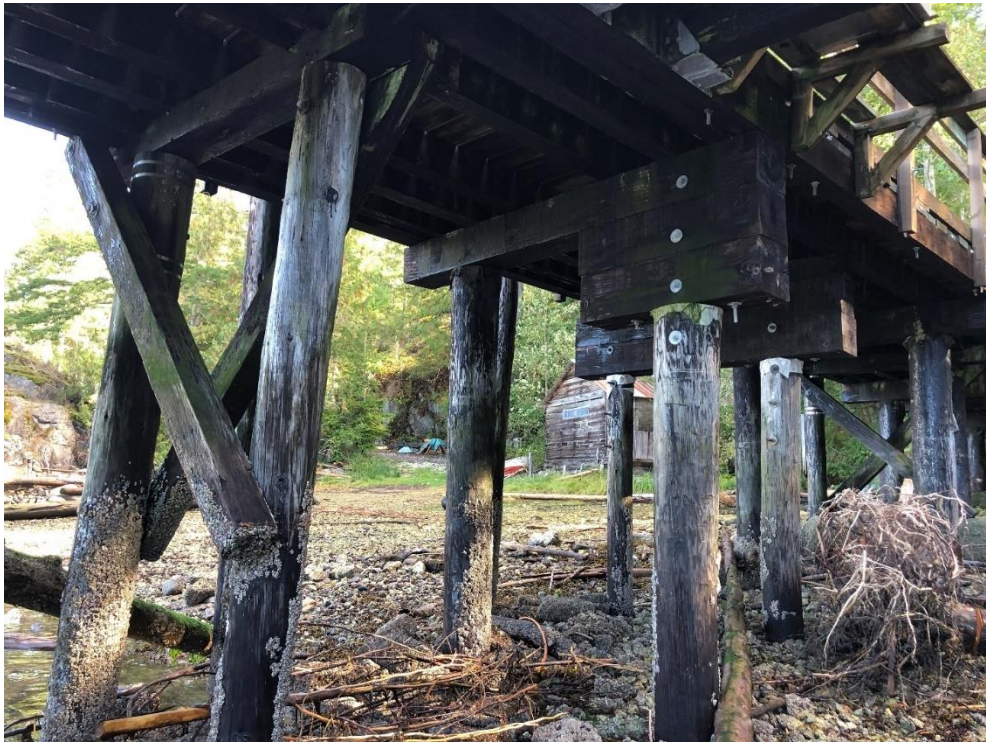
Photo 16 - Pile cap at Bent 7 and corbels
