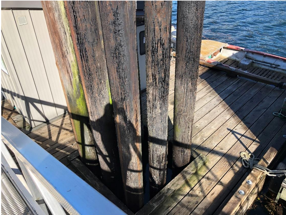
Photo 50 - East end Mooring Piles
