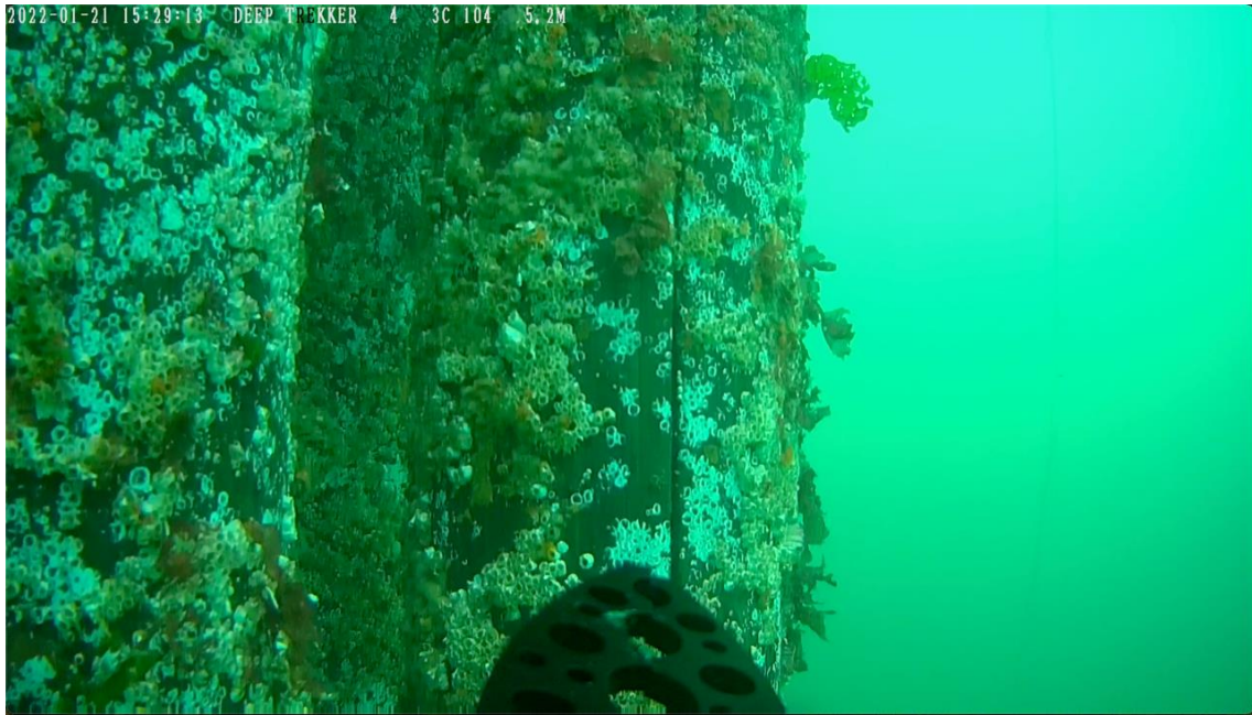
Photo 57 - West end Mooring Piles
