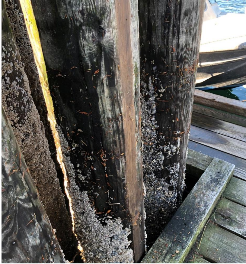
Photo 55 - West end Mooring Piles – up to 10% CSL
