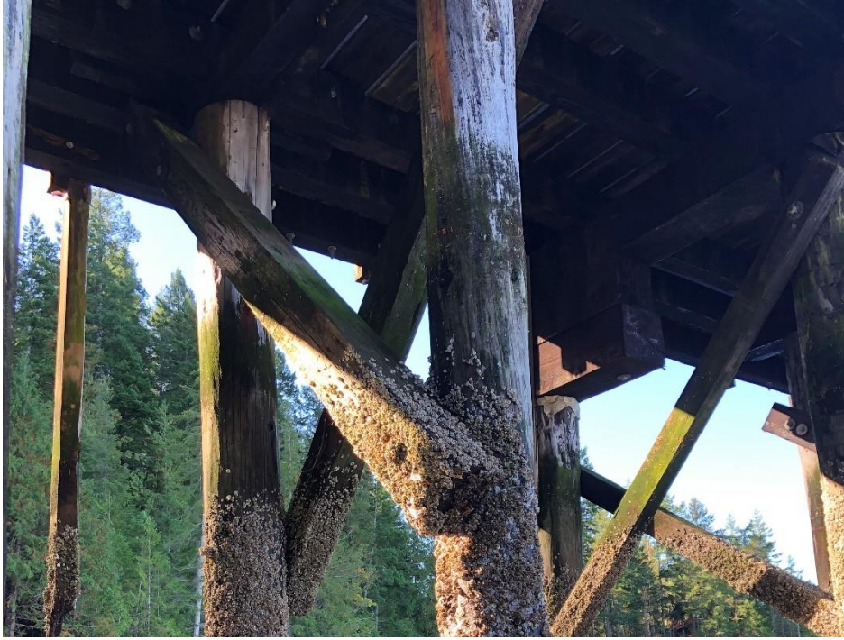
Photo 31 - General condition of the Cross Bracing
