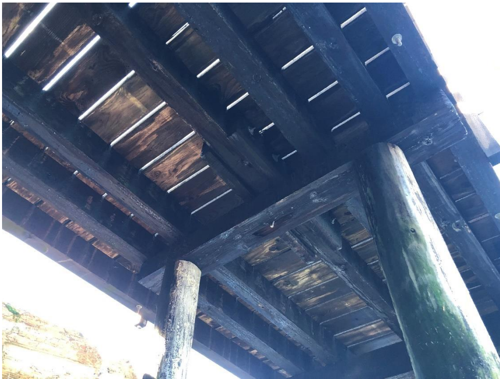
Photo 8 - Typical View of Timber Stringers
