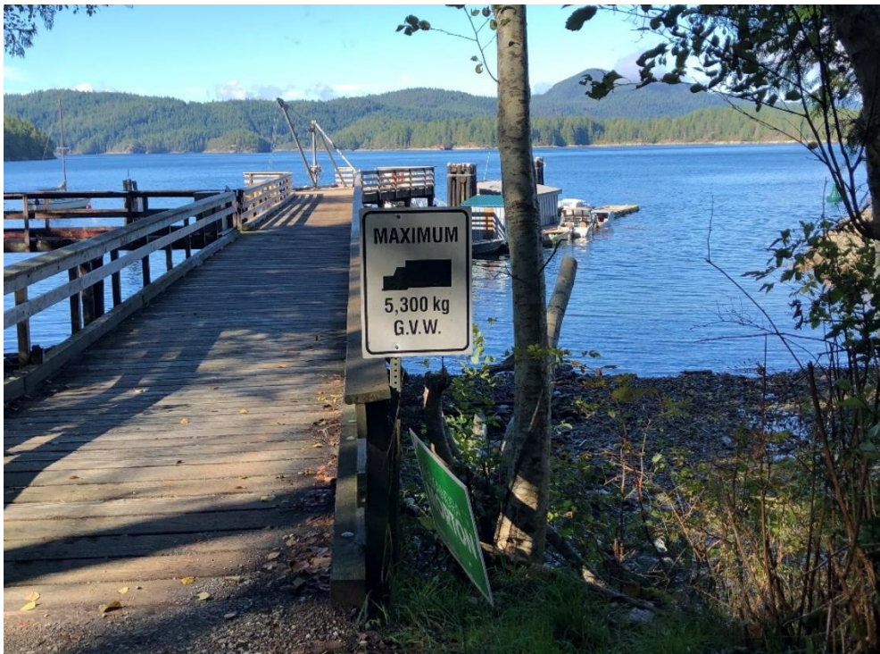
Photo 2 - Load rating sign
