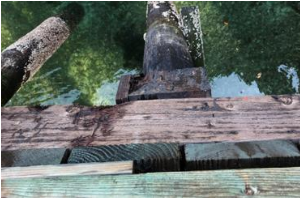
Photo 22 - Pile cap at Bent 14
