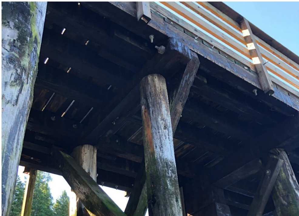
Photo 20 - Pile cap at Bent 12
