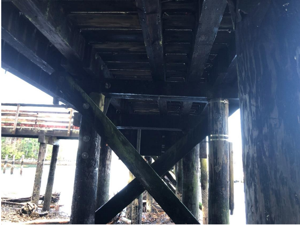
Photo 13 - Pile cap at Bent 4
