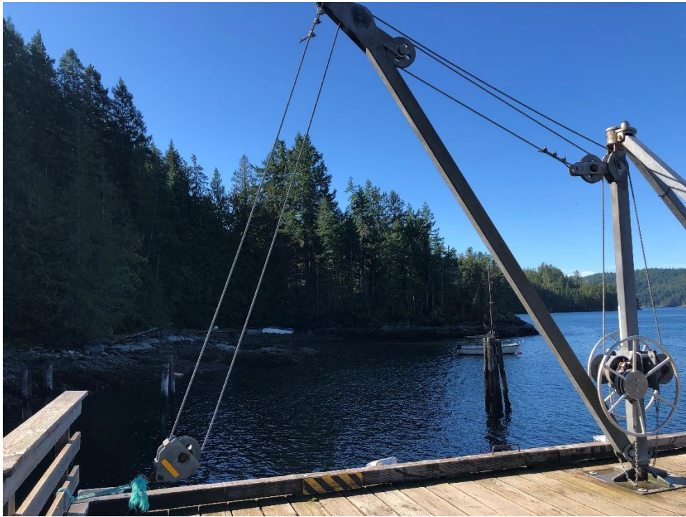
Photo 36 - Derrick Loading Crane
