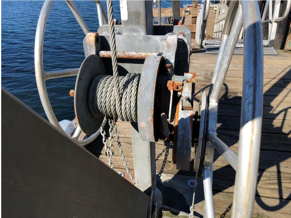
Photo 37 - Derrick Loading Crane
