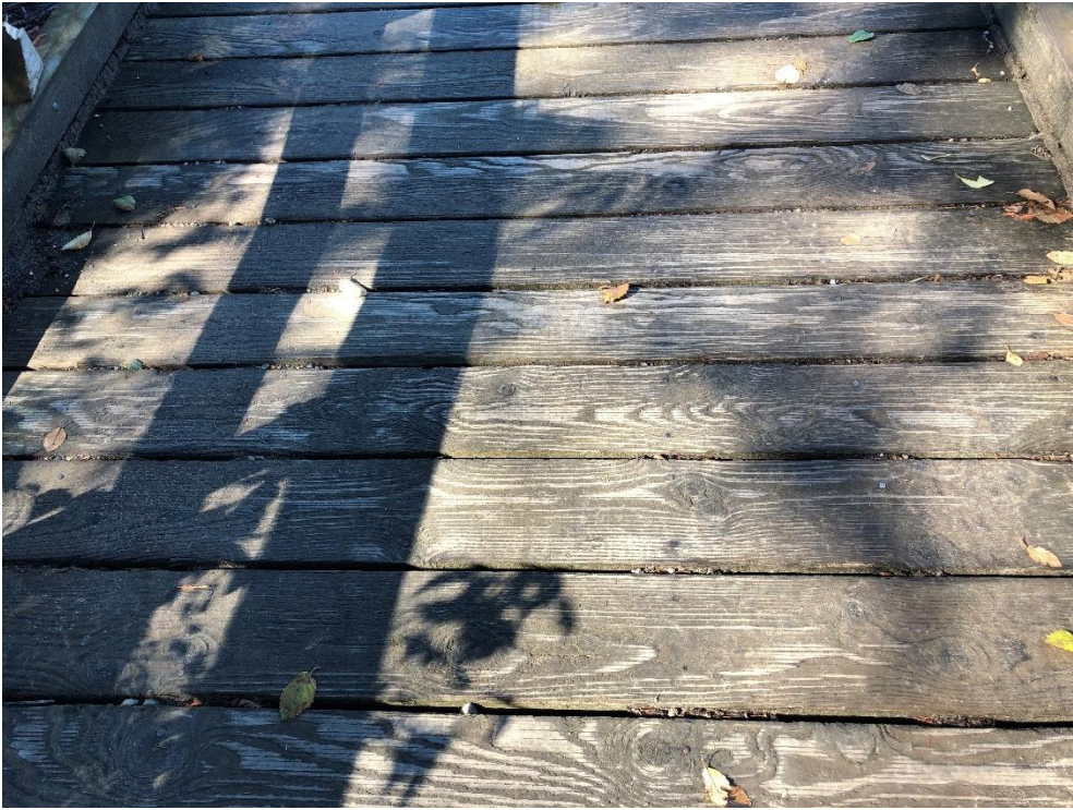
Photo 6 - Wharf Structure Decking
