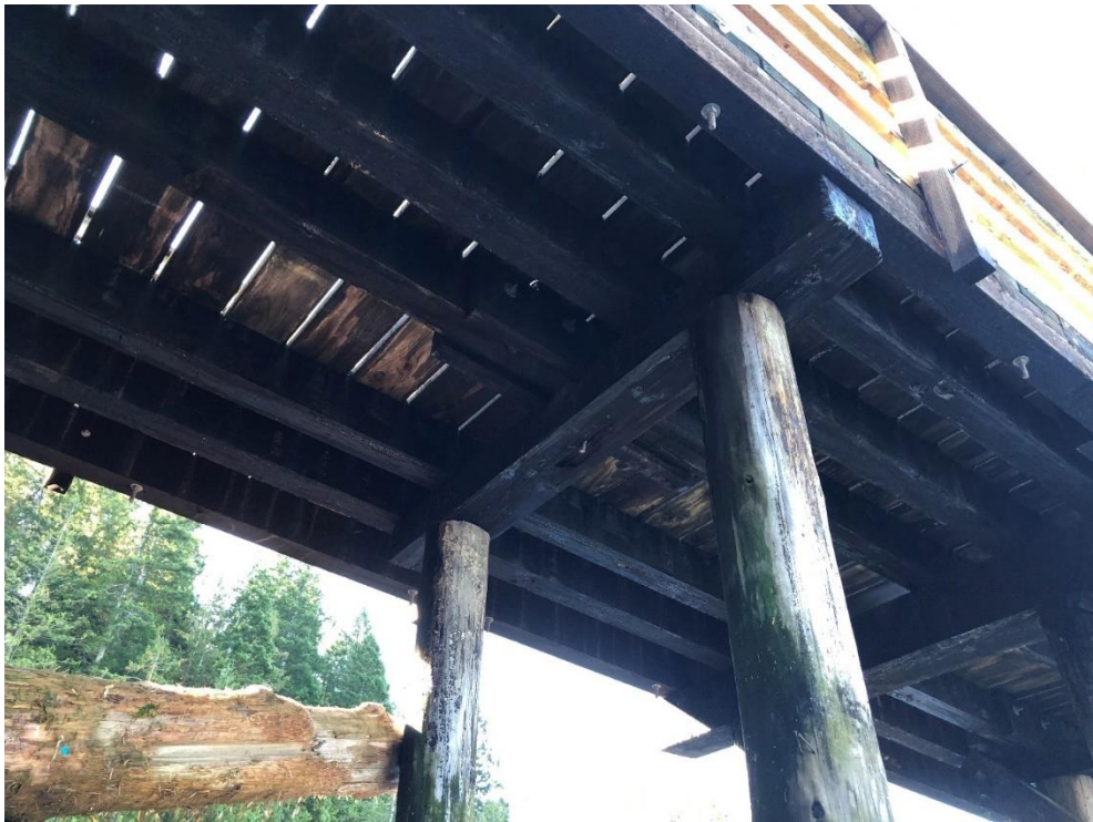
Photo 18 - Pile cap at Bent 10
