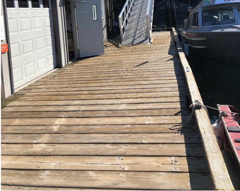
Photo 43 - Typical condition of the Main Float deck
