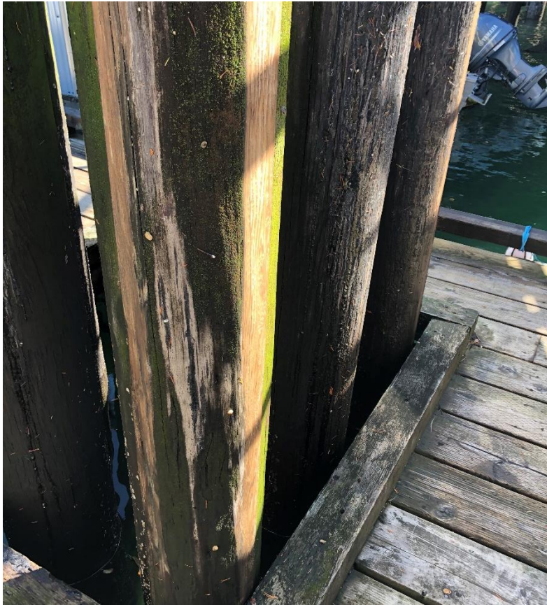
Photo 52 - East end Mooring Piles
