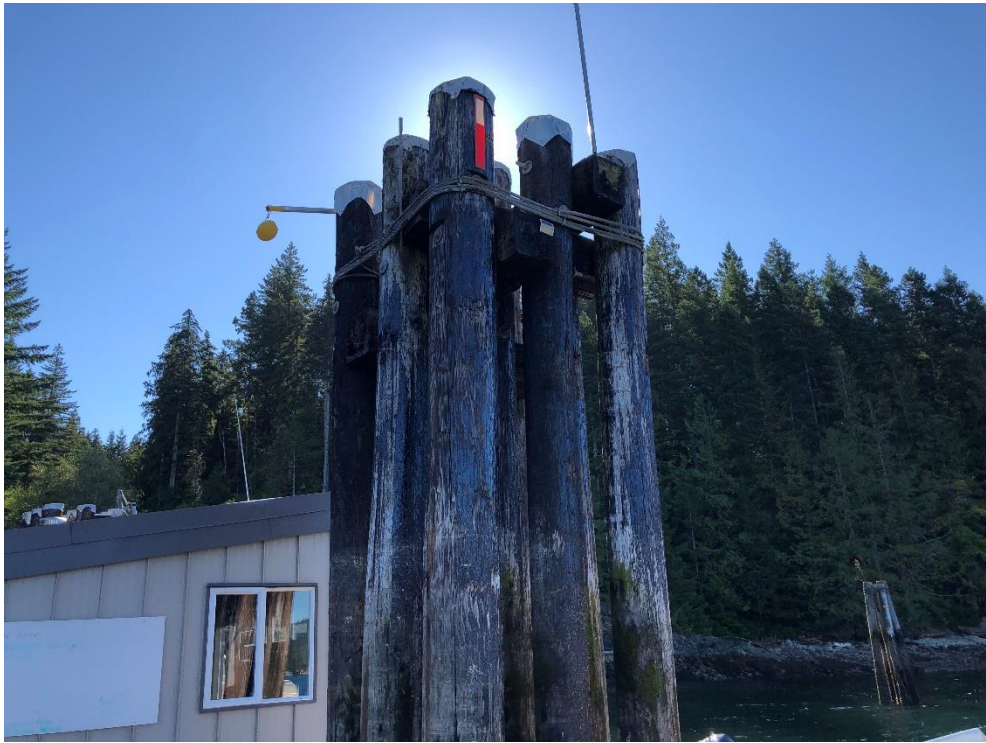
Photo 54 - West end Mooring Piles
