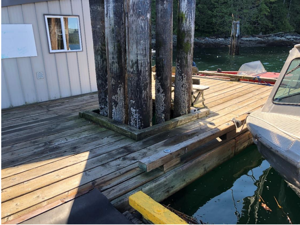
Photo 53 - West end Mooring Piles
