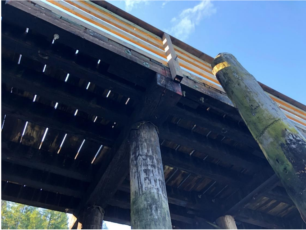
Photo 19 - Pile cap at Bent 11
