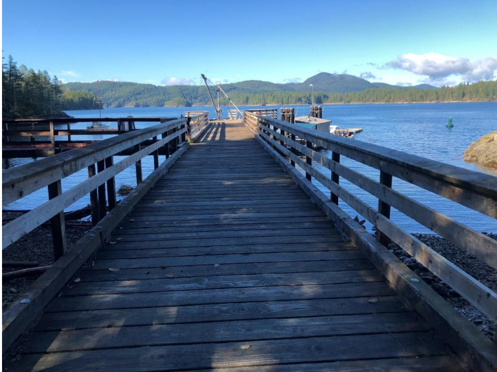
Photo 3 - Wharf Structure Topsides
