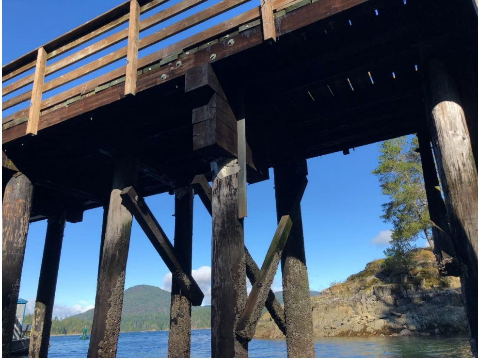
Photo 21 - Pile cap at Bent 13 with corbels
