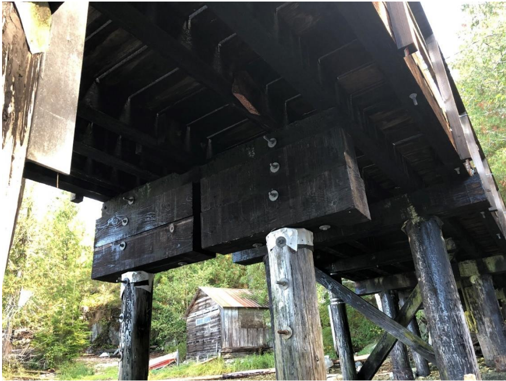
Photo 14 - Pile cap at Bent 6 and corbels
