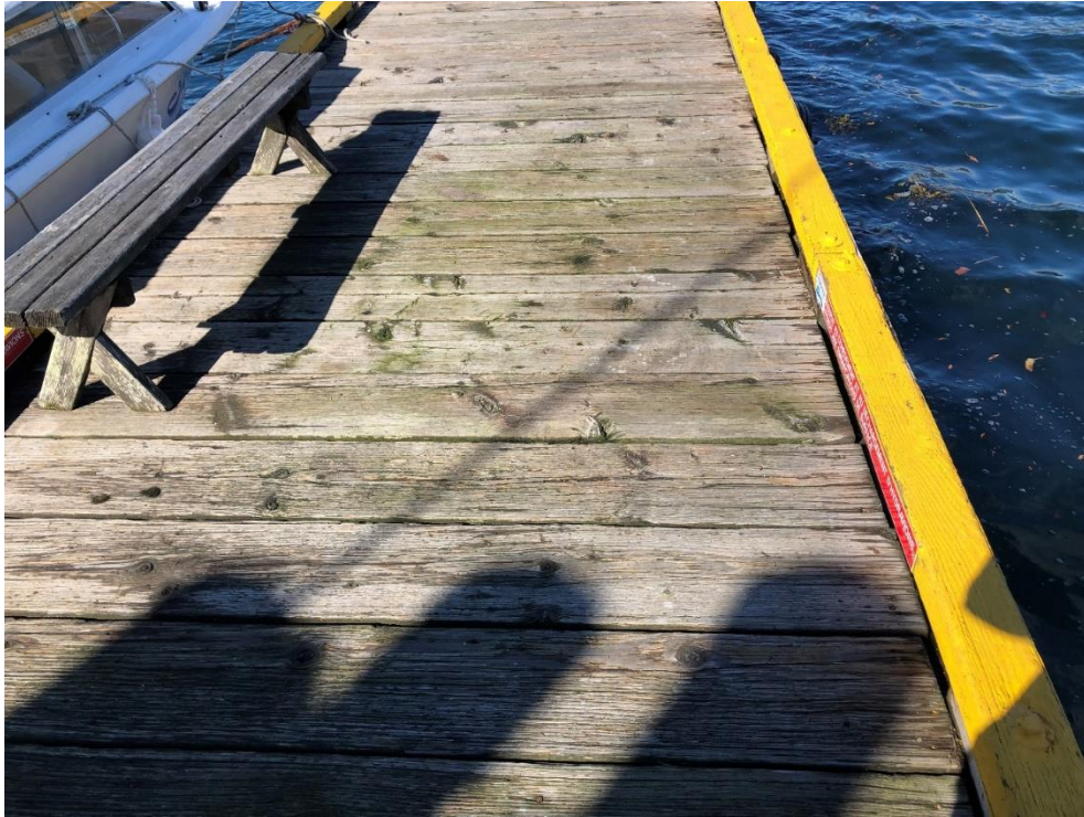
Photo 59 - Typical condition of the Seaplane Float deck
