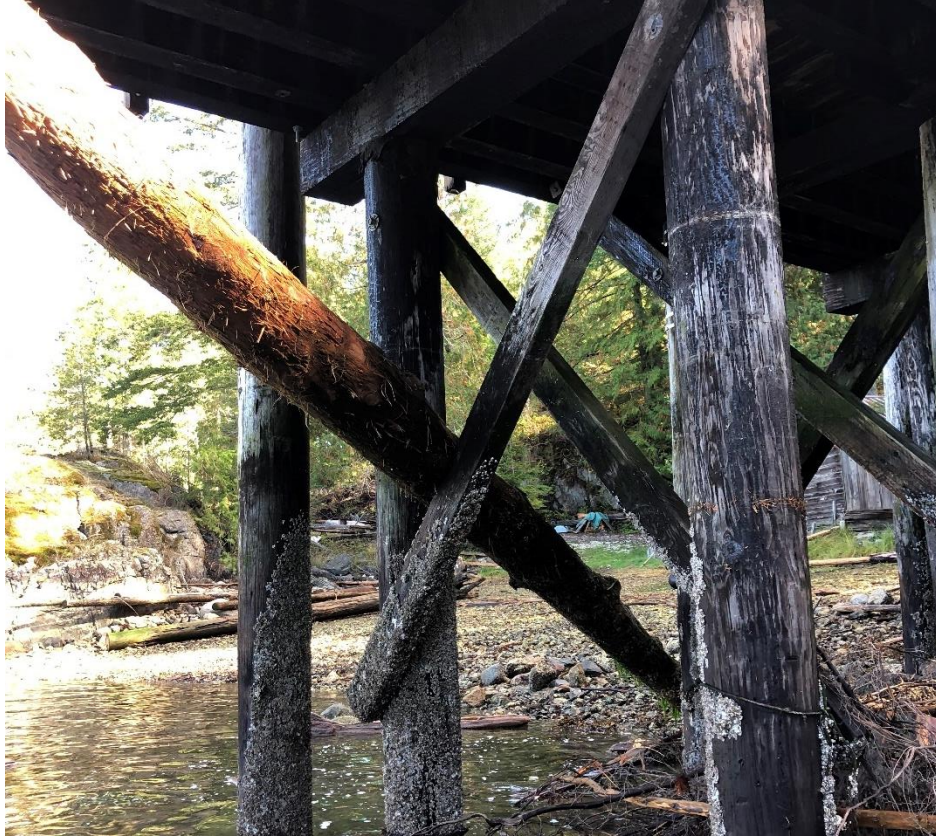
Photo 33 - Log resting on the Cross Bracing
