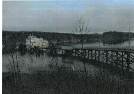
Existing Ferry Berth
