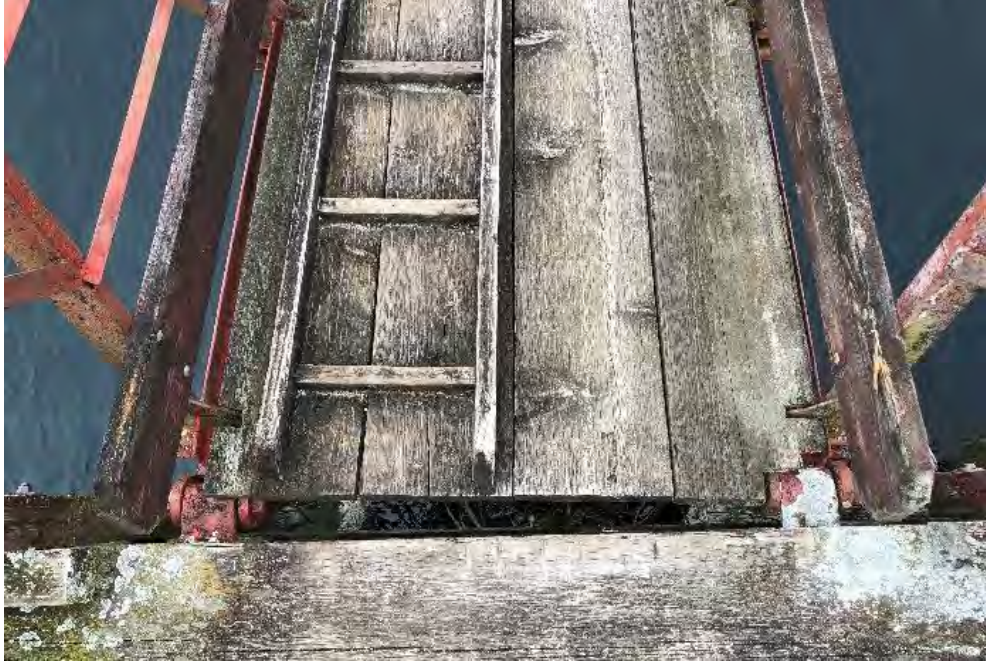
Photo 31 – Gangway Upper Hinge Connection
