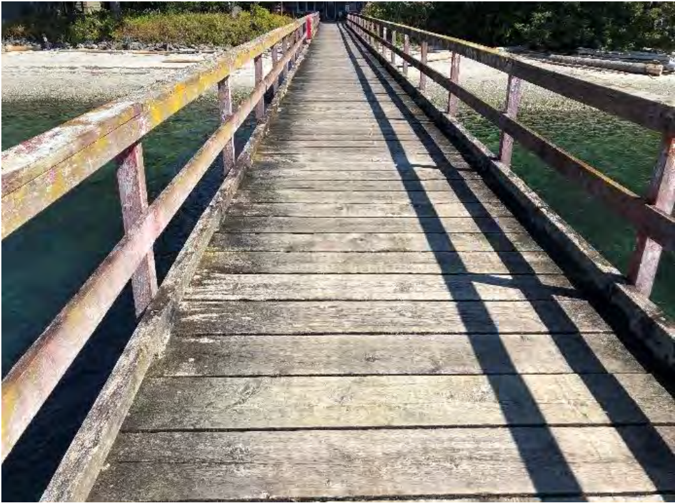
Photo 2 – Pier Structure Topsides
