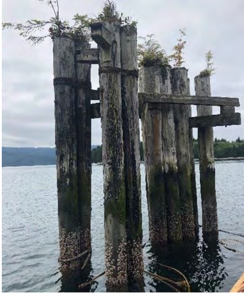
Photo 45 – South Mooring Dolphin
