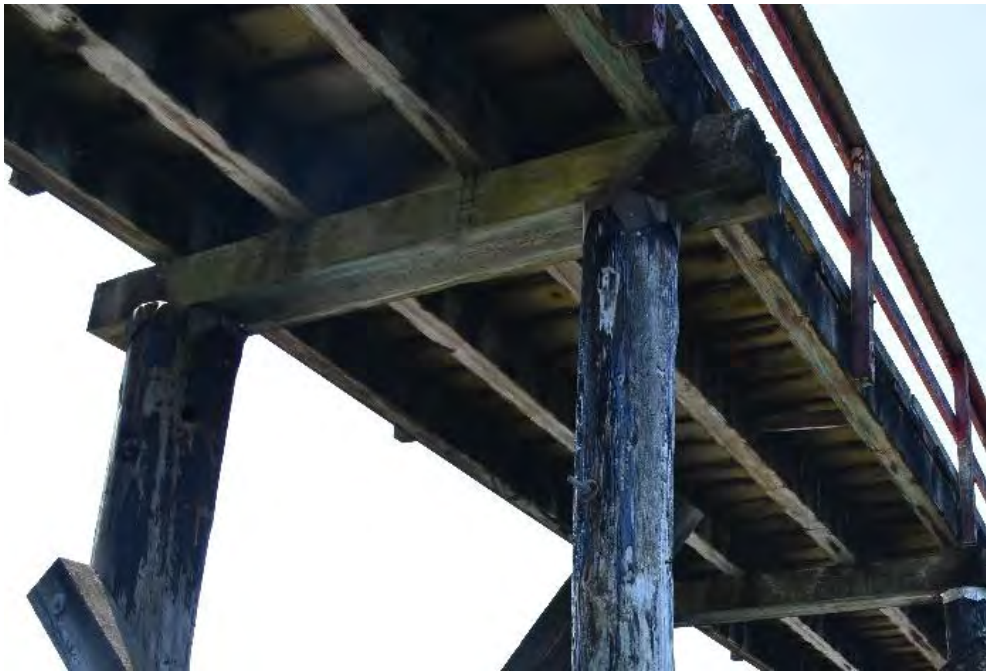
Photo 14 – Timber Pile Cap at Bent 12
