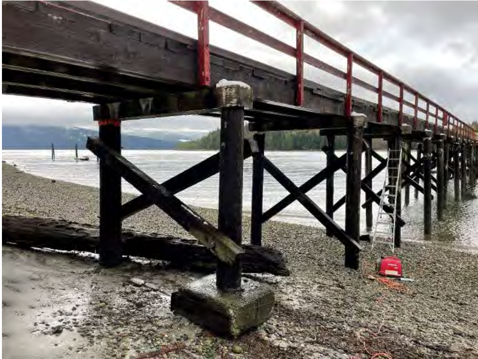
Photo 17 – Pile 4B concrete footing
