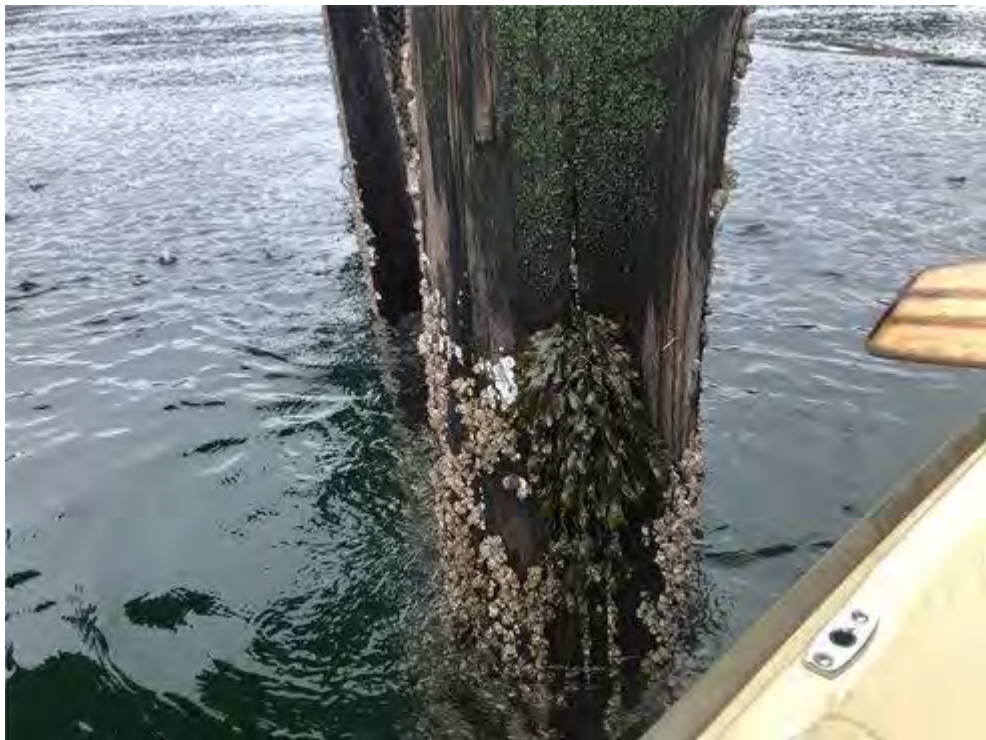
Photo 26 – Fender Pile 14A
