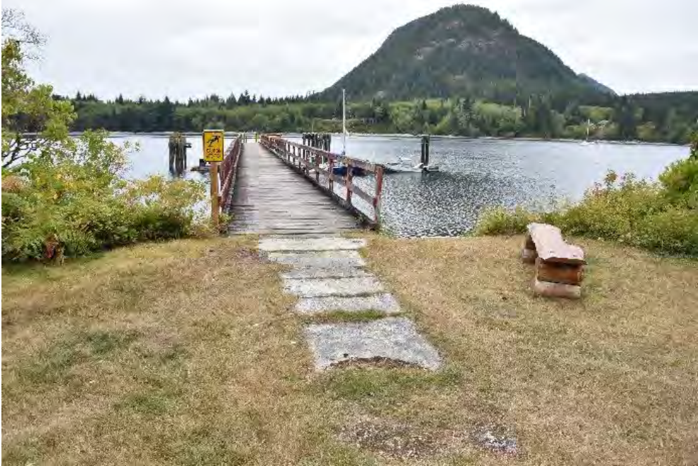
Photo 1 – Pier Approach Area
