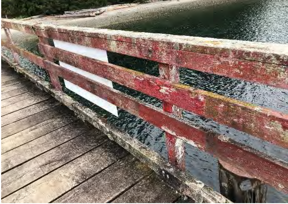
Photo 3 – Pier Structure Handrails
