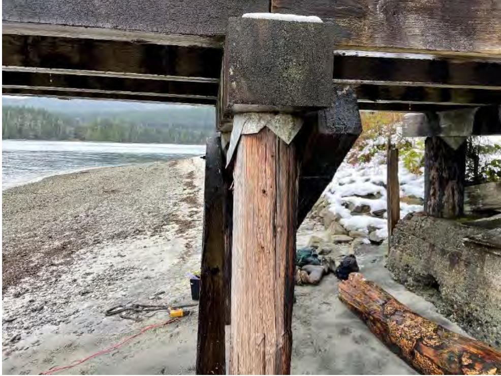
Photo 13 – Typical Timber Pile Cap End Grain
