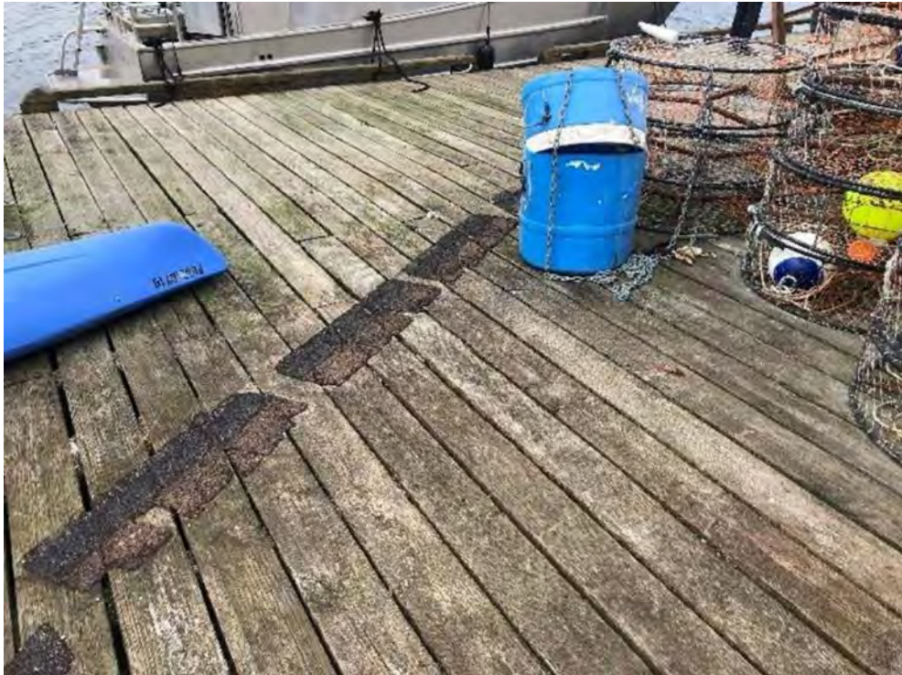
Photo 36 – General view of Float A
