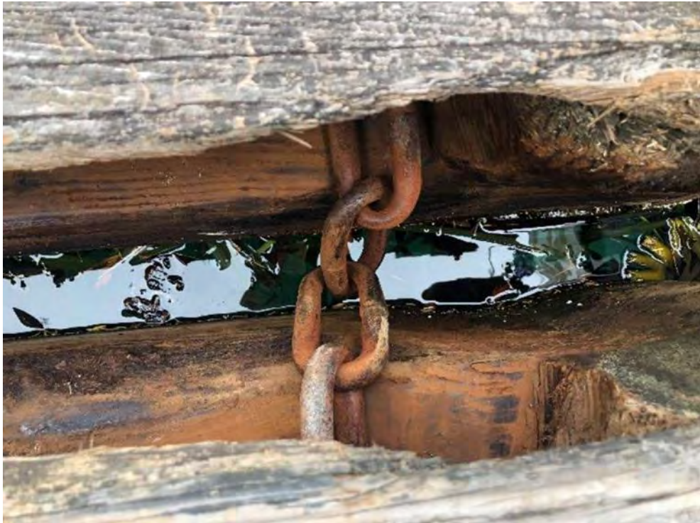
Photo 40 – Chain Connection to Float B
