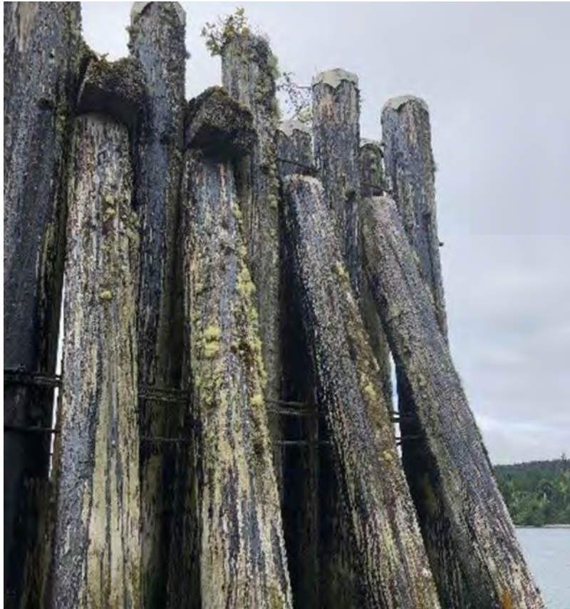
Photo 44 – North Mooring Dolphin
