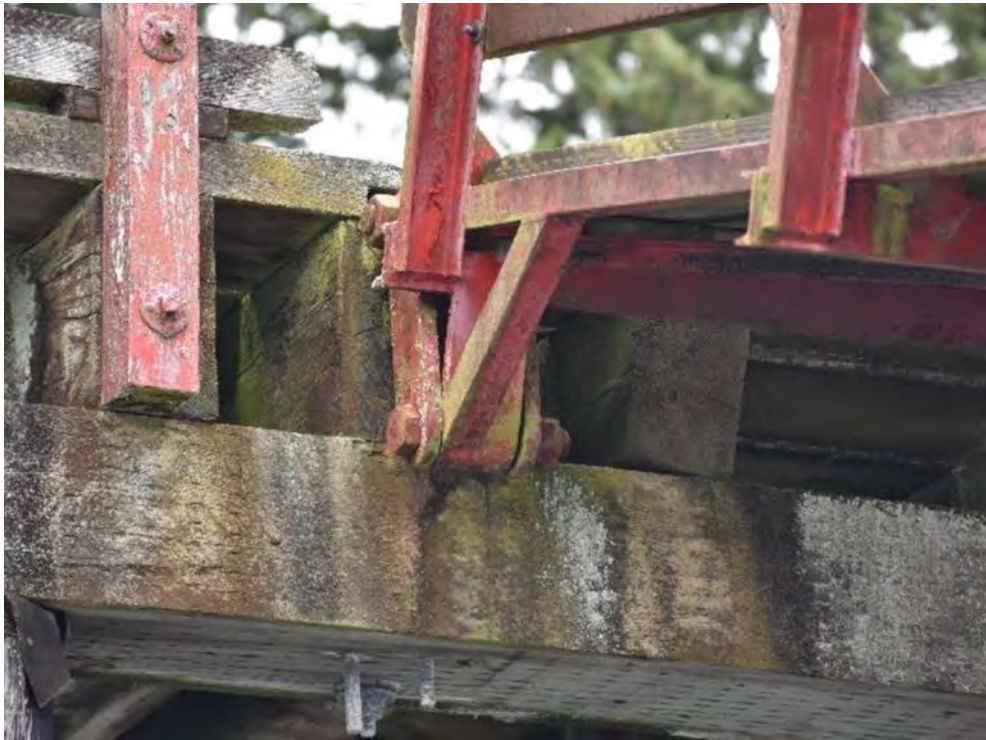
Photo 32 – Gangway Upper Hinge Connection
