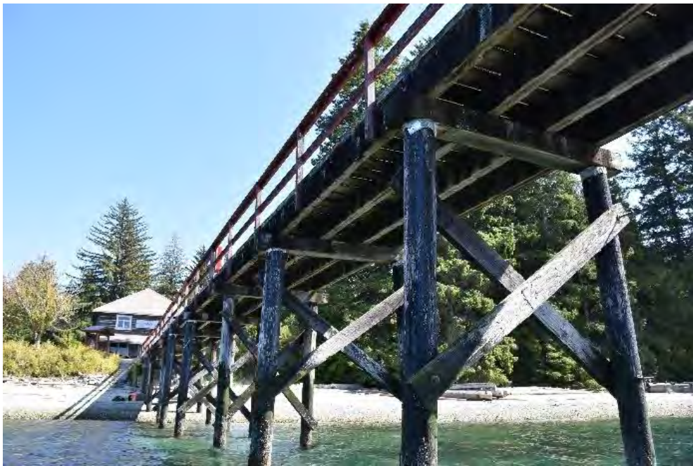
Photo 12 – General View of Timber Pile Cap Bents
