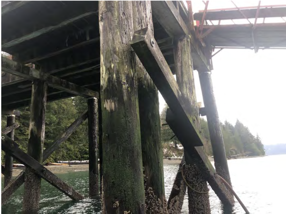
Photo 30 – Cross Bracing at Bent 15
