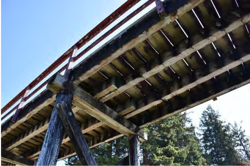
Photo 11 – Typical View of Timber Stringers
