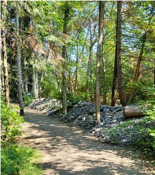
Photo 11: A Windrow Berm in the Left Floodplain to Protect a Wellhead (August 7, 2024)
