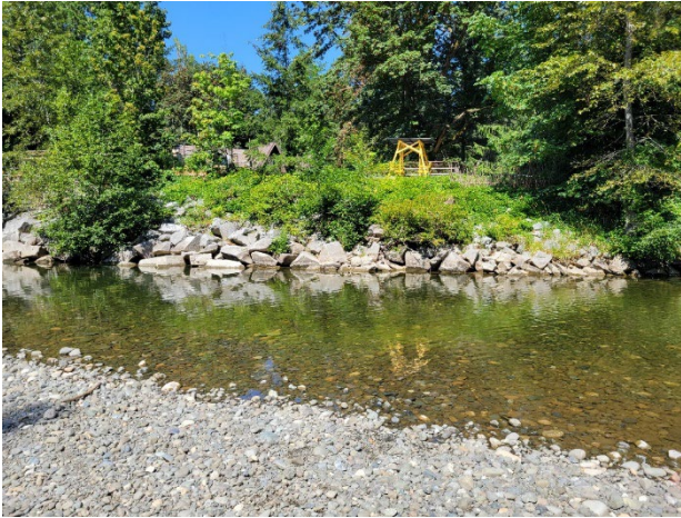
Photo 1: Established Trees and Vegetation, Especially Himalayan Blackberry, in the Riprap Apron Between Hwy 19a Bridge and Regent Road Bridge (August 7, 2024)
