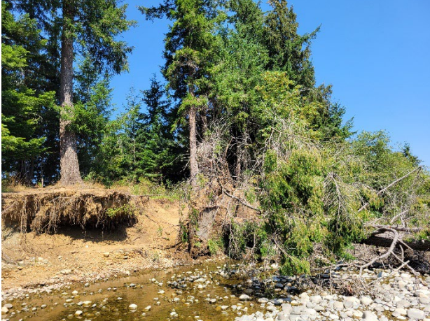
Photo 5: Actively eroding Bank Undercutting Several Mature Trees (August 7, 2024)
