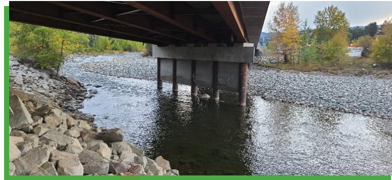
Photo 4: Bridge Inspection on Highway 3 over the Similkameen River
