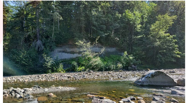
Photo 8: Eroding Silt Bluff on the Right Bank at Lorna Lane (August 7, 2024)
