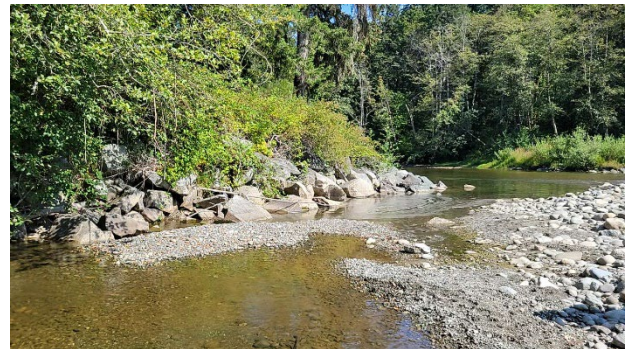
Photo 4: Riprap Extending up a Side Channel Towards the Glenmore Dike and into Heavy Vegetation (August 7, 2024)
