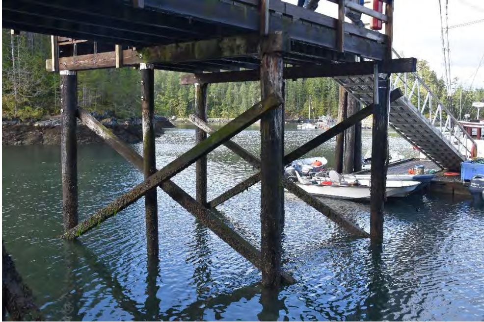
Photo 19 - General view of Cross Bracing
