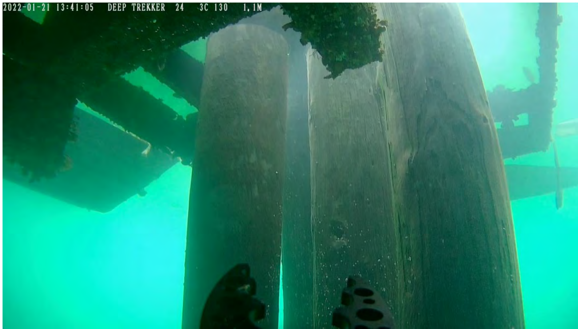
Photo 29 - South Mooring Piles
