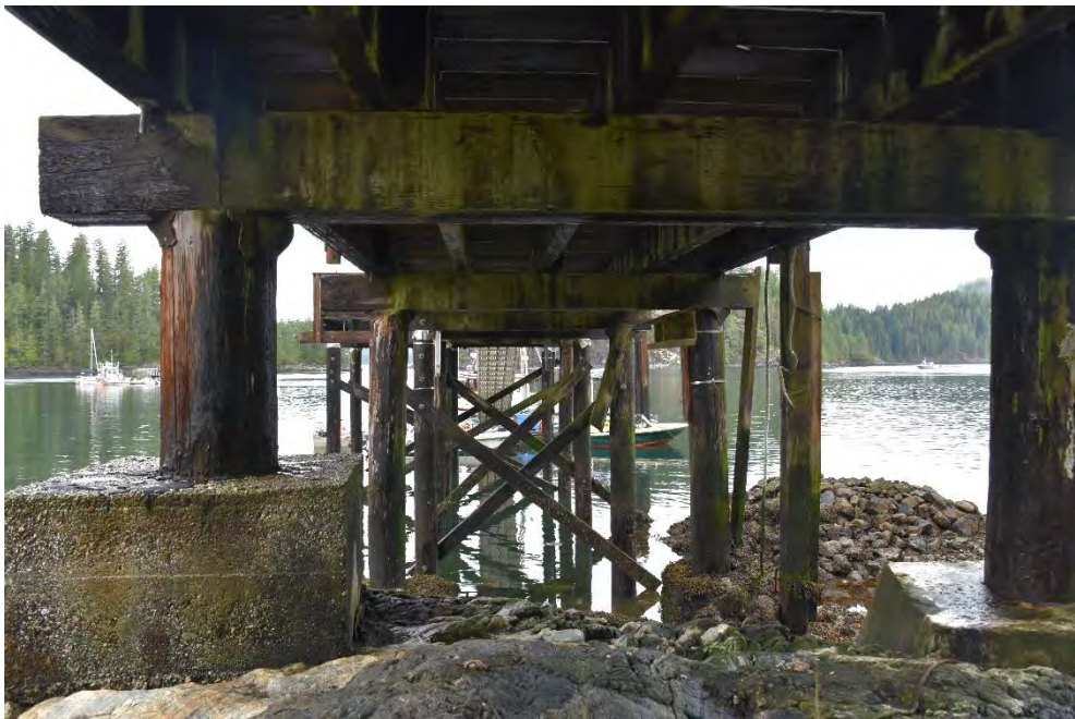
Photo 6 - General view of the Pile Cap Bents
