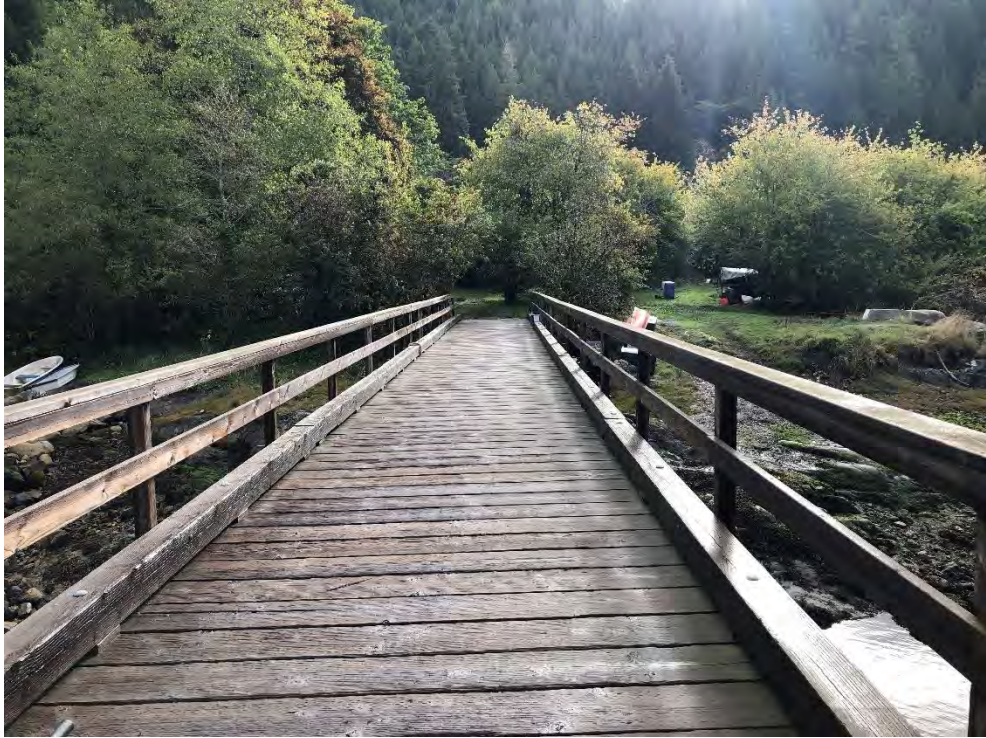
Photo 3 - Topsides of the Wharf Structure
