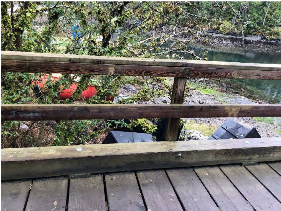
Photo 4 - General View of the Handrails
