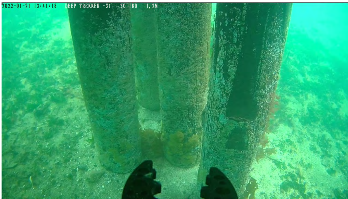
Photo 30 - South Mooring Piles
