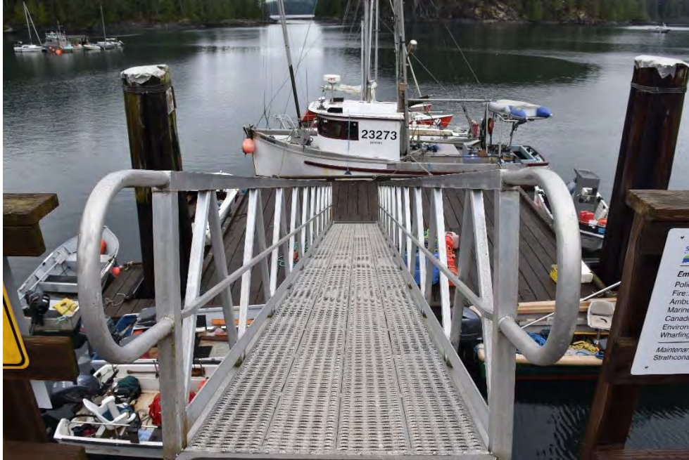
Photo 21 - General View of Aluminum Gangway
