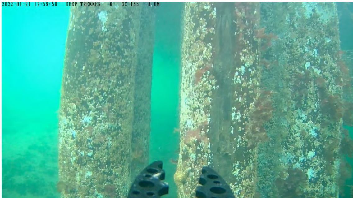
Photo 32 - North Mooring Piles
