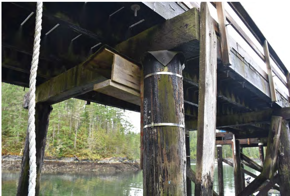
Photo 18 - Pile 5A with typical existing banded repair
