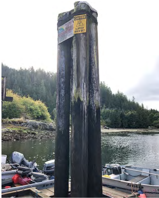
Photo 27 - South Mooring Piles
