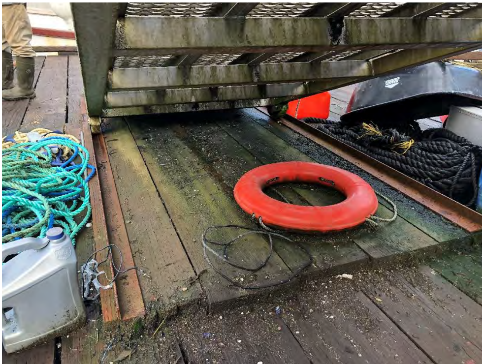
Photo 22 - Gangway slider plate and rollers
