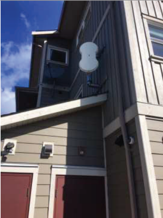
3. Point to point radio transceiver on Kyuquot First Nation Band Office
