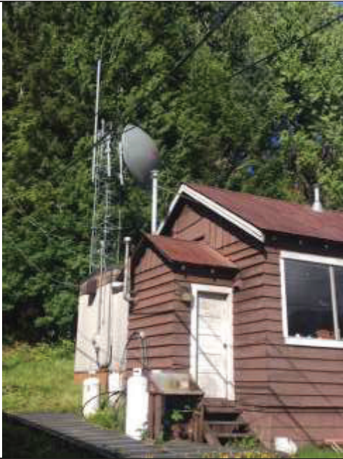
1. TELUS microwave receive site on Walters Island
