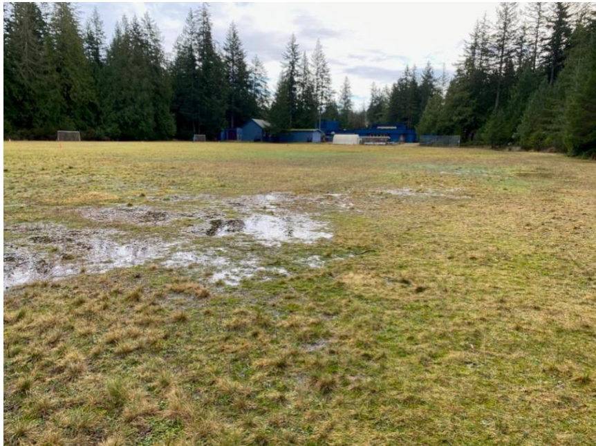
Figure 10. Water is pooling seasonally in the sports field which would be improved as part of the project.
