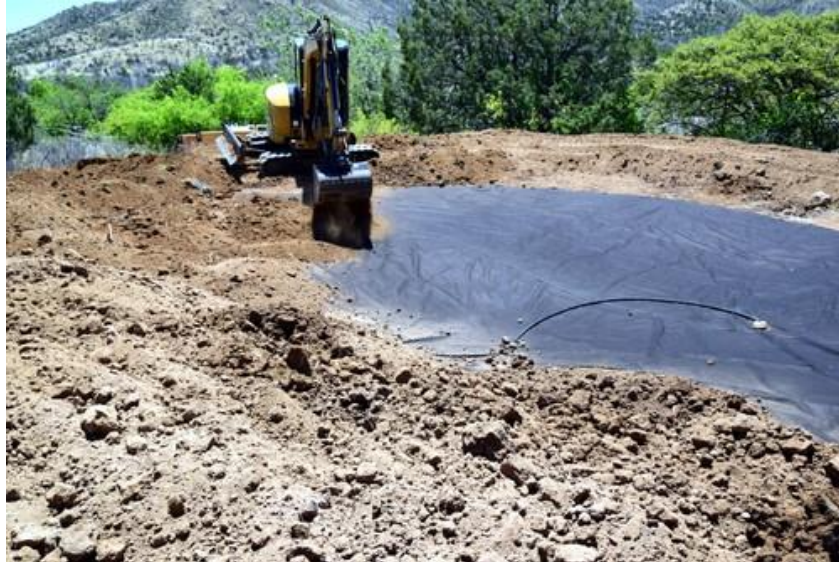
Figure 15. The excavator is used to place soil over the liner and geo-textile pads. Heavy equipment must be kept off of the liner at all times to protect it from damage. Photo: Biebighauser.
