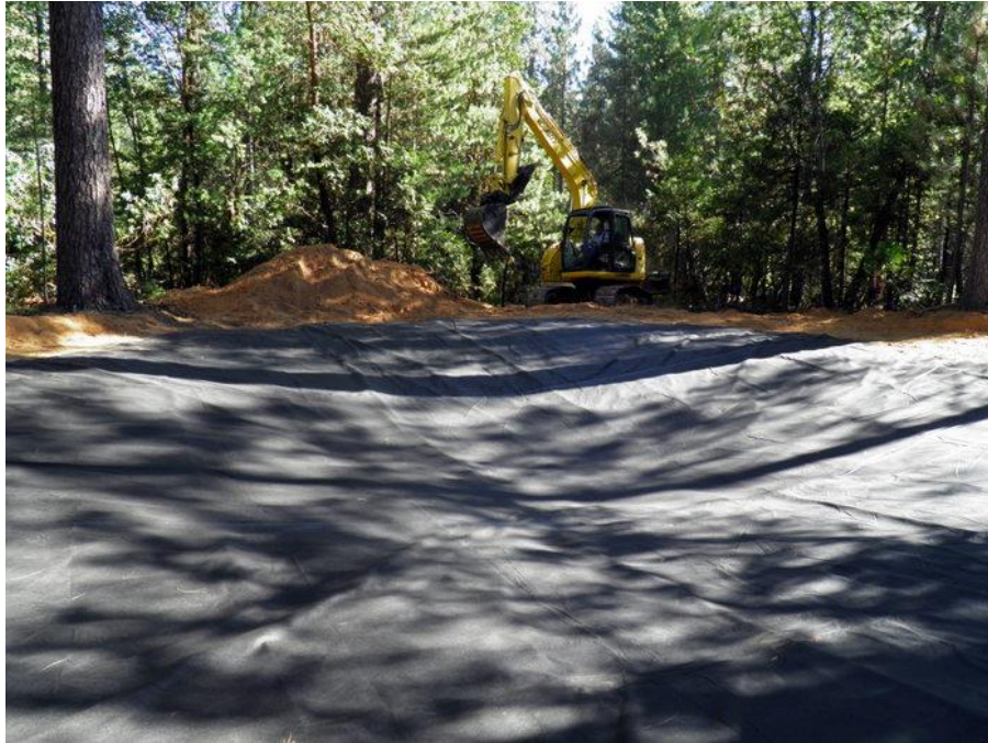
Figure 12. An aquatic-safe liner, sandwiched between layers of geotextile, is ready for covering with soil by the excavator. It is critical that the liner and geo-textile pads be ordered one piece, and factory seamed. Photo: Biebighauser.
