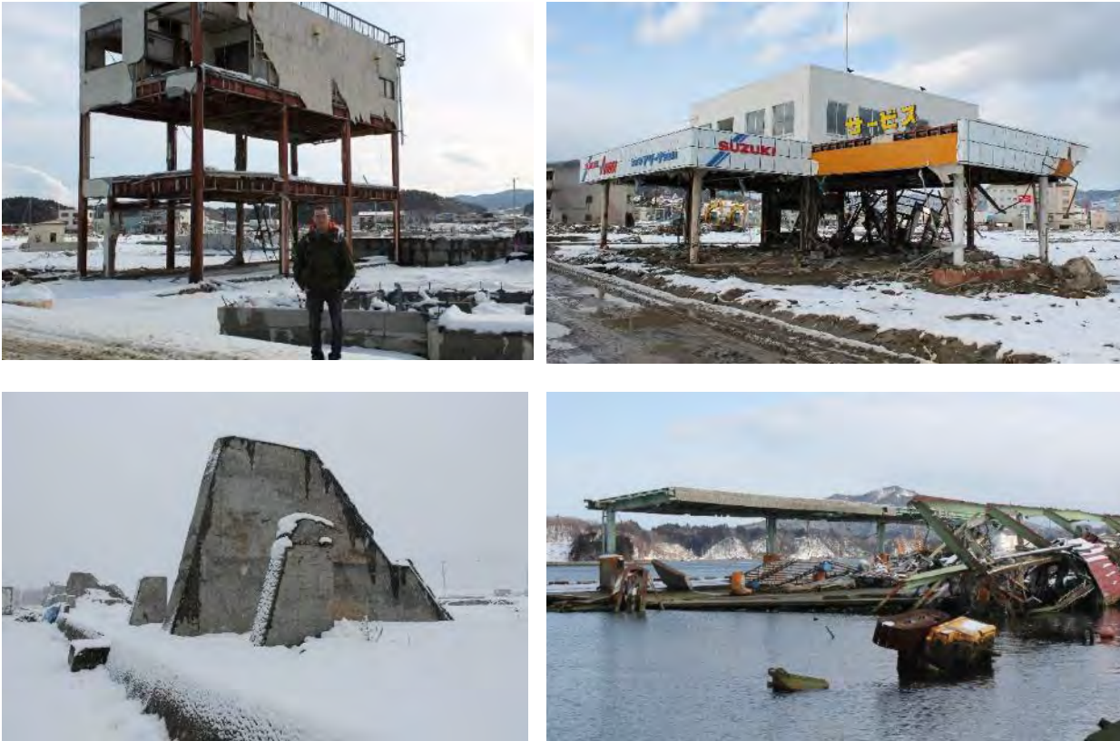
Figure 4.2 Damaged infrastructure in the City of Miyako, Japan following the 2011 Tohoku tsunami. Top photos show damage to inland buildings, bottom left photo shows remains of tsunami protection wall, and bottom right shows damage to port installations.
