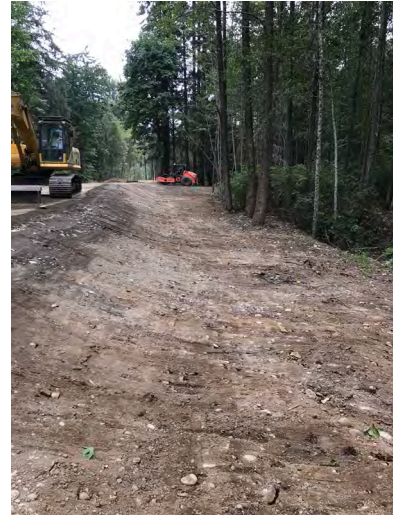
Photo 4: Sta. 0+150 (RHS) facing Up Chainage
