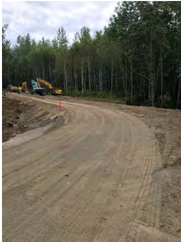
Photo 1: Overview of Work Area from Sta. 0+000
