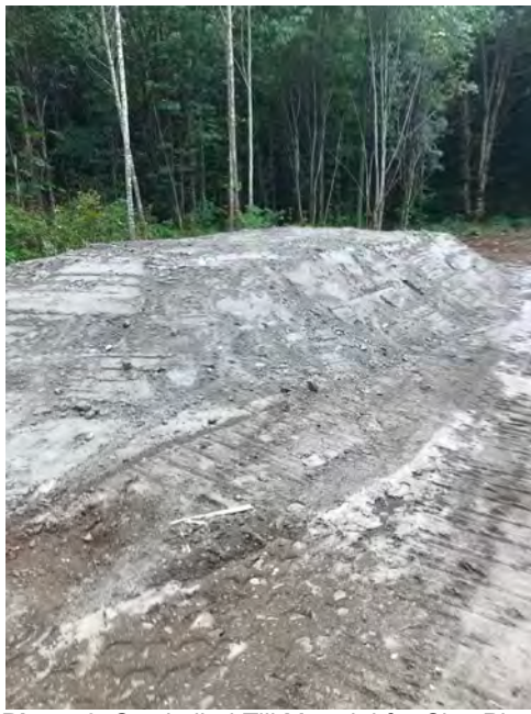
Photo 3: Stockpiled Till Material for Clay Plug
