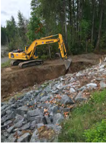
Photo 1: Outlet Channel Maintenance
