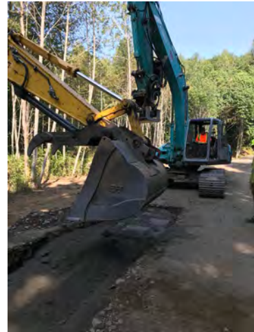
Photo 2: Backfilling and Compaction
