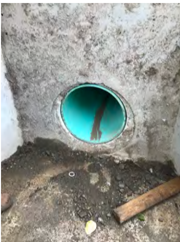
Photo 3: Headwall to be Grouted Smooth
