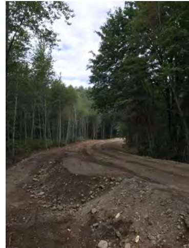
Photo 4: Temporary Dike Widening
