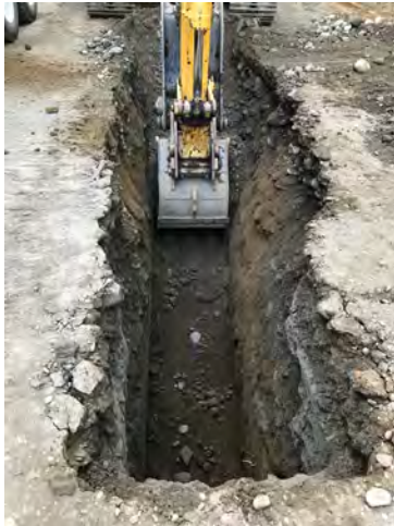
Photo 1: Excavation to Approved Subgrade
