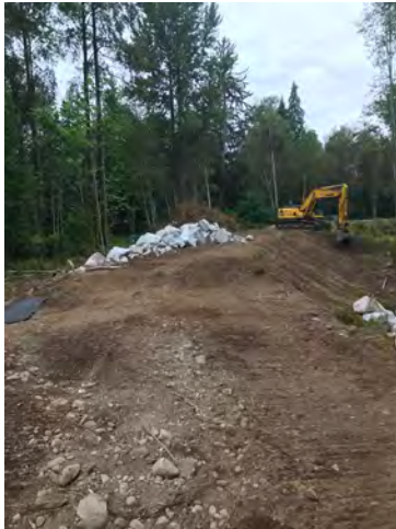
Photo 3: Access Ramp to Private Property
