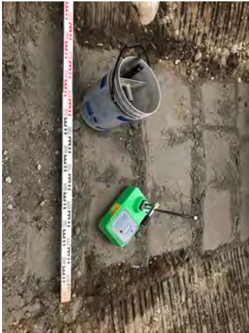
Photo 3: Backfilling and Compaction at Sta. 0+060
