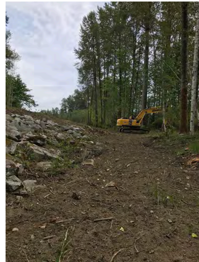
Photo 8: Sta. 0+310 (RHS) facing Up Chainage
