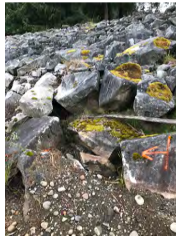
Photo 4: Marked Riprap Repair Area
