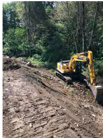
Photo 2: Clearing and Grubbing, Sta. 0+285
