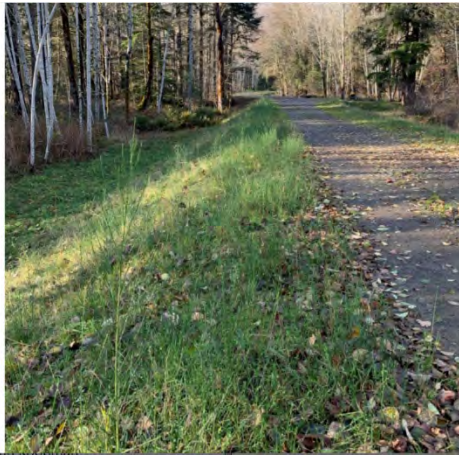
Figure 2 – A portion of the Glenmore Road dike on riverside slope
