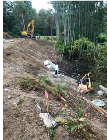
Photo 4: Equipment for Slab Preparation
