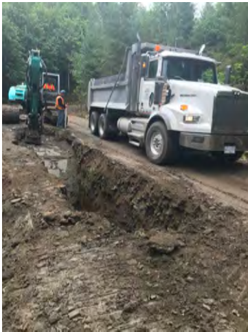
Photo 3: Flow of Traffic Maintained
