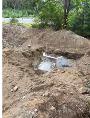
Photo 2: Concrete at Headwall
