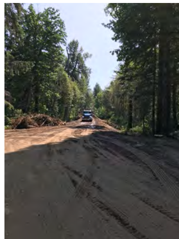
Photo 4: Trucking Sandy Organic Material Offsite
