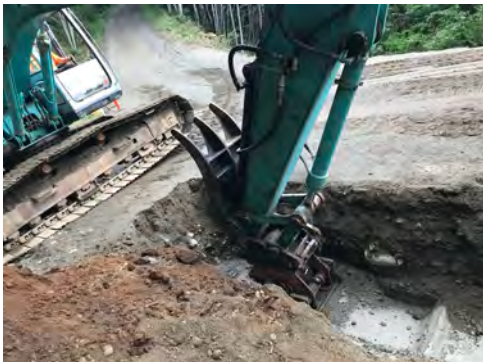
Photo 3: Backfilling and Compaction at Sta. 0+005
