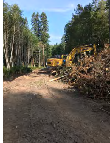
Photo 2: Clearing and Grubbing, Sta. 0+290
