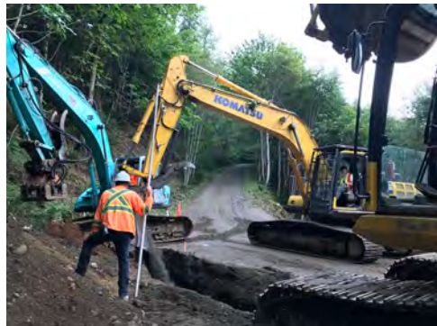
Photo 4: Backfilling and Compaction at Sta. 0+005
