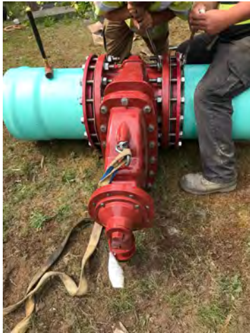
Photo 3: Preparation of Gate Valve
