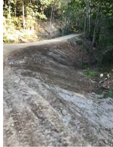
Photo 2: Sandy Organic Material at Sta. 0+000
