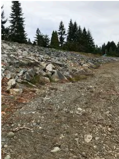
Photo 11: Sta. 0+450 (RHS) facing Up Chainage
