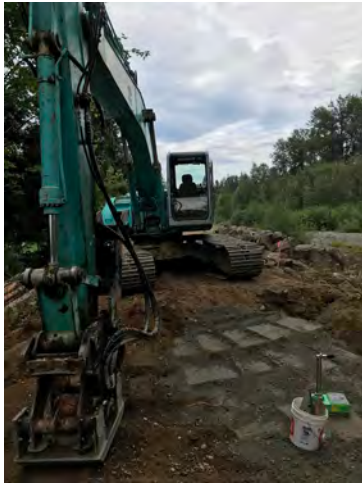
Photo 3: Backfilling and Compaction
