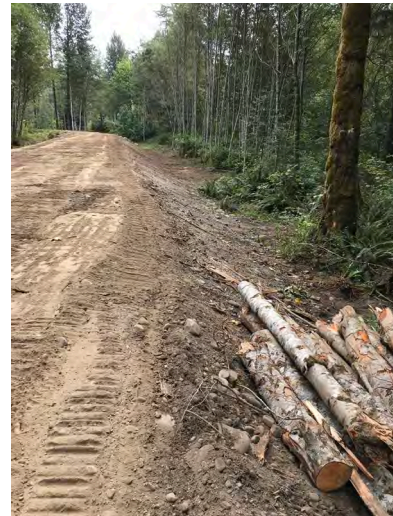
Photo 6: Sta. 0+250 (RHS) facing Up Chainage
