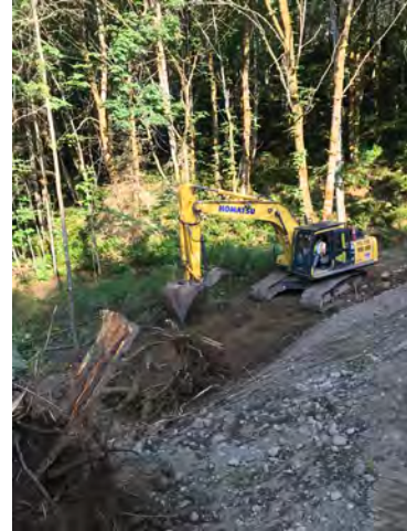
Photo 2: Clearing and Grubbing, Sta. 0+020
