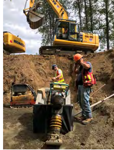
Photo 2: Backfilling and Compaction
