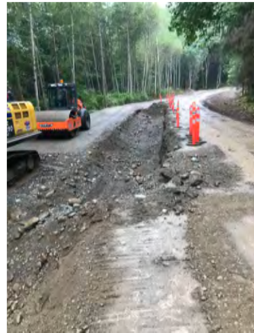
Photo 4: Construction of Temporary Bypass
