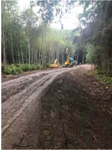
Photo 1: Overview of Work Area from Sta. 0+150
