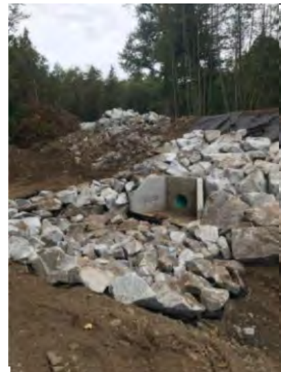
Figure 3 – Riprap and flood box at outlet channel of dike
