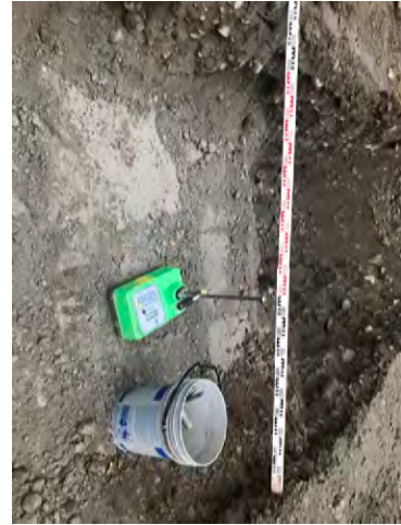
Photo 2: Backfilling and Compaction, Sta. 0+075
