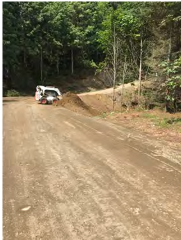
Photo 2: Placing Sandy Organic Material at Sta. 0+000
