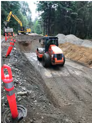
Photo 1: Compaction of Full Rebuild Section
