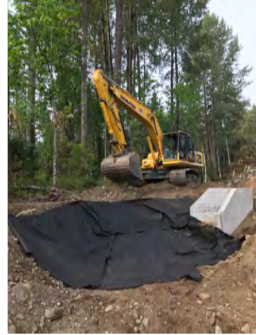
Photo 2: Outlet Channel at Headwall
