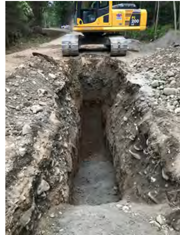
Photo 2: Excavation at Sta. 0+060
