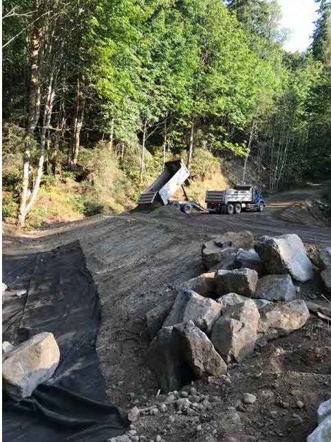
Photo 1: Filter Fabric at Sta. 0+008-0+023 per S.I.
