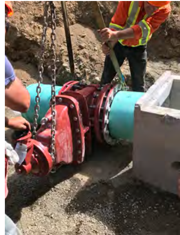
Photo 4: Installation of Gate Valve
