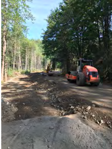
Photo 1: Backfilling and Compaction in Rebuild Section
