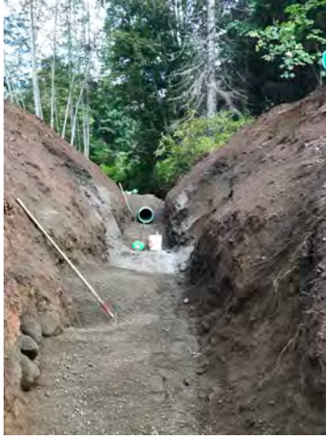
Photo 1: Clay Plug at Flood Box
