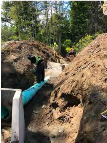
Photo 3: Backfilling and Compaction
