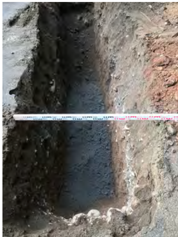
Photo 2: Excavation at Sta. 0+005
