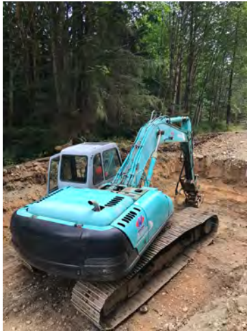
Photo 3: Compaction of Subgrade in Rebuild Section
