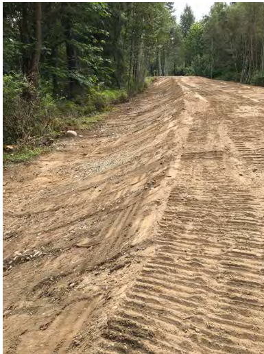
Photo 5: Sta. 0+250 (LHS) facing Up Chainage
