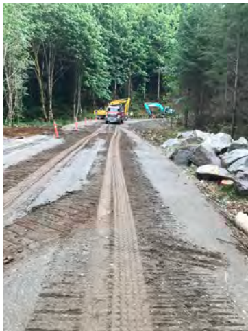
Photo 1: Overview of Work Area
