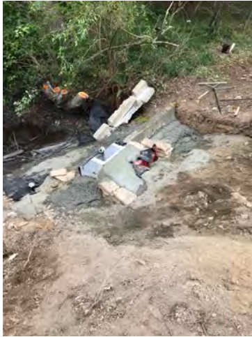
Photo 1: Concrete at Sump and Valve
