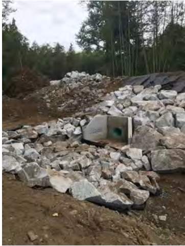
Photo 1: Riprap at Outlet Channel
