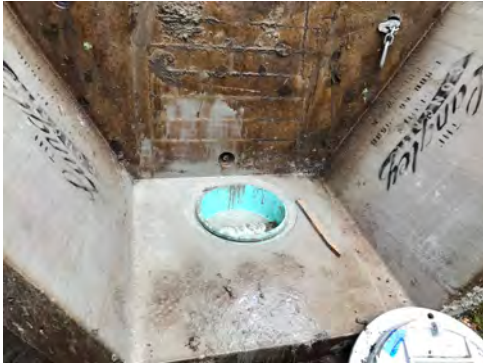
Photo 1: Flood Box Headwall Modification
