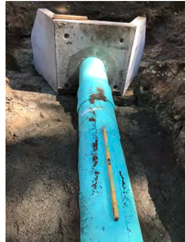
Photo 4: Confirmation of Pipe Grade
