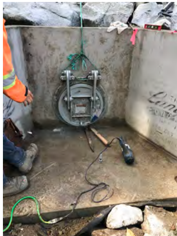
Photo 2: Installation of Flap Gate (see NOTE)
