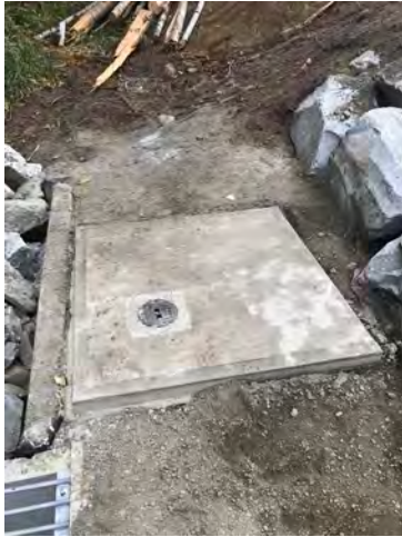
Photo 1: Concrete Pad at Flood Box Inlet
