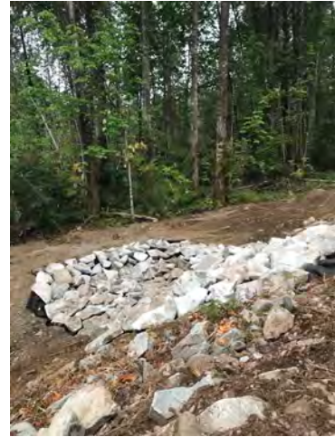
Photo 2: Riprap at Outlet Channel
