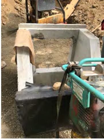
Photo 1: Installation of Concrete Sump
