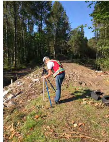
Photo 4: Survey of Flood Box Area
