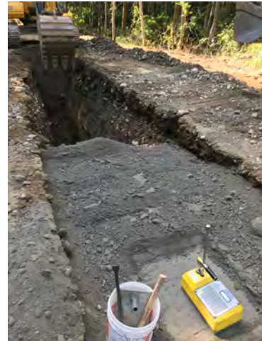
Photo 4: Field Density Testing
