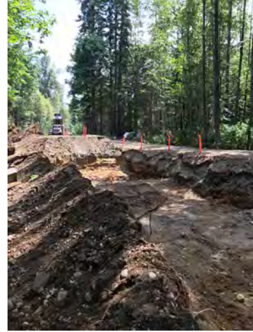
Photo 2: Excavation in Rebuild Section, looking East
