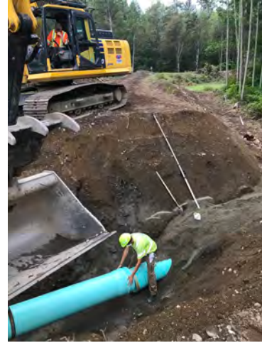
Photo 2: Installation of 450mm PVC
