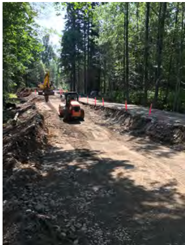
Photo 1: Backfilling and Compaction in Rebuild Section
