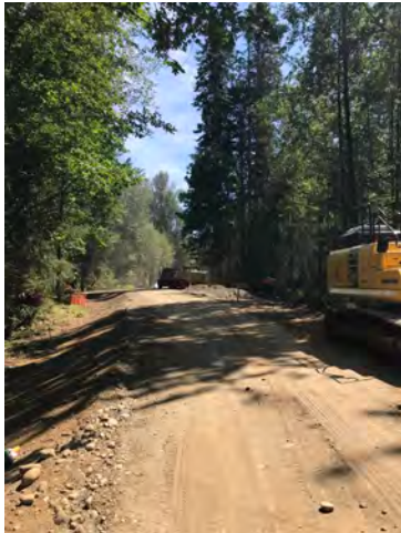
Photo 3: Importing and Stockpiling Till Material
