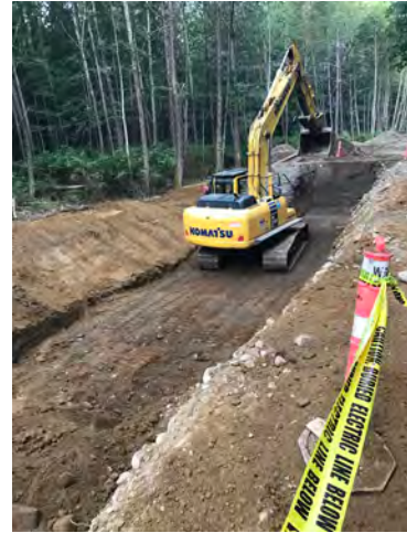
Photo 2: Excavation of Full Rebuild Section
