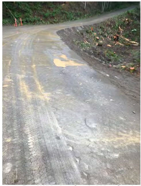
Photo 4: Road Widening, Sta. 0+000 to Sta. 0+020
