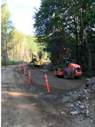
Photo 1: Backfilling and Compaction in Rebuild Section
