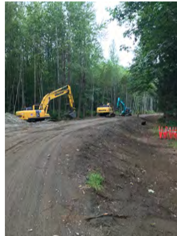
Photo 2: Disturbed Banks to be Hydroseeded
