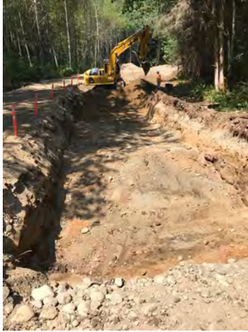
Photo 1: Excavation in Rebuild Section, looking West
