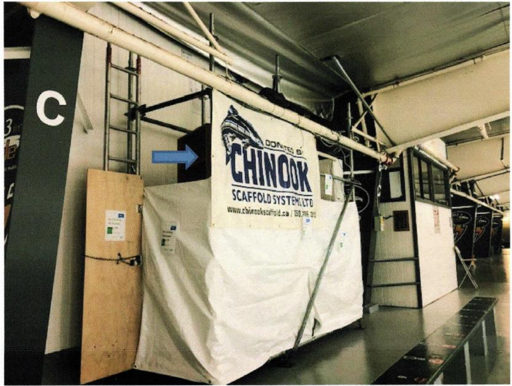
EXHIBIT 3 – Scaffolding for media centre (located on mezzanine level near announcer's booth).
