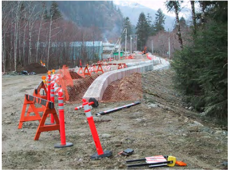
Figure 7: Flood Wall Construction Along North Maquinna Drive
