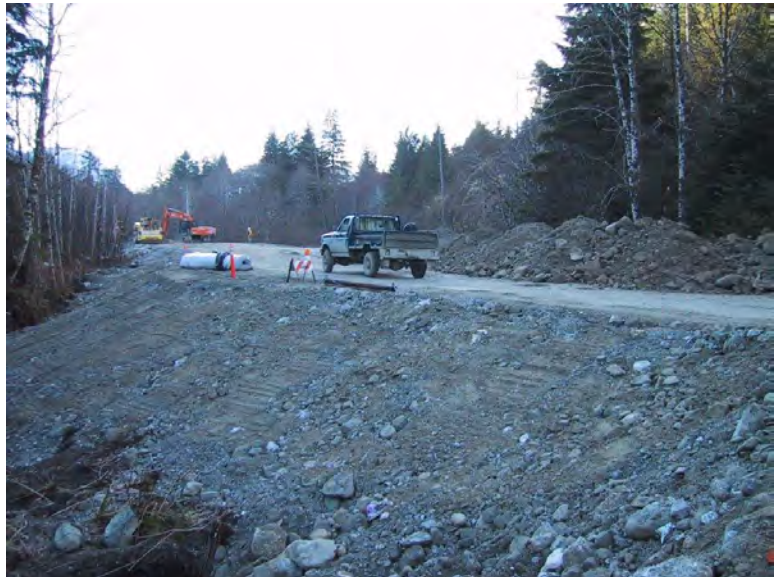
Figure 8: Construction of the Cook Street Dike
