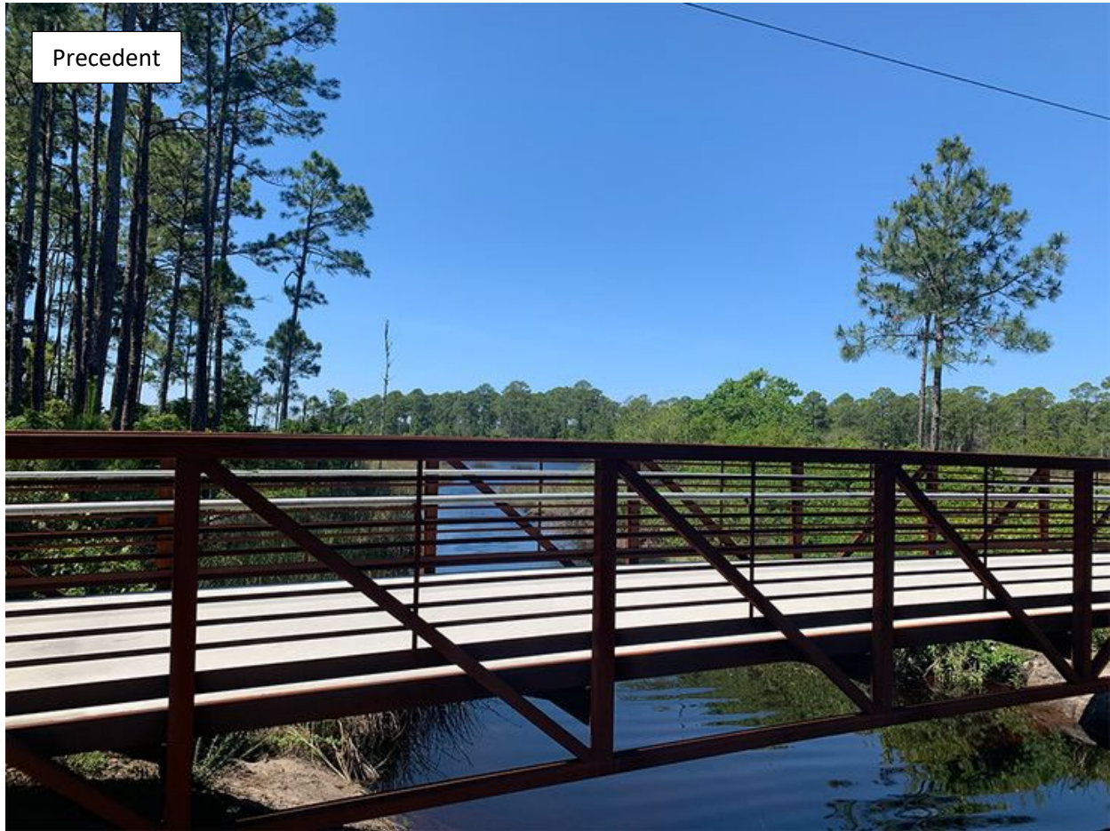
An example of an active transportation bridge.
