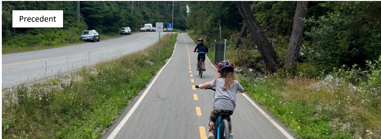
The Tofino to Ucluelet Multi-Use Path weaves in and out of the forest in Pacific Rim National Park, providing separation from vehicle traffic while preserving the area's natural character.
