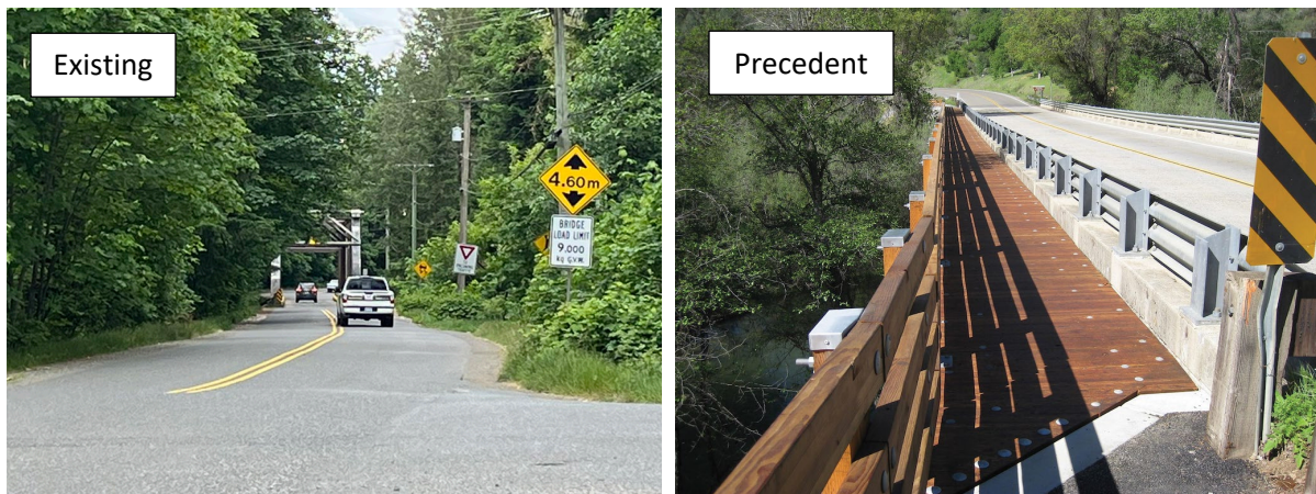
Existing Regent Road Bridge (Left) and an example of a separated pathway retrofitted to the side of a bridge (Right) Photo Sources: Bunt & Associates Engineering Ltd. (Left), US FHWA "Small Town and Rural Design Guide" (Right, 2016)
