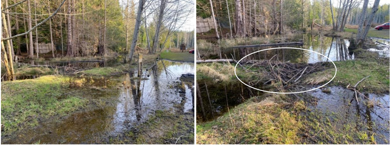
Figure 32. Left: The beaver dam is causing flooding of the parking lot. Right: Close up of the beaver dam, beaver have repaired a breach in this dam, evidenced by the darker area of fresh soil covered in sticks (circled in white) March 6 2025.
