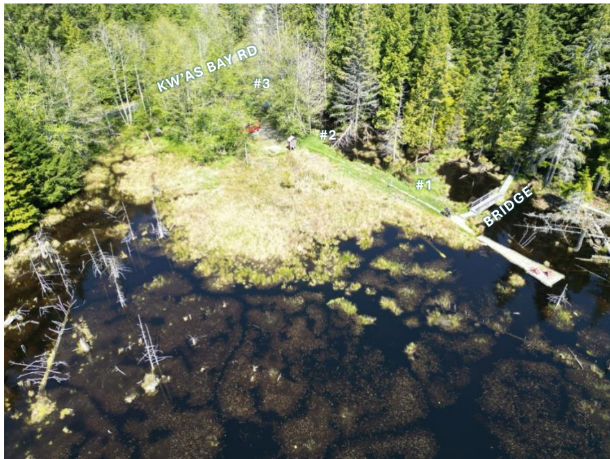
Figure 49. Aerial photo showing the bridge and beaver dams (numbered #1,2,3), and Kw'as Bay Rd. May 1, 2024.
