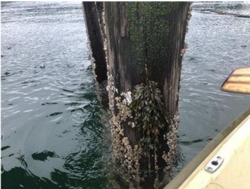
Photo 26 – Fender Pile 14A
