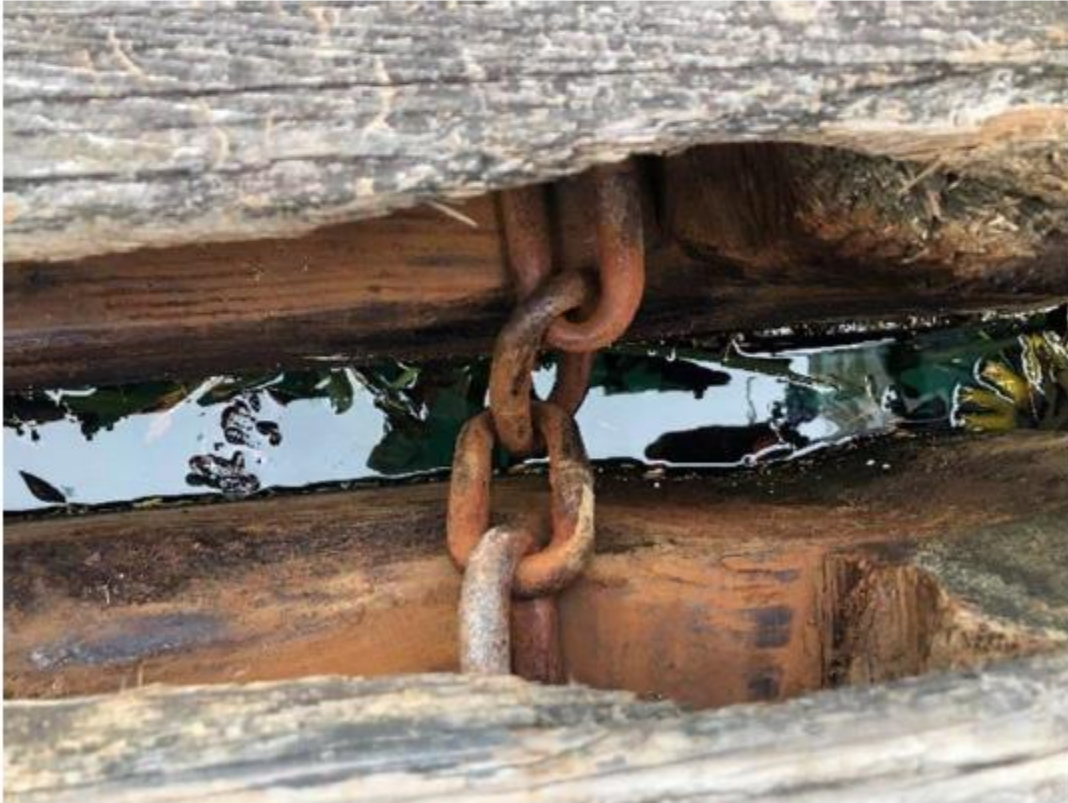
Photo 40 – Chain Connection to Float B
