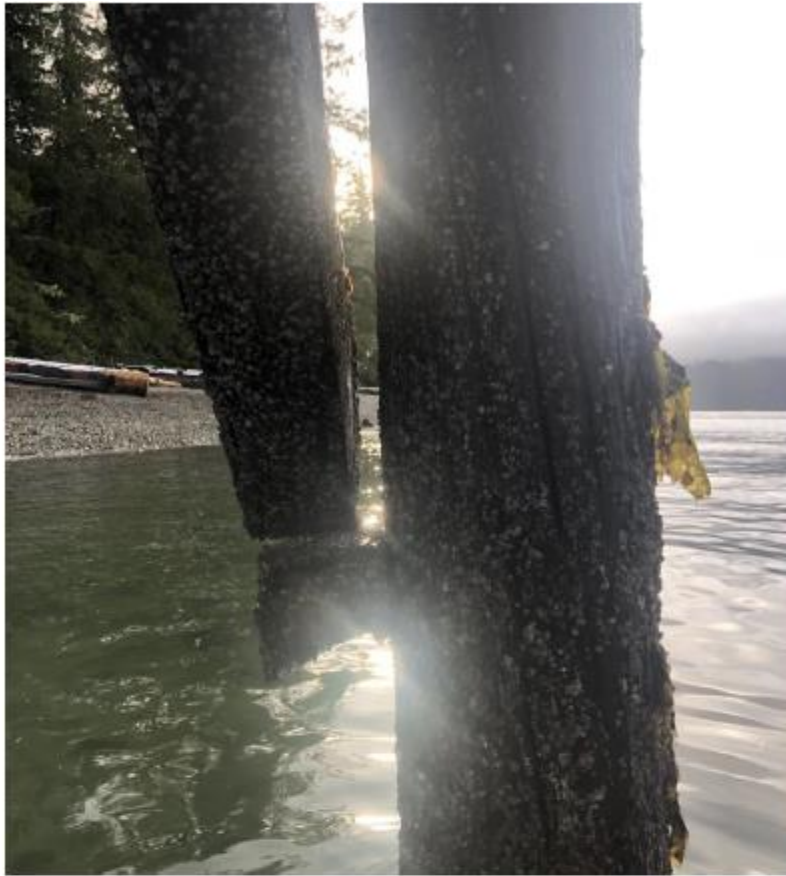
Photo 29 – Cross Bracing at Bent 8
