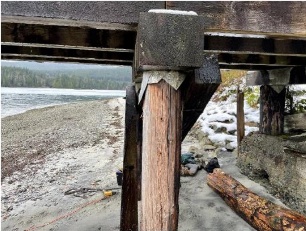
Photo 13 – Typical Timber Pile Cap End Grain
