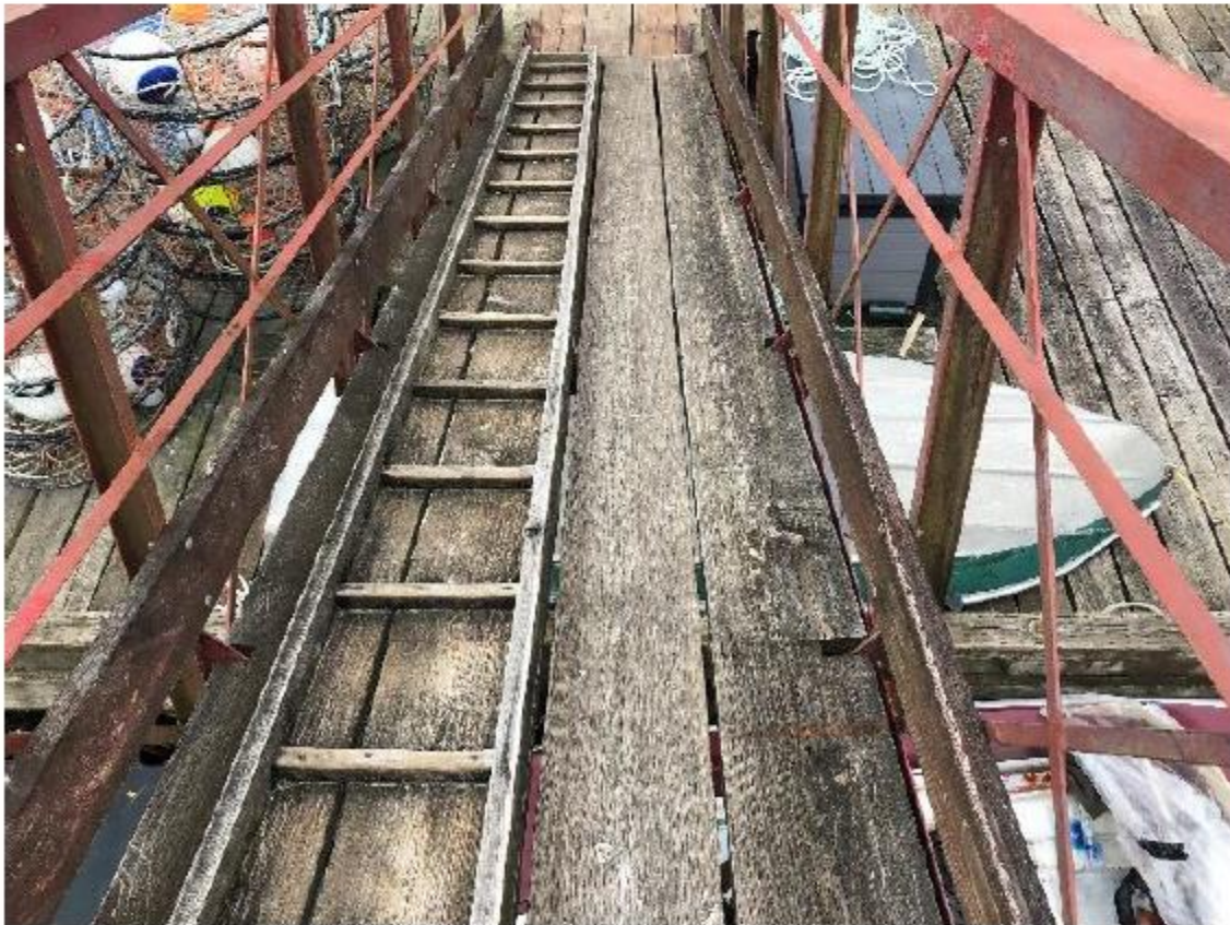
Photo 34 – Gangway Timber Deck Planks
