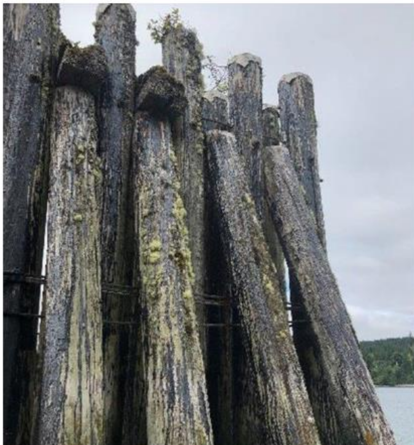
Photo 44 – North Mooring Dolphin
