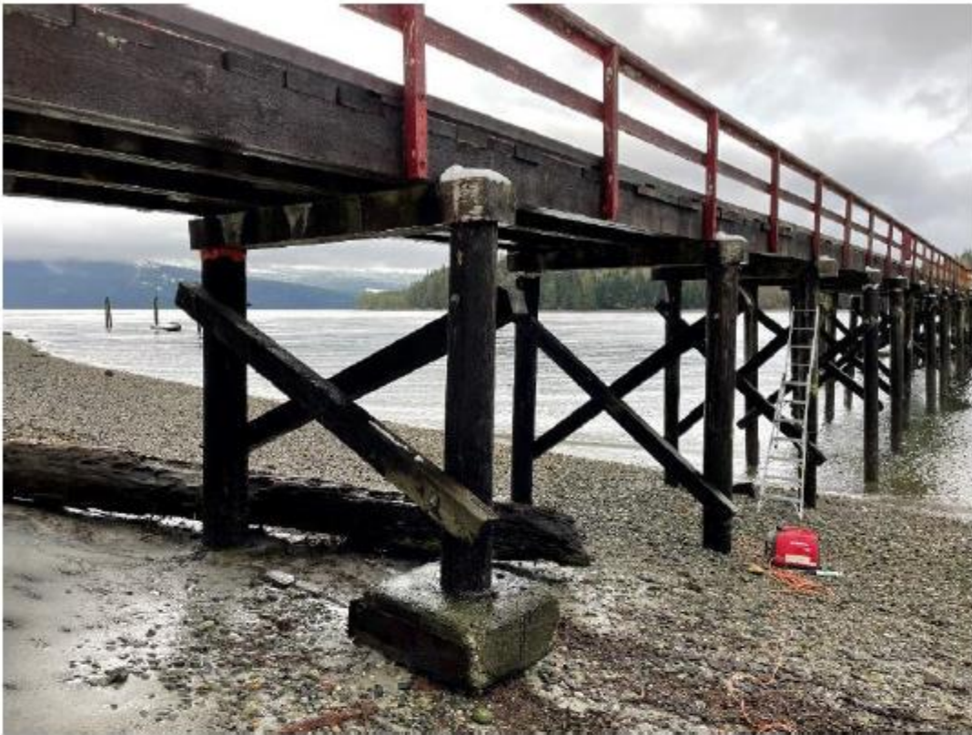
Photo 17 – Pile 4B concrete footing
