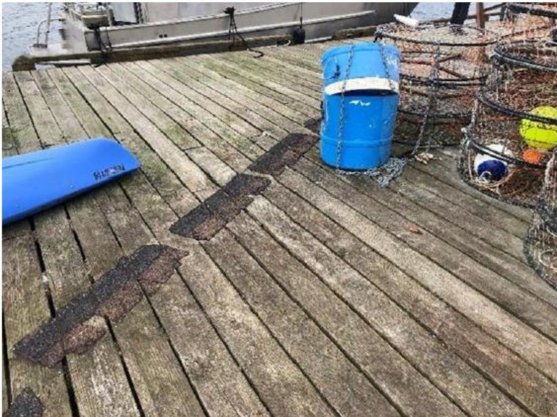
Photo 36 – General view of Float A
