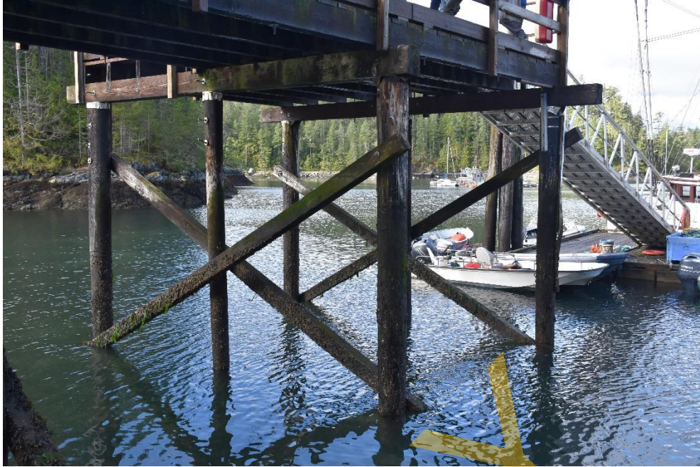
Photo 19 - General view of Cross Bracing
