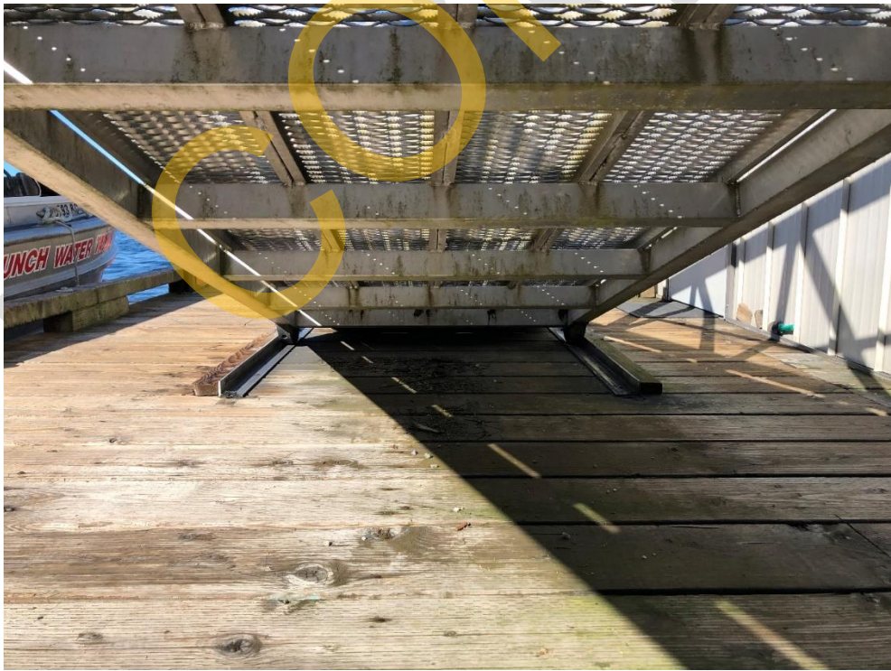
Photo 40 - Gangway slider plate and rollers
