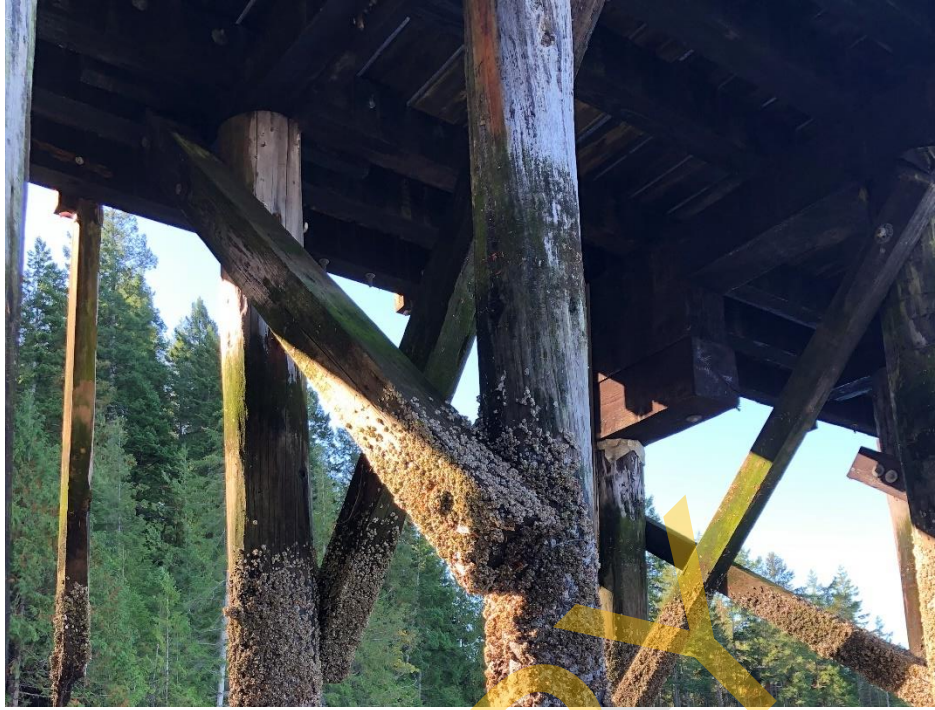
Photo 31 - General condition of the Cross Bracing
