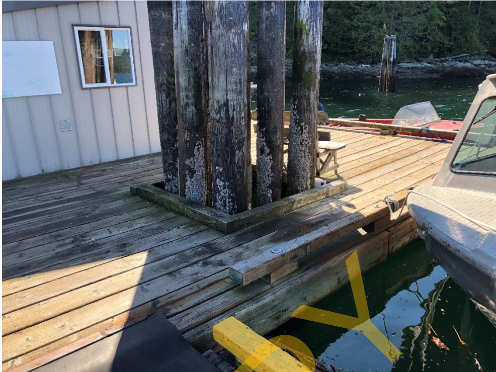
Photo 53 - West end Mooring Piles
