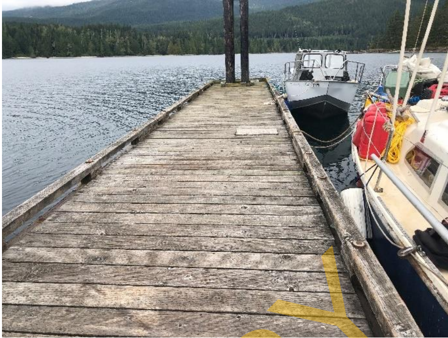
Photo 37 – General view of Float B
