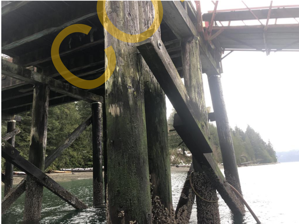
Photo 30 – Cross Bracing at Bent 15
