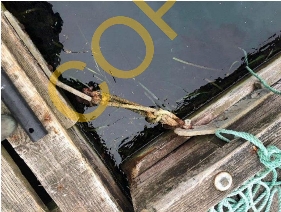
Photo 38 – Rope connection to Float B
