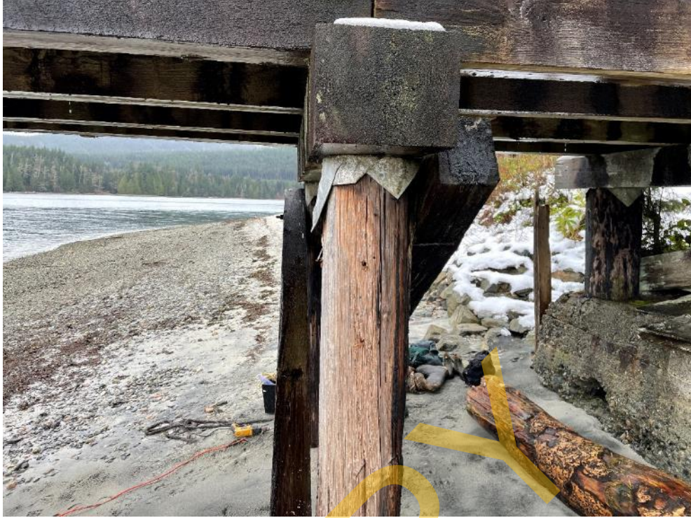
Photo 13 – Typical Timber Pile Cap End Grain
