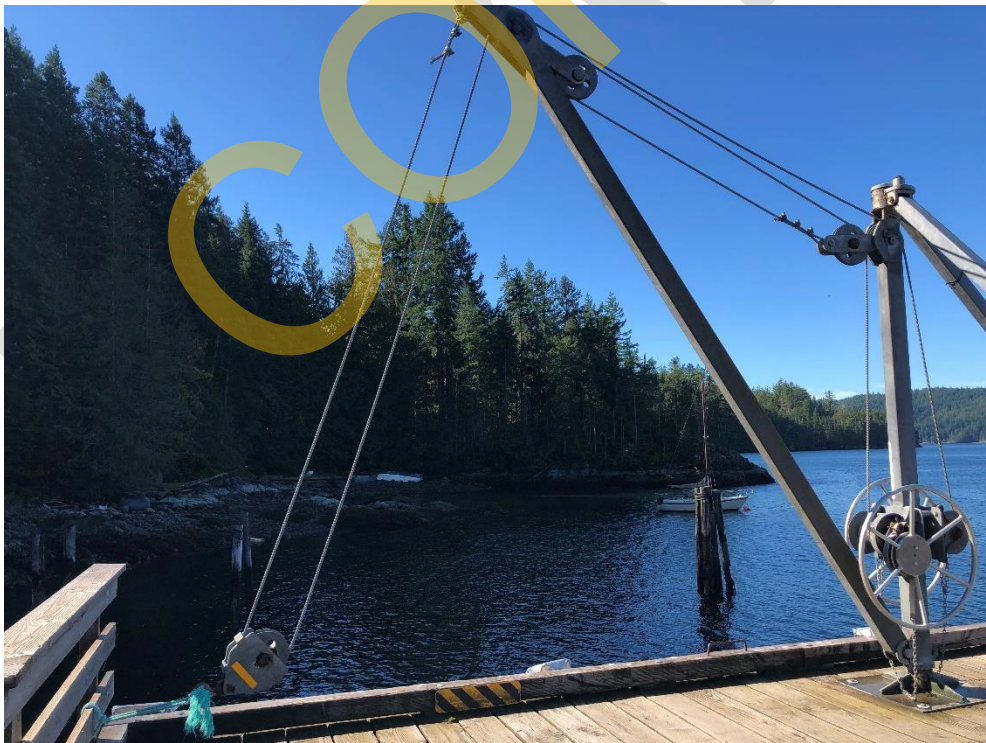
Photo 36 - Derrick Loading Crane
