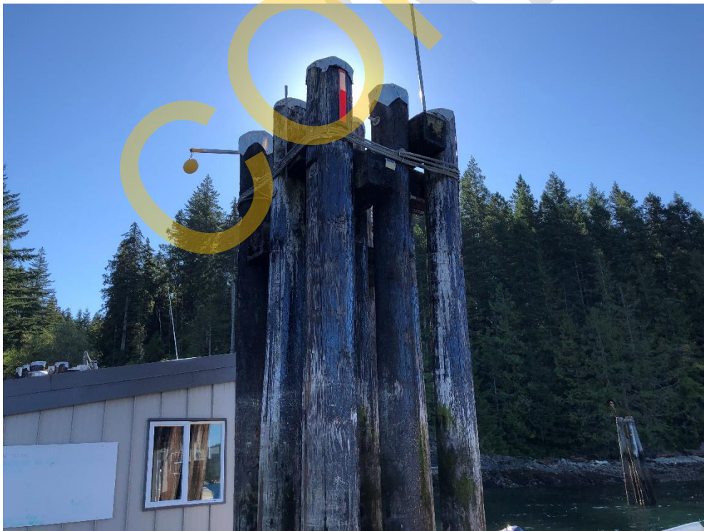
Photo 54 - West end Mooring Piles
