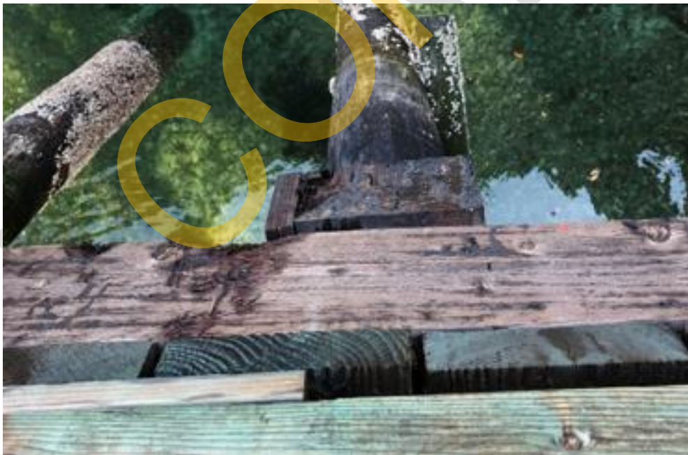
Photo 22 - Pile cap at Bent 14
