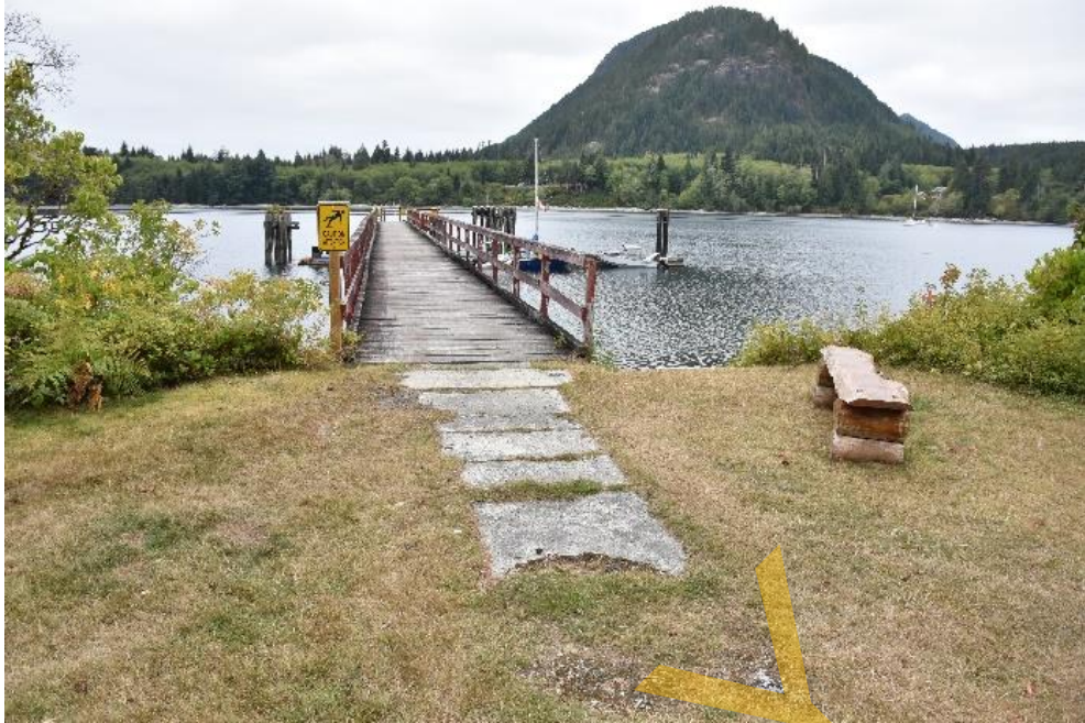
Photo 1 – Pier Approach Area
