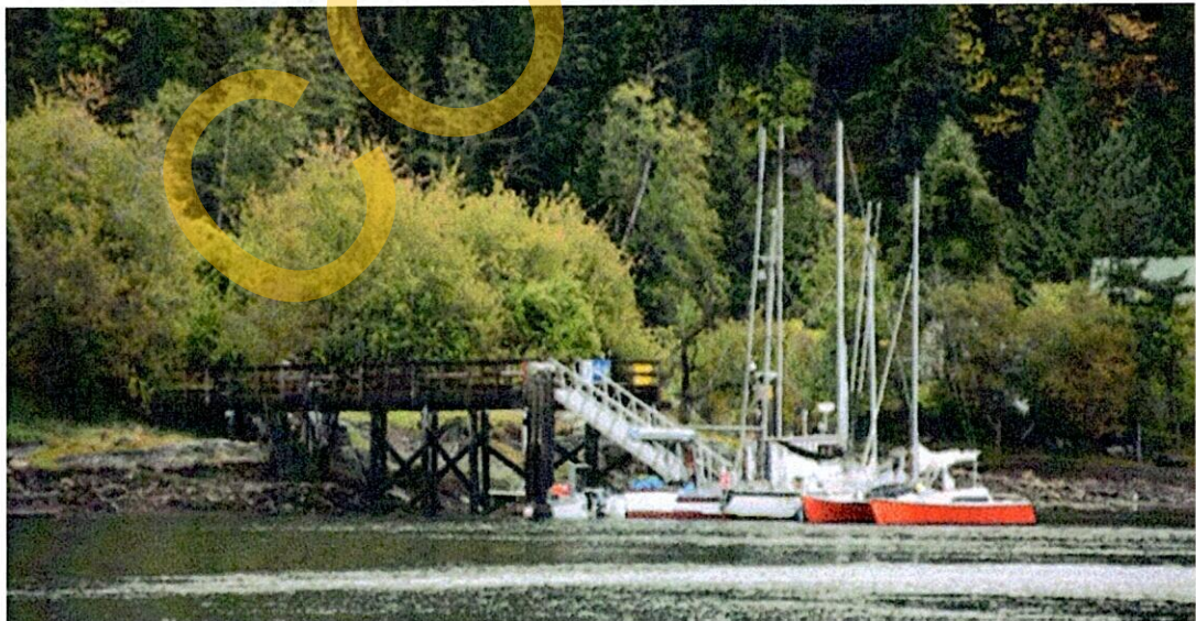
Figure 3 – Owen Bay wharf (McElhanney Engineering Ltd. 2019)
