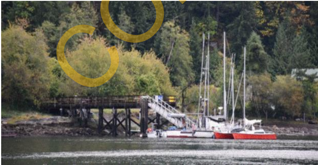
Figure 3 – Owen Bay wharf (McElhanney Engineering Ltd. 2019)
