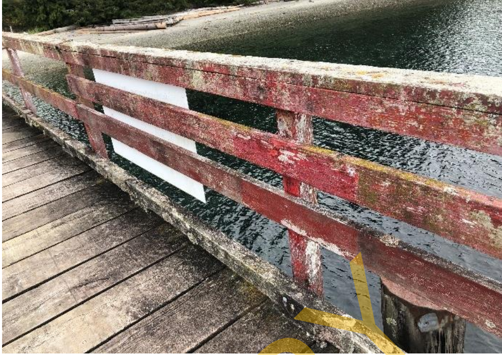
Photo 3 – Pier Structure Handrails
