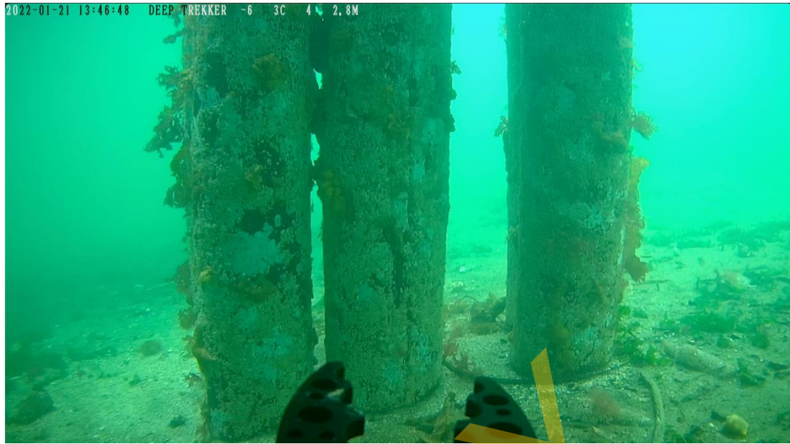
Photo 31 - North Mooring Piles
