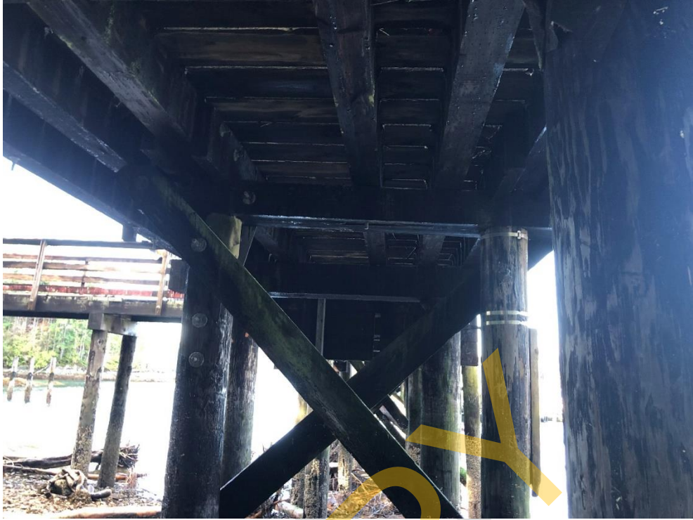
Photo 13 - Pile cap at Bent 4
