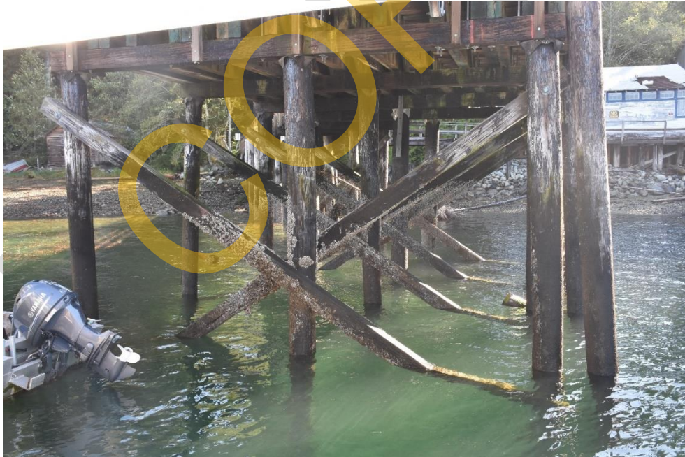
Photo 32 - General view of Cross Bracing
