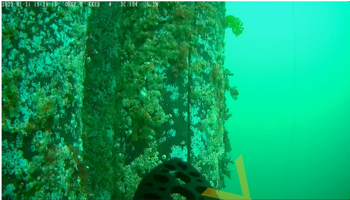
Photo 57 - West end Mooring Piles
