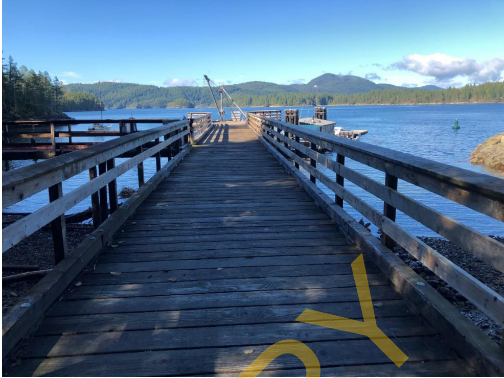
Photo 3 - Wharf Structure Topsides
