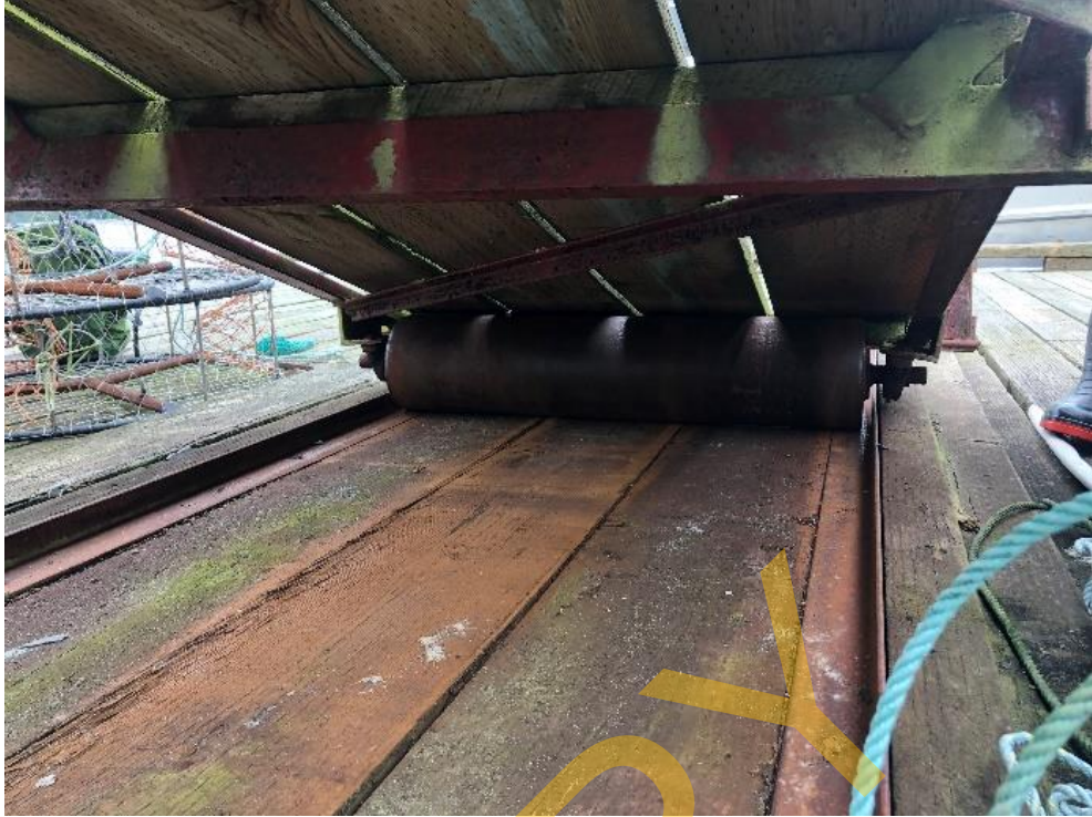
Photo 33 – Gangway Timber Slider Plate and Roller
