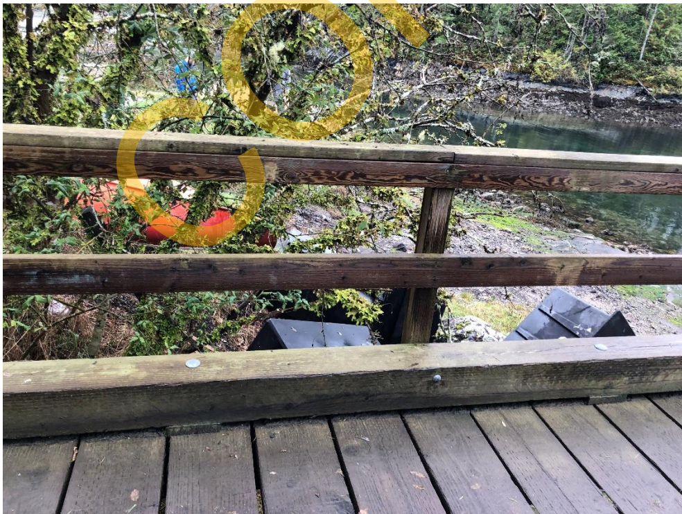
Photo 4 - General View of the Handrails
