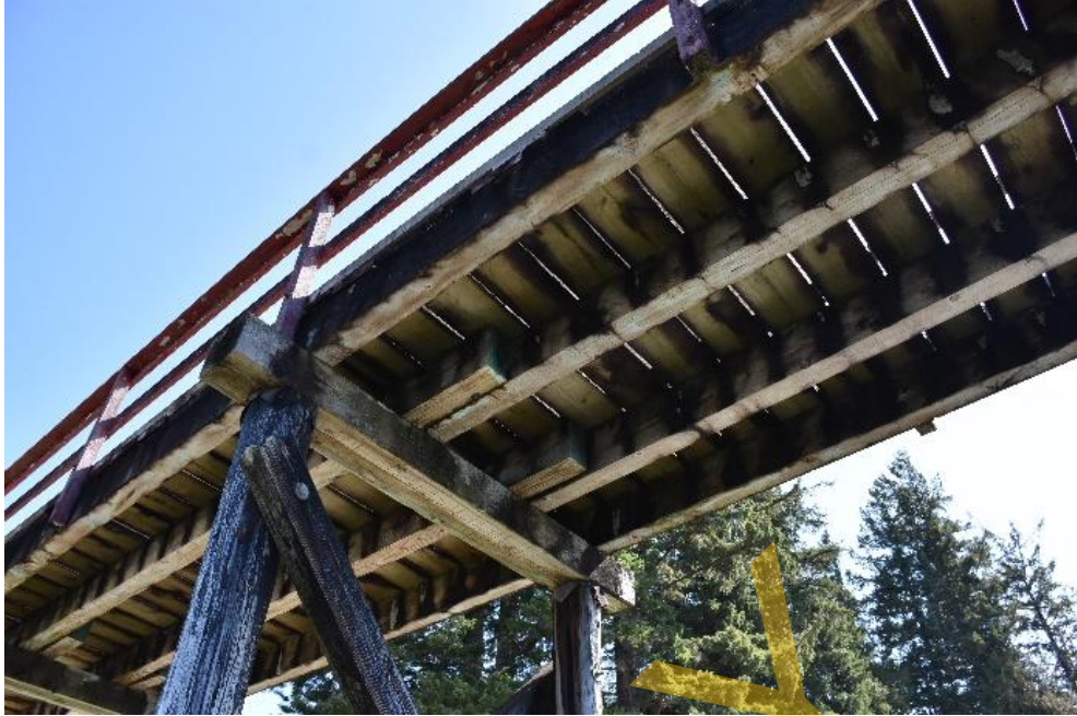
Photo 11 – Typical View of Timber Stringers
