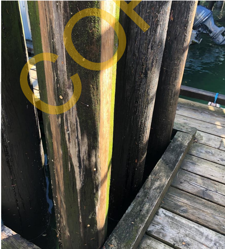
Photo 52 - East end Mooring Piles
