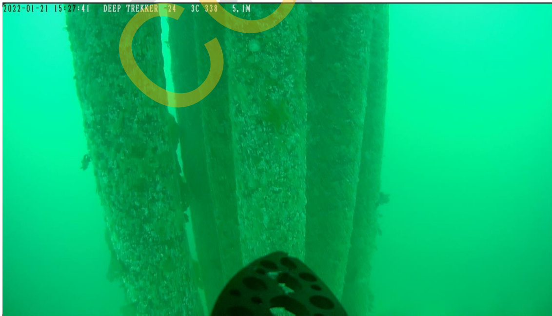
Photo 56 - West end Mooring Piles
