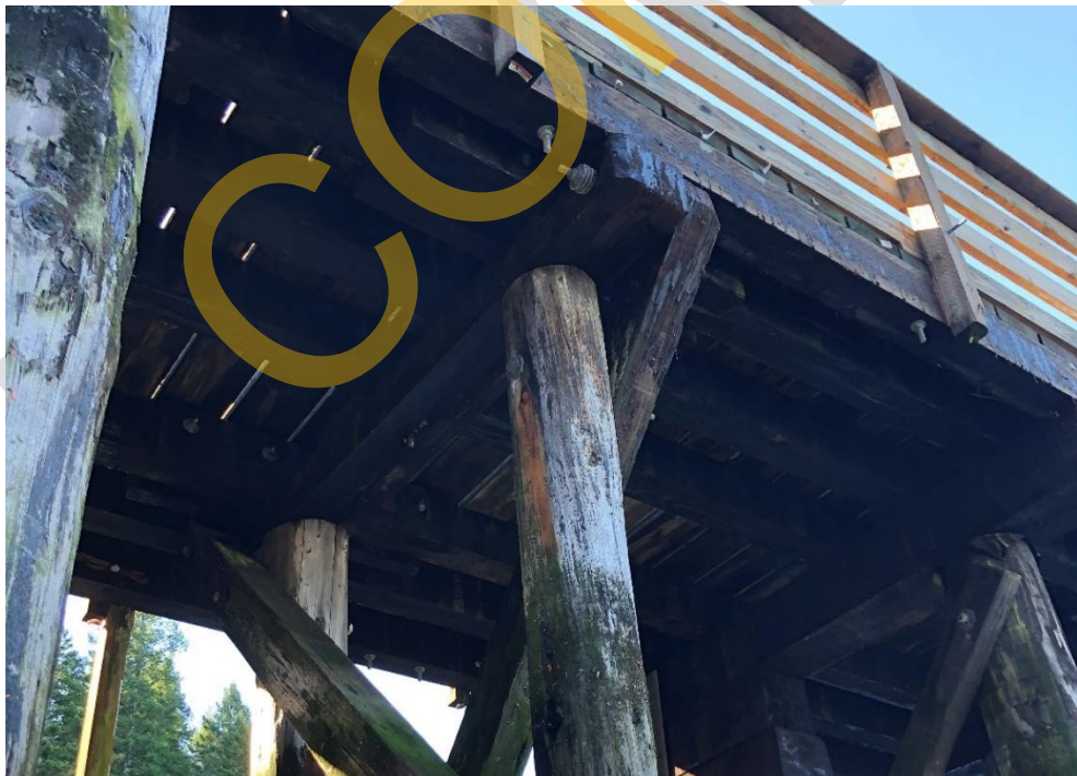
Photo 20 - Pile cap at Bent 12
