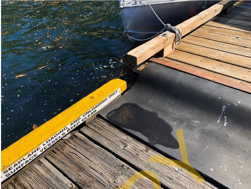
Photo 61 - Transition from the Main Float to the Seaplane Float
