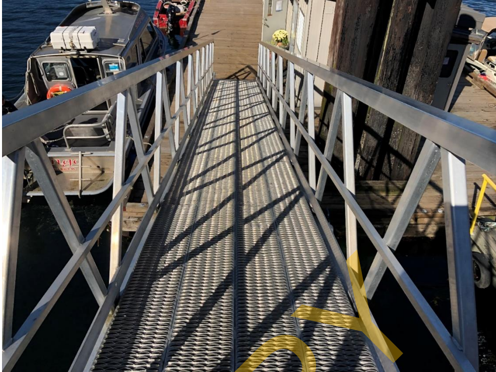
Photo 39 - General View of Aluminum Gangway
