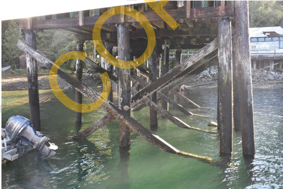
Photo 32 - General view of Cross Bracing
