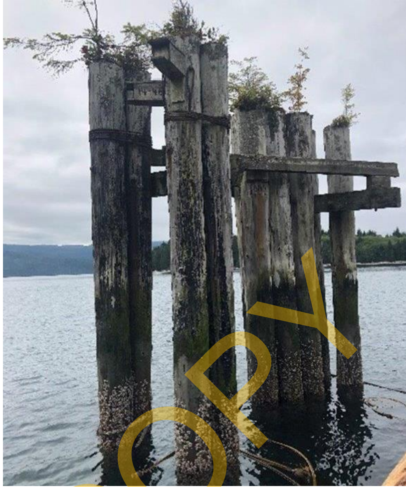
Photo 45 – South Mooring Dolphin
