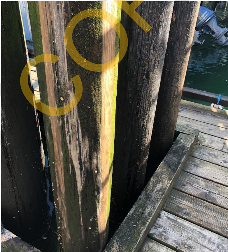
Photo 52 - East end Mooring Piles
