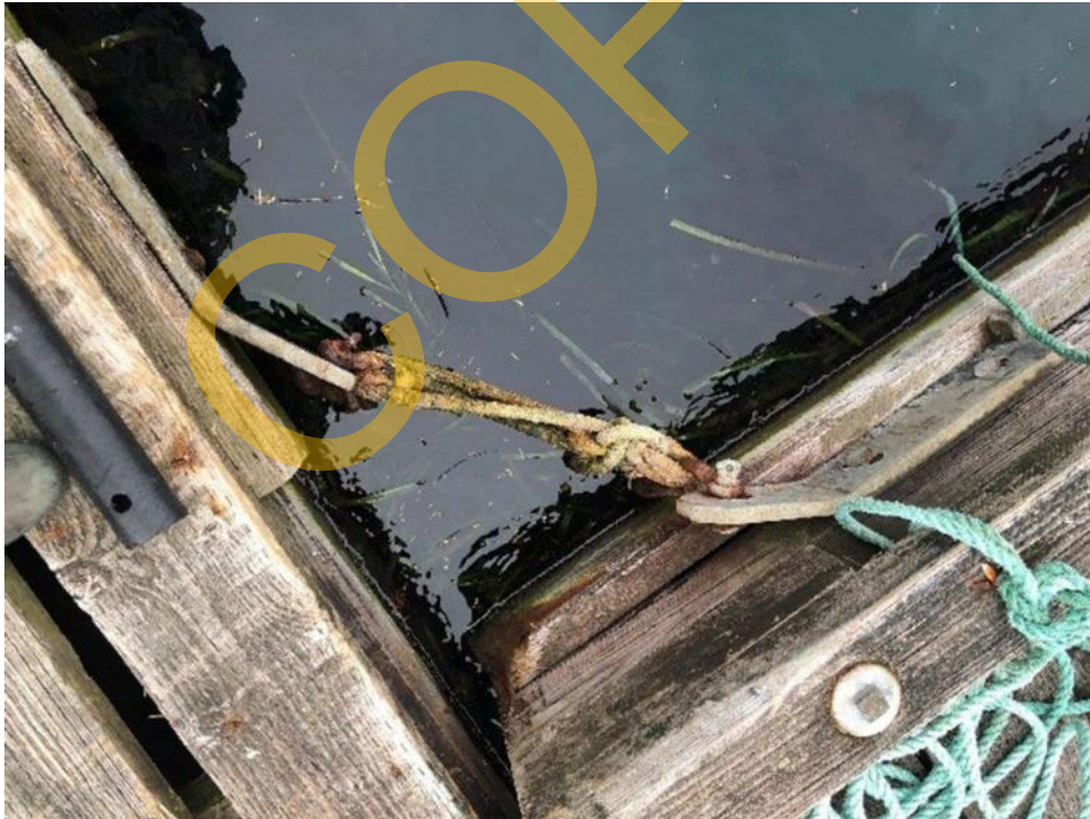
Photo 38 – Rope connection to Float B
