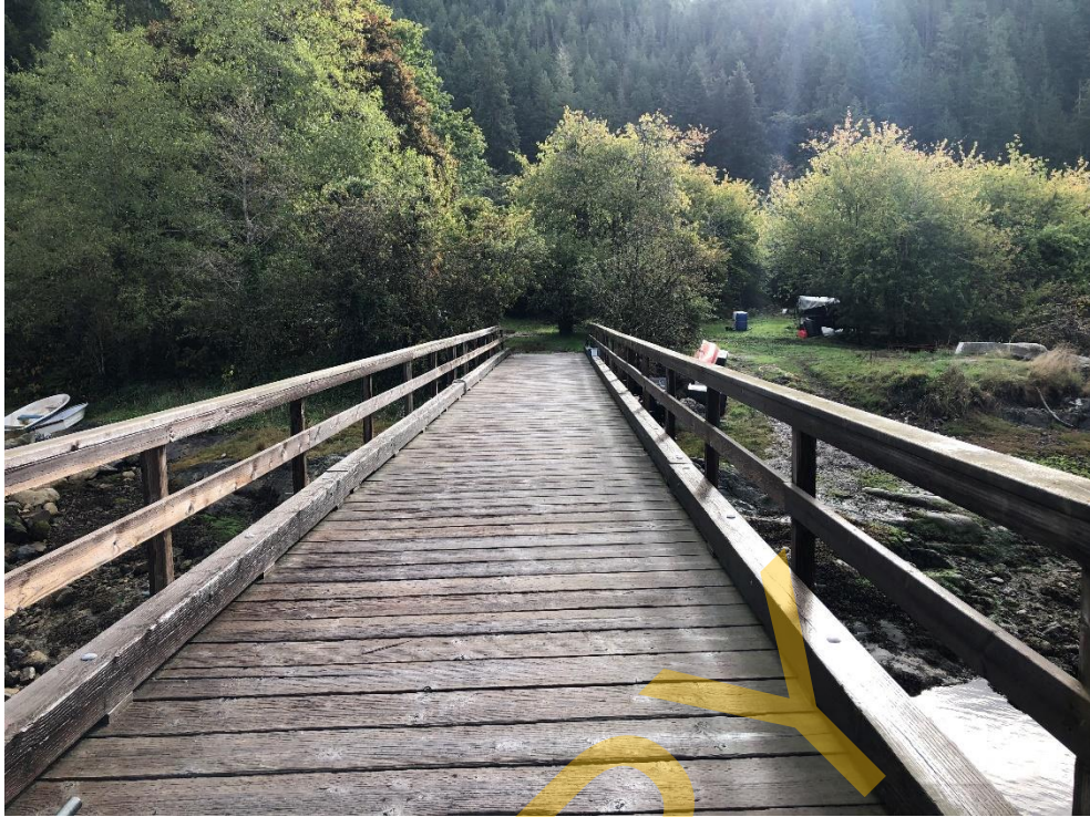
Photo 3 - Topsides of the Wharf Structure
