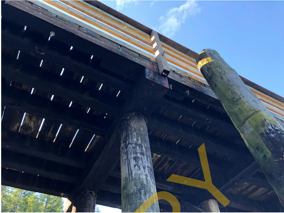
Photo 19 - Pile cap at Bent 11
