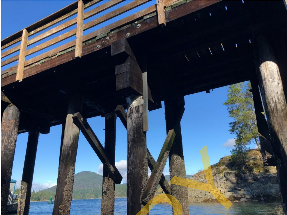
Photo 21 - Pile cap at Bent 13 with corbels
