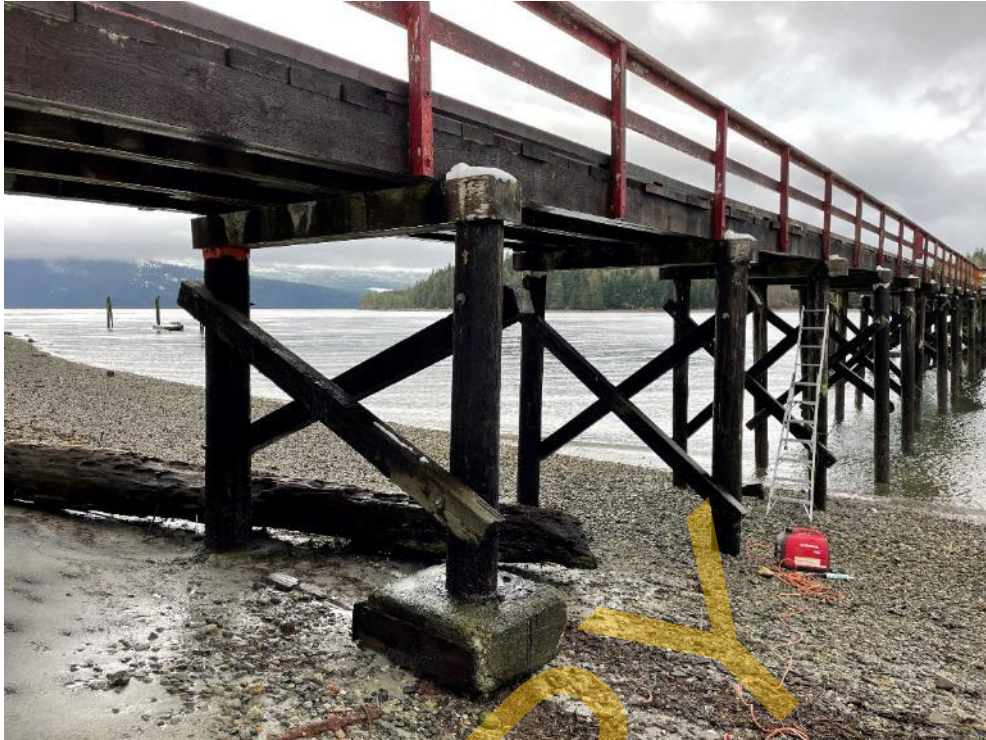
Photo 17 – Pile 4B concrete footing
