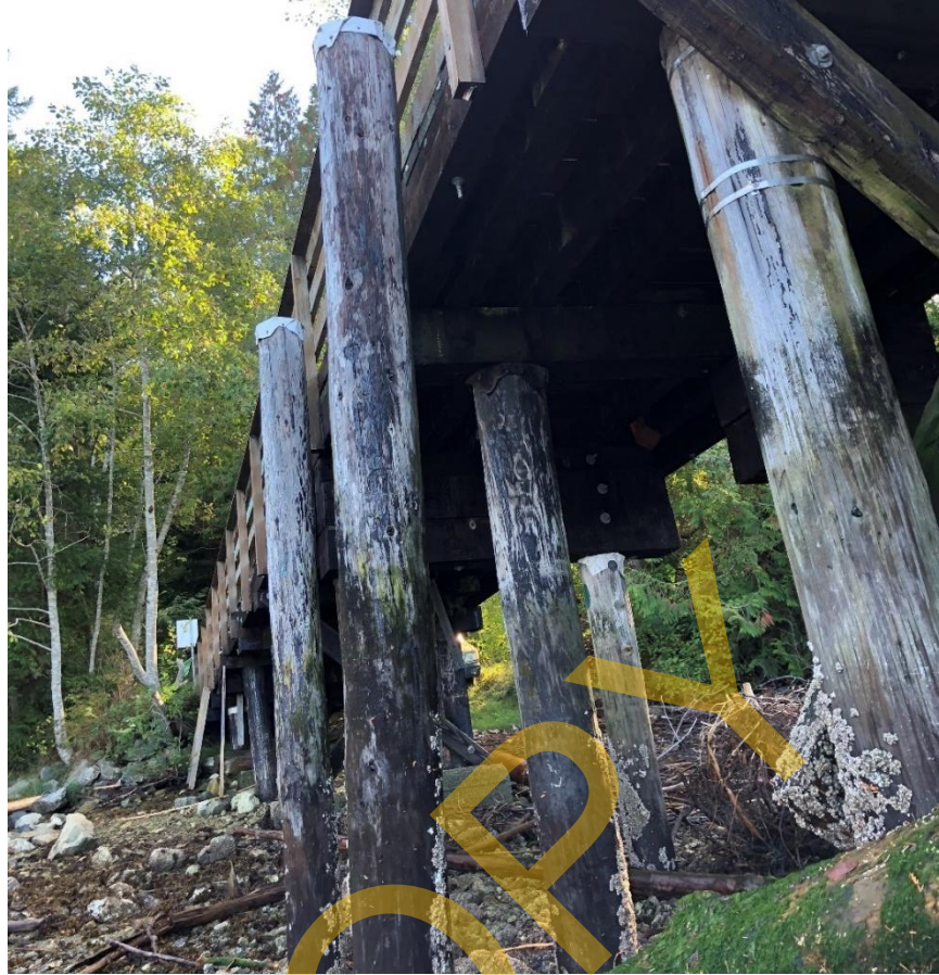
Photo 29 - North end fender piles
