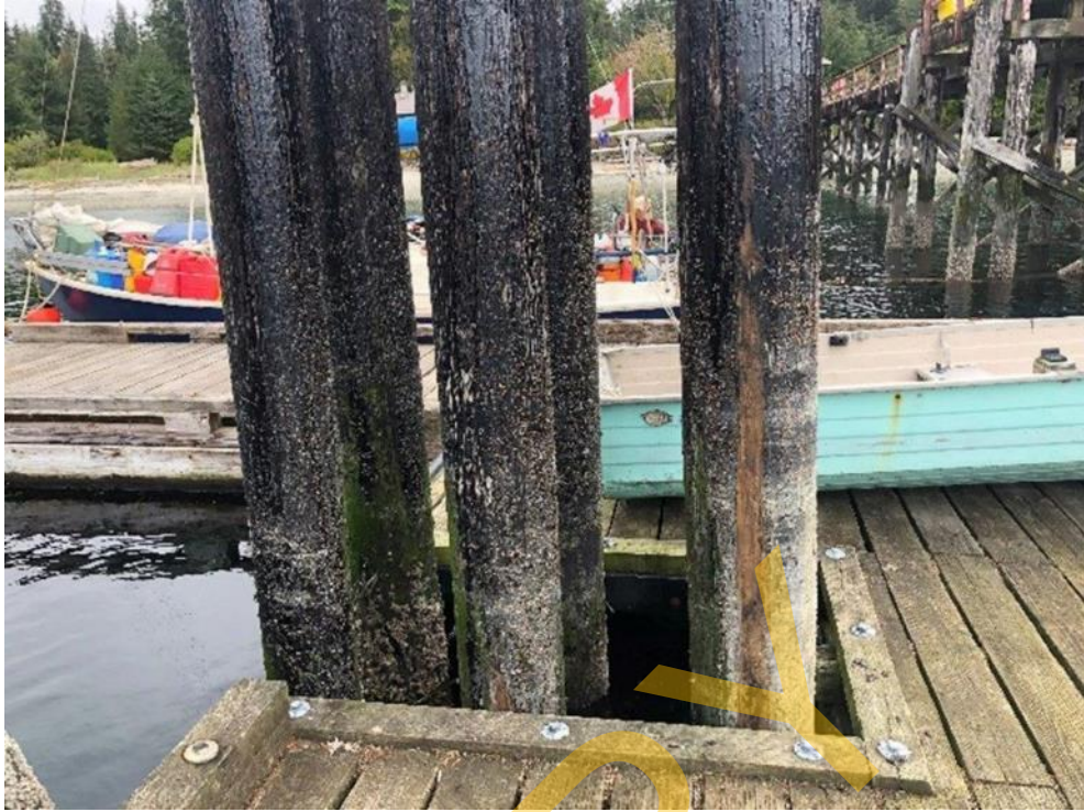
Photo 43 – Float A North Mooring Piles
