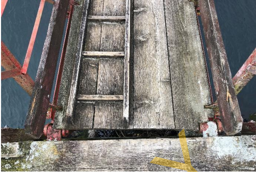
Photo 31 – Gangway Upper Hinge Connection
