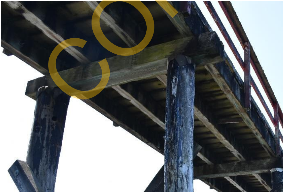
Photo 14 – Timber Pile Cap at Bent 12
