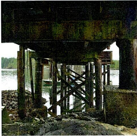
Figure 2 – Typical configuration of wharf piles and cross-bracing.
