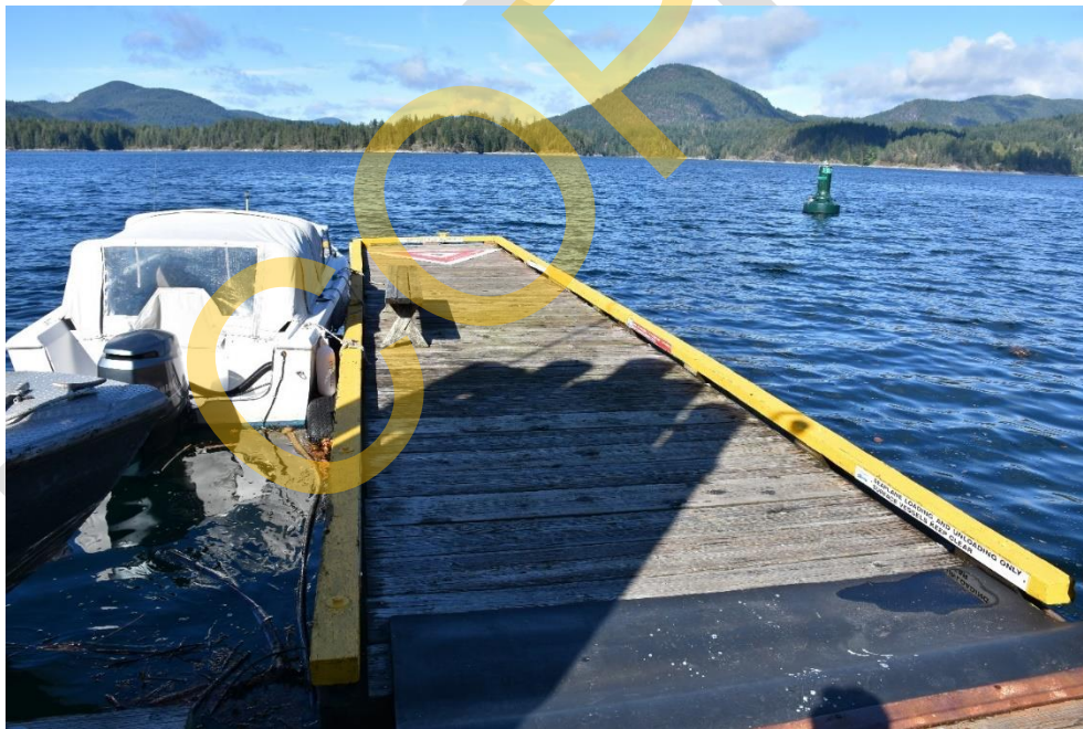
Photo 58 - General view of the Seaplane Float
