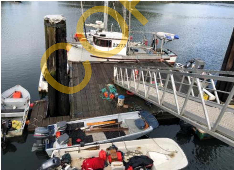
Photo 24 - General View of the float
