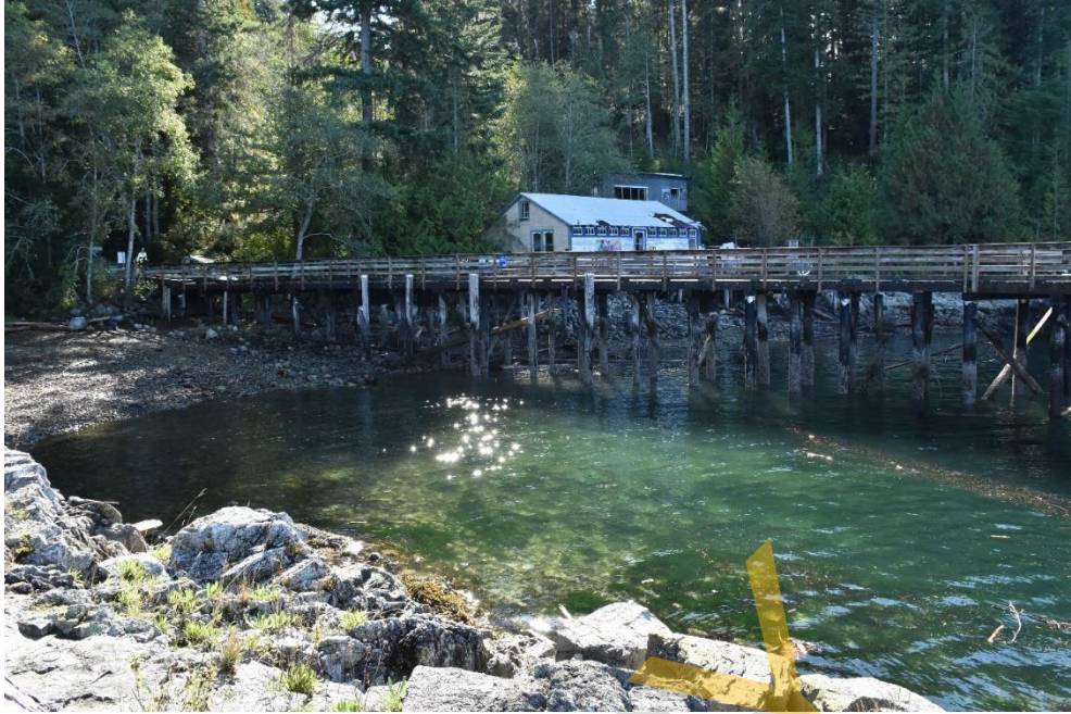
Photo 9 - General View facing south of the timber pile caps
