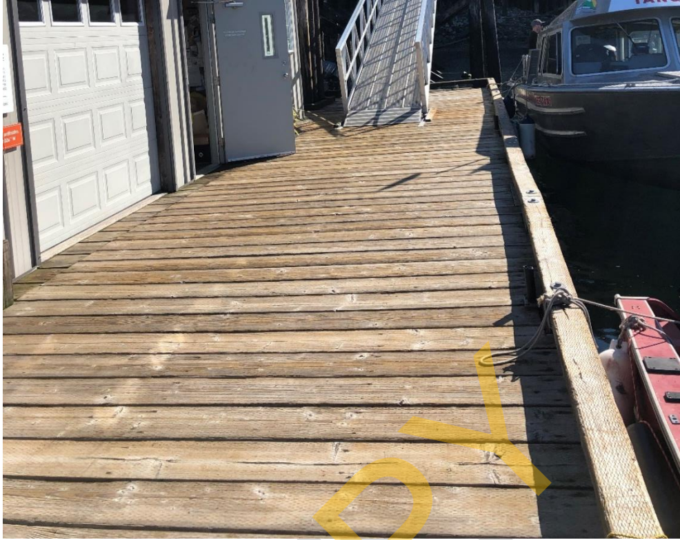
Photo 43 - Typical condition of the Main Float deck
