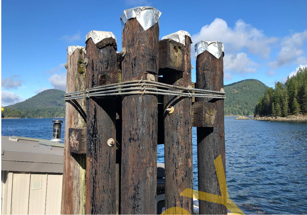
Photo 51 - East end Mooring Piles
