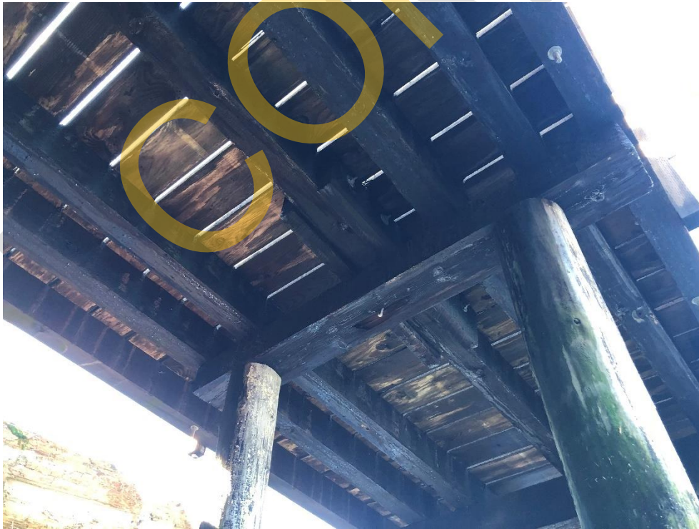
Photo 8 - Typical View of Timber Stringers
