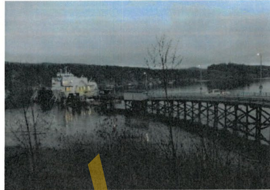
Existing Ferry Berth
