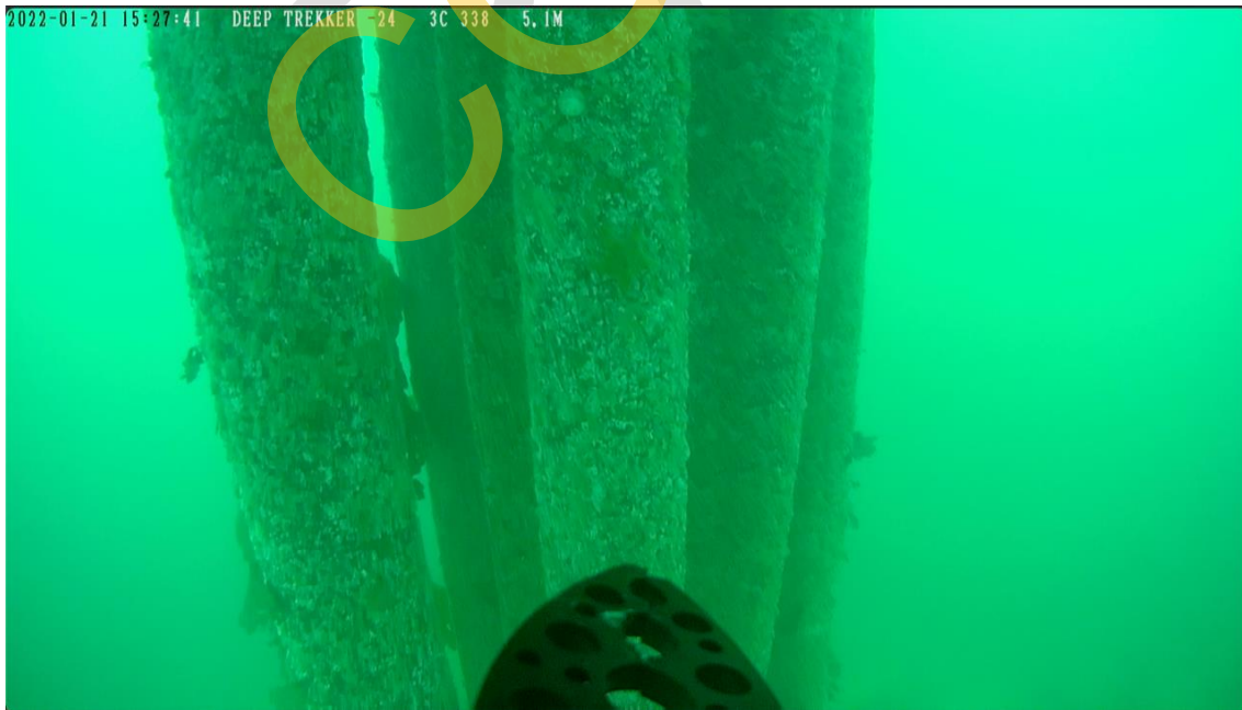
Photo 56 - West end Mooring Piles
