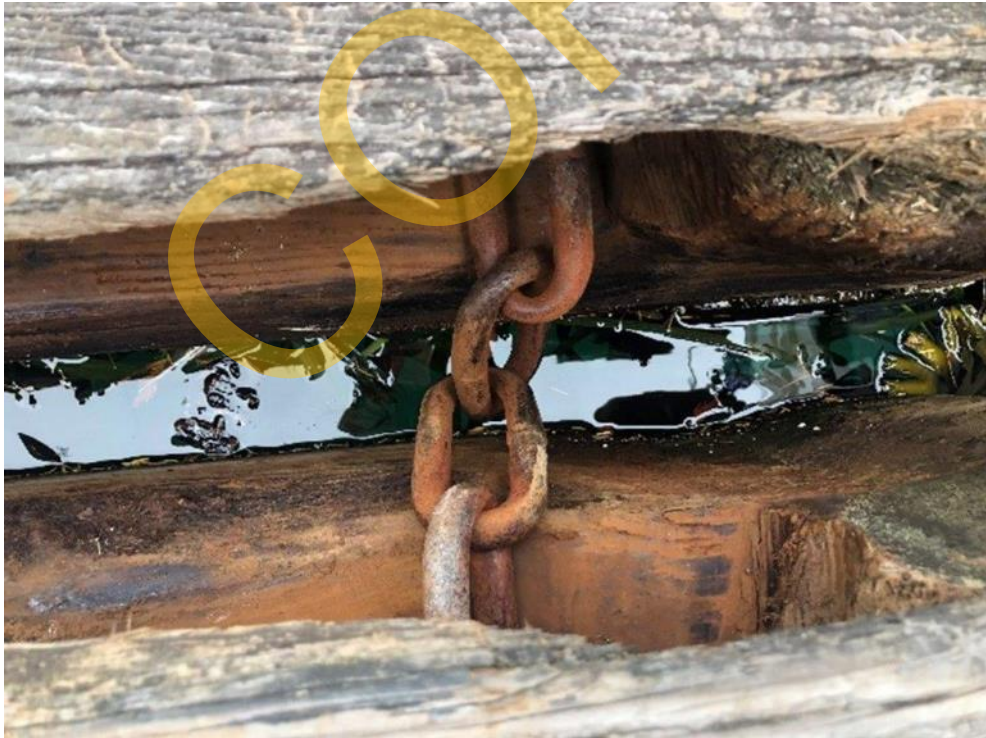
Photo 40 – Chain Connection to Float B
