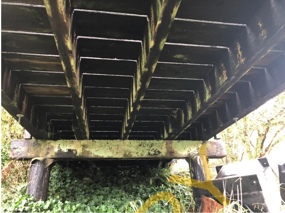
Photo 5 - General view of the Stringers
