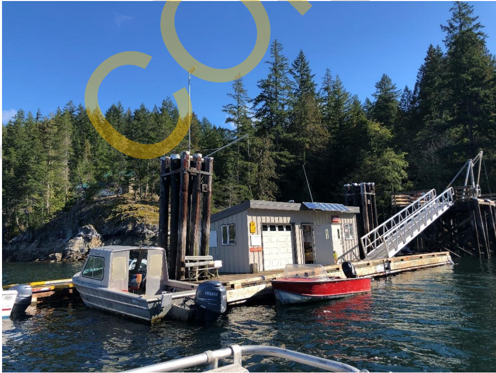
Photo 42 - General View of the Main Float
