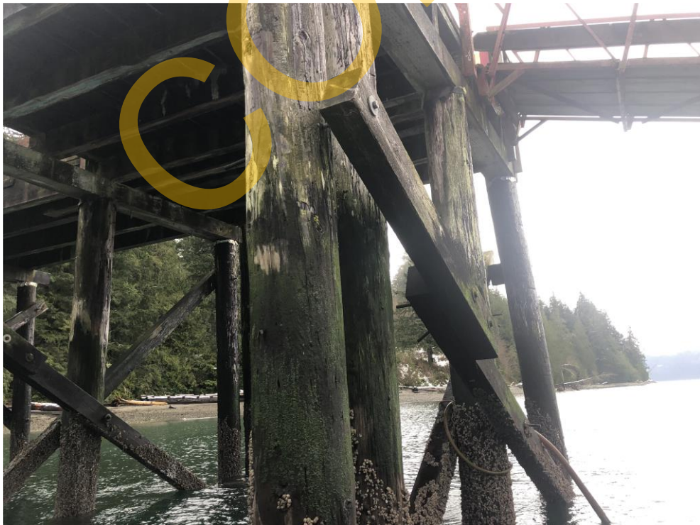
Photo 30 – Cross Bracing at Bent 15
