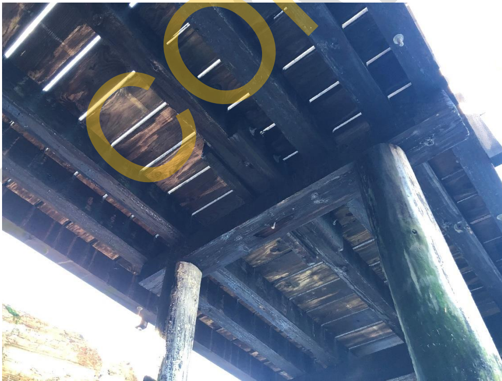
Photo 8 - Typical View of Timber Stringers
