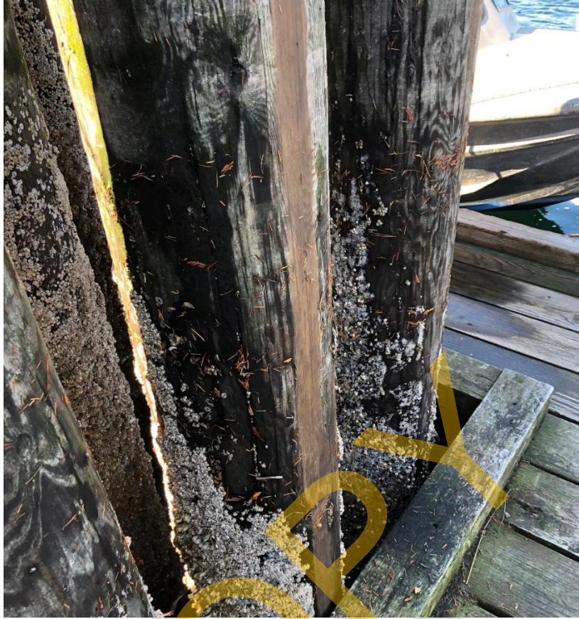
Photo 55 - West end Mooring Piles – up to 10% CSL
