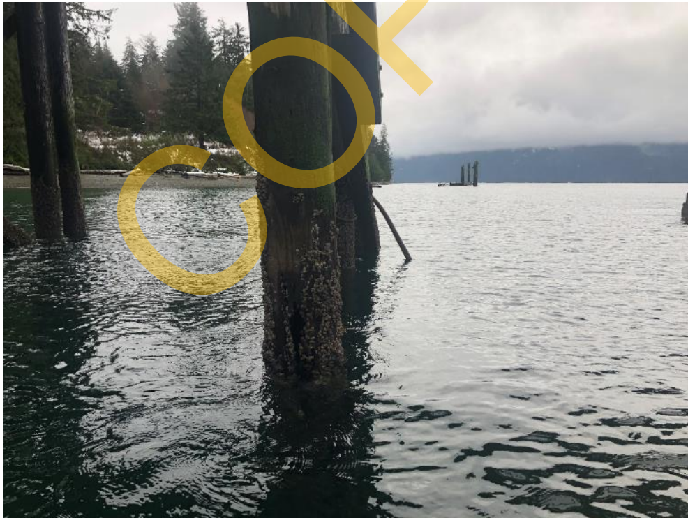
Photo 28 – Fender Pile 15C
