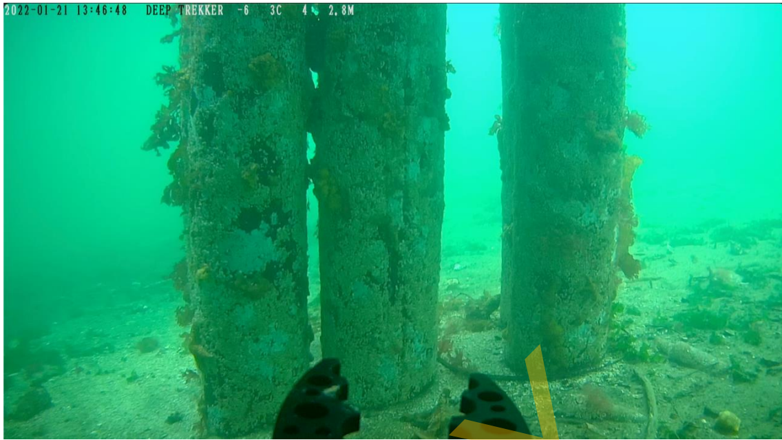
Photo 31 - North Mooring Piles
