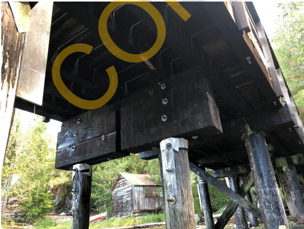
Photo 14 - Pile cap at Bent 6 and corbels
