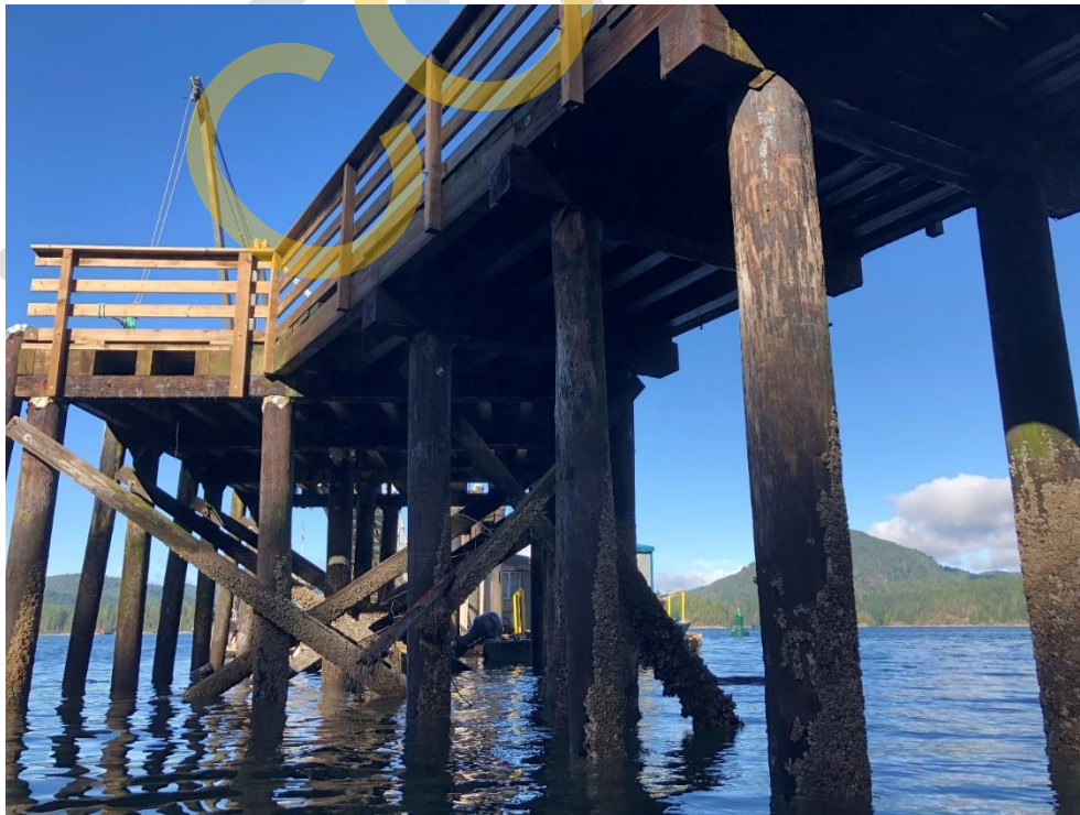
Photo 34 - Log resting on the Cross Bracing
