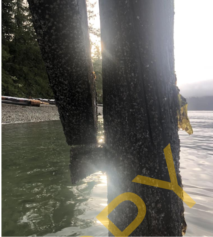
Photo 29 – Cross Bracing at Bent 8
