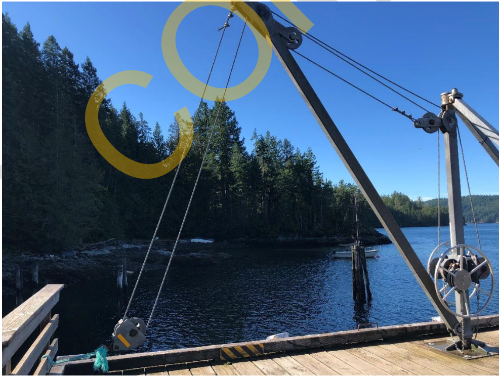
Photo 36 - Derrick Loading Crane
