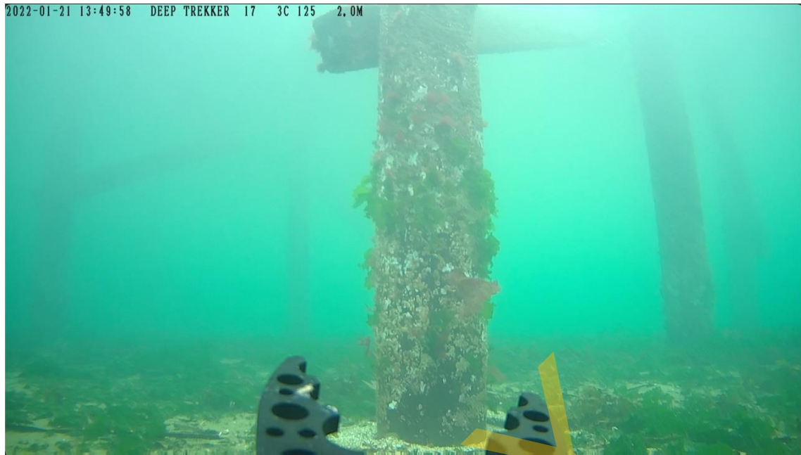
Photo 15 - Typical condition of underwater piles
