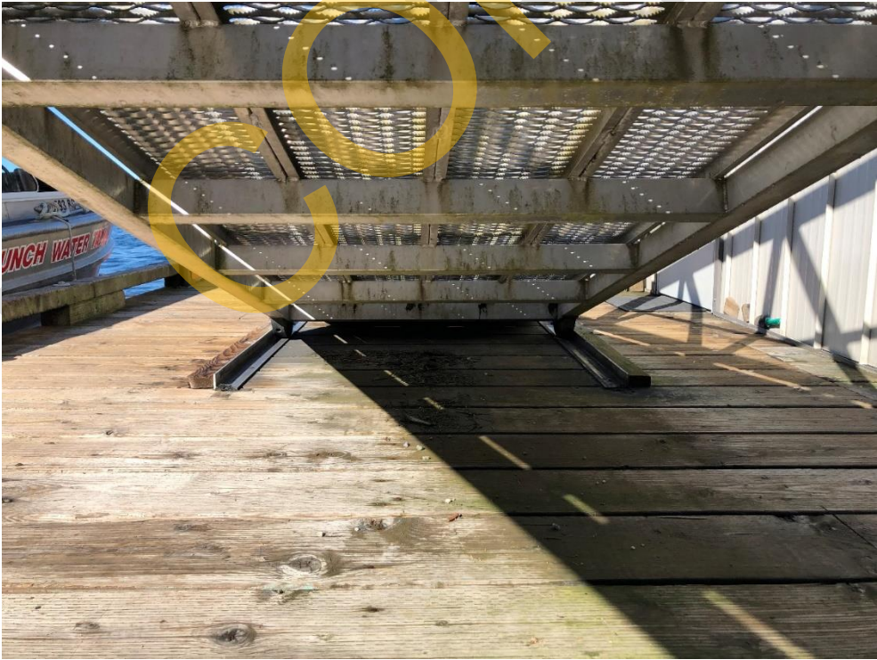
Photo 40 - Gangway slider plate and rollers
