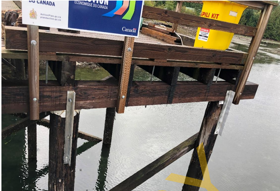
Photo 13 - Through bolts in the Pile Cap at Bent 9
