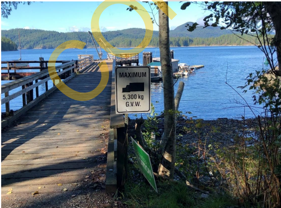
Photo 2 - Load rating sign
