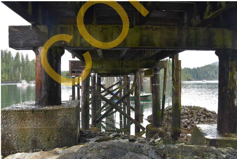
Photo 6 - General view of the Pile Cap Bents
