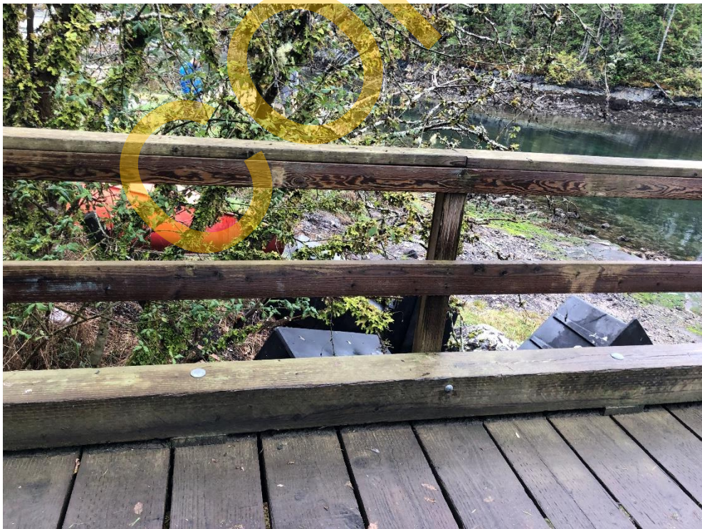
Photo 4 - General View of the Handrails
