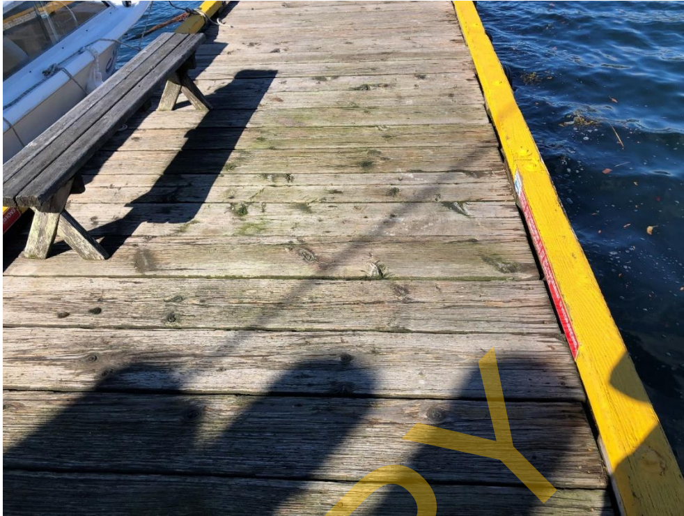
Photo 59 - Typical condition of the Seaplane Float deck
