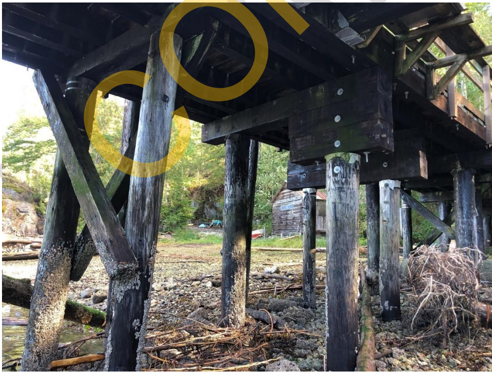
Photo 16 - Pile cap at Bent 7 and corbels
