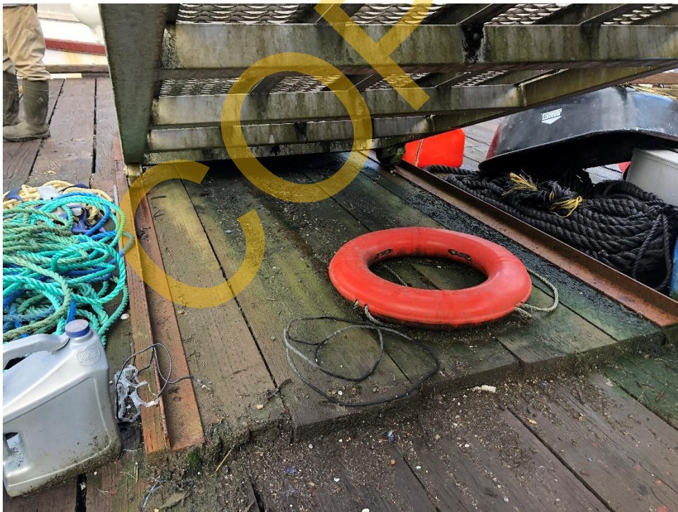
Photo 22 - Gangway slider plate and rollers
