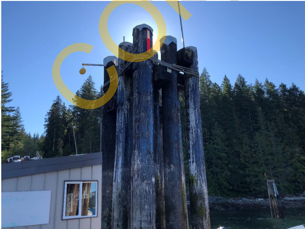
Photo 54 - West end Mooring Piles
