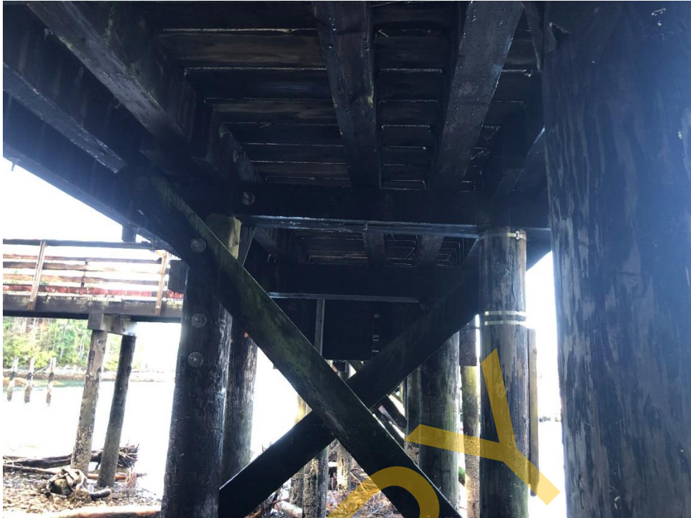
Photo 13 - Pile cap at Bent 4
