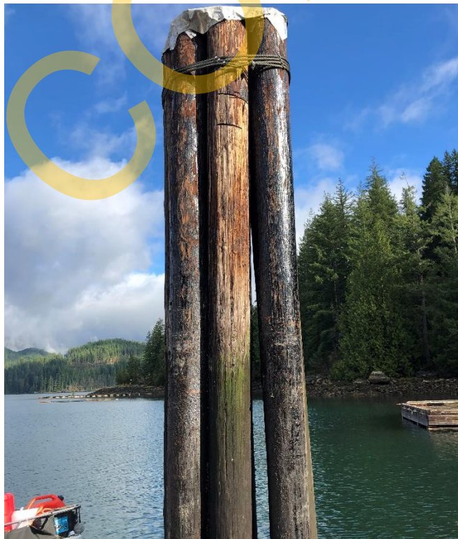
Photo 28 - North Mooring Piles
