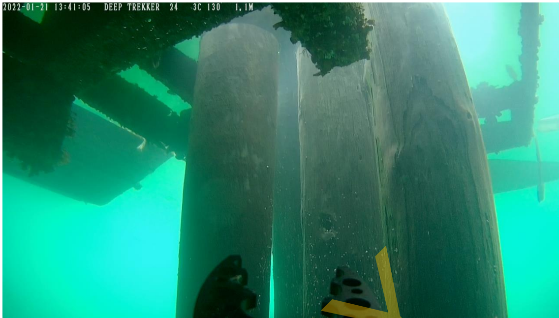
Photo 29 - South Mooring Piles
