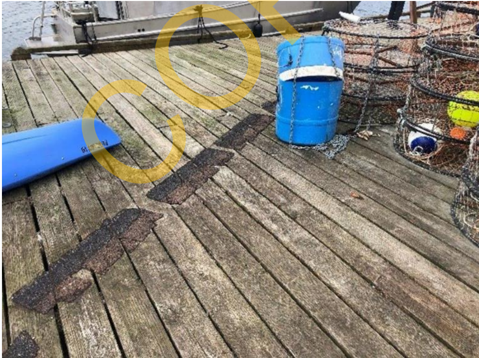
Photo 36 – General view of Float A
