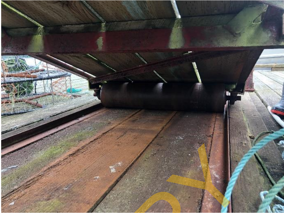
Photo 33 – Gangway Timber Slider Plate and Roller
