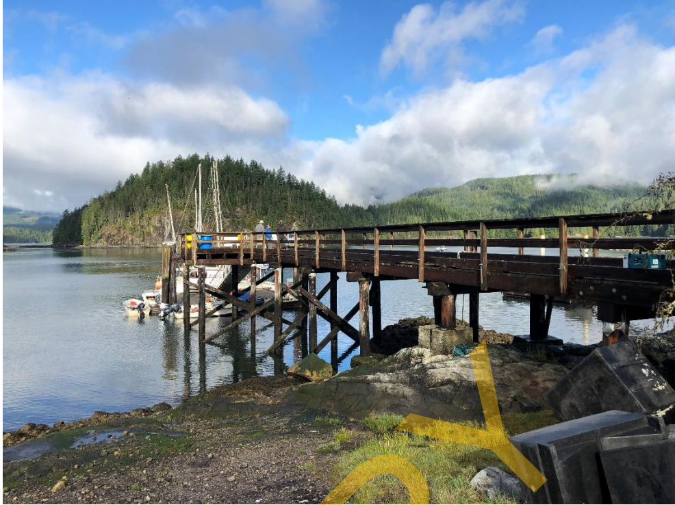
Photo 1 - General View facing West
