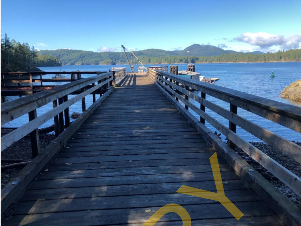
Photo 3 - Wharf Structure Topsides
