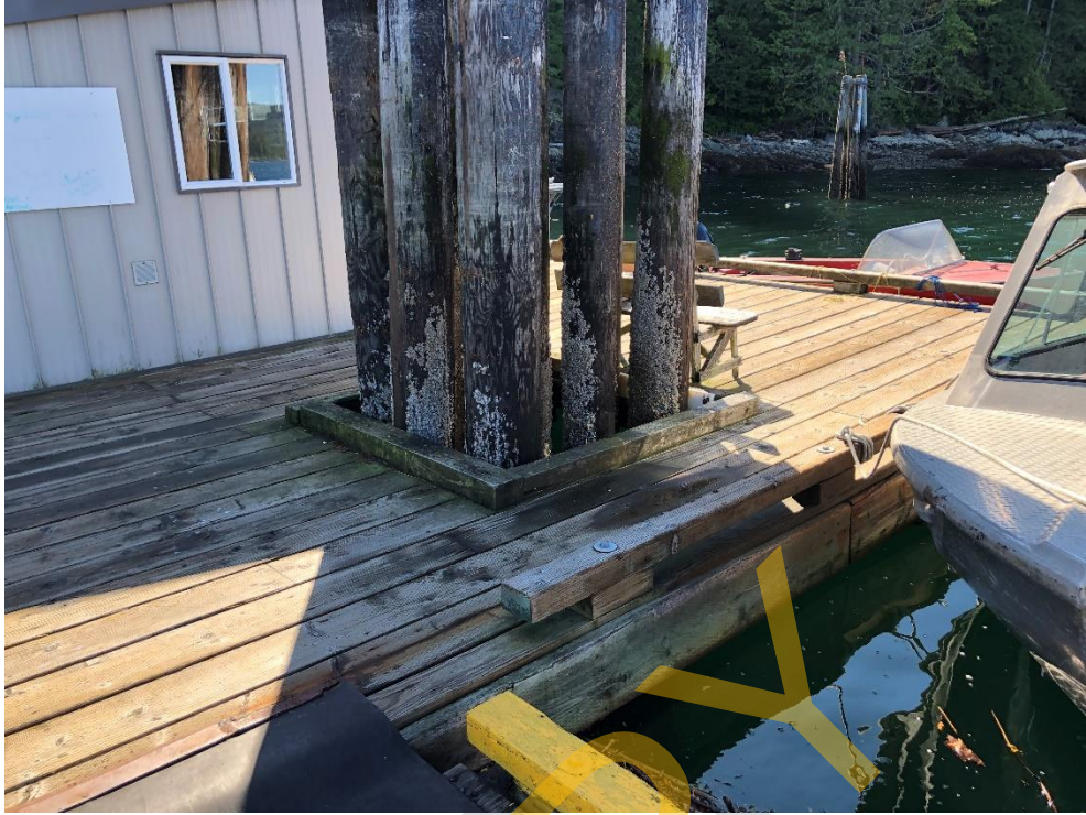
Photo 53 - West end Mooring Piles
