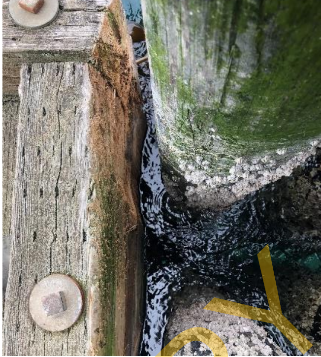
Photo 41 – Wearing to Float A from North Mooring Dolphin
