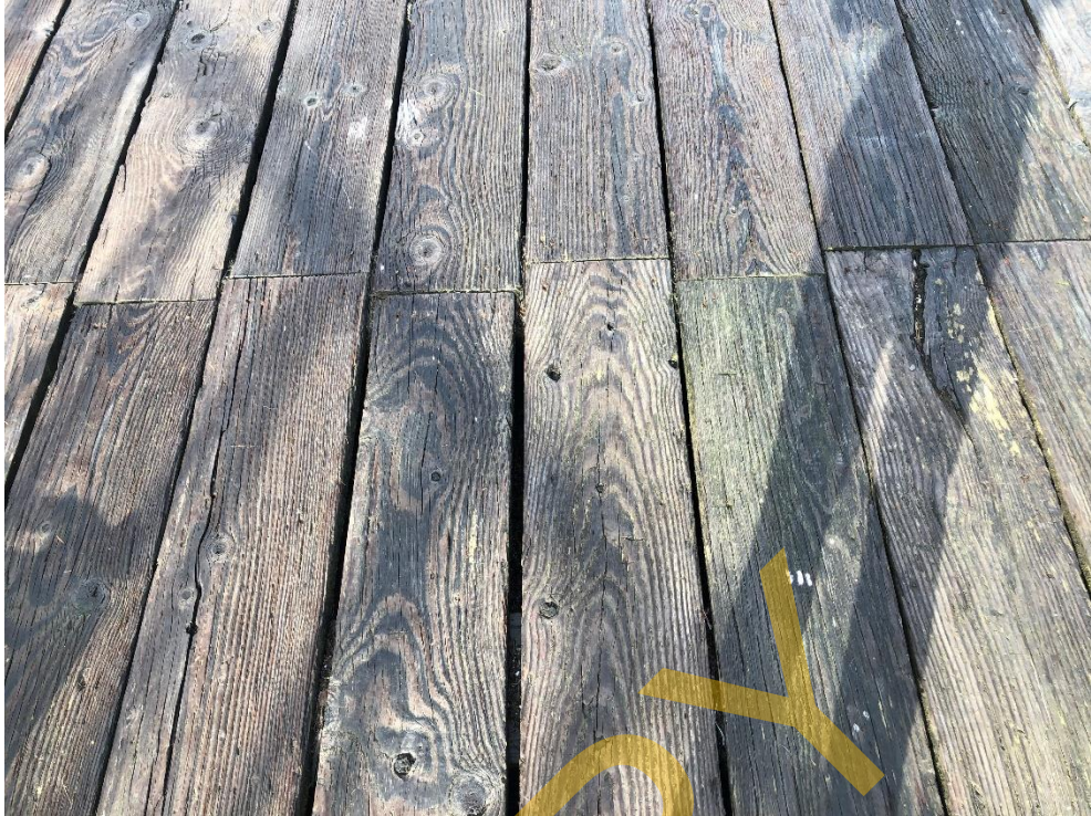
Photo 25 - Typical condition of the timber decking
