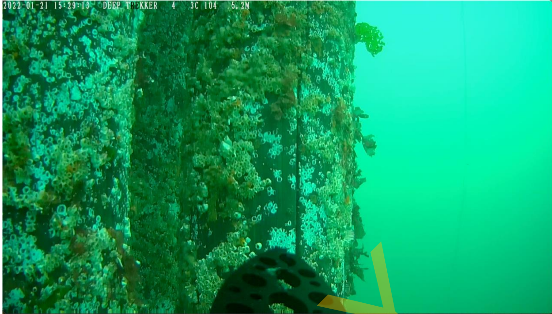
Photo 57 - West end Mooring Piles
