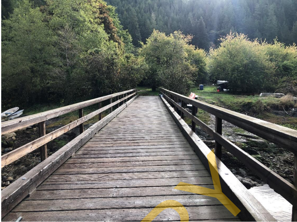
Photo 3 - Topsides of the Wharf Structure
