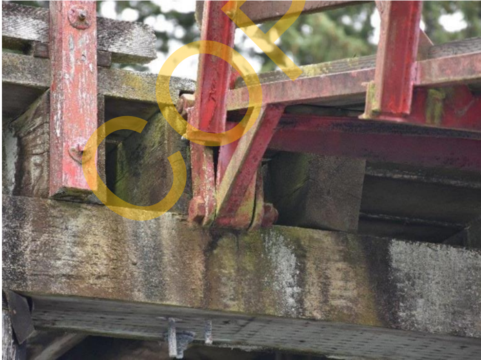
Photo 32 – Gangway Upper Hinge Connection
