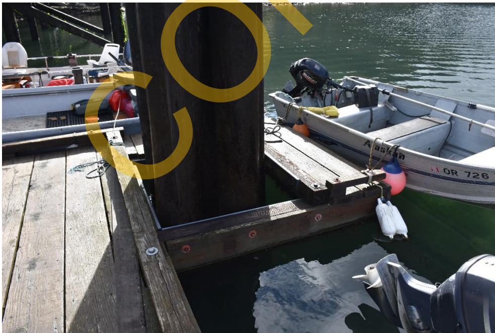
Photo 34 - South Mooring Well with significant flotation loss
