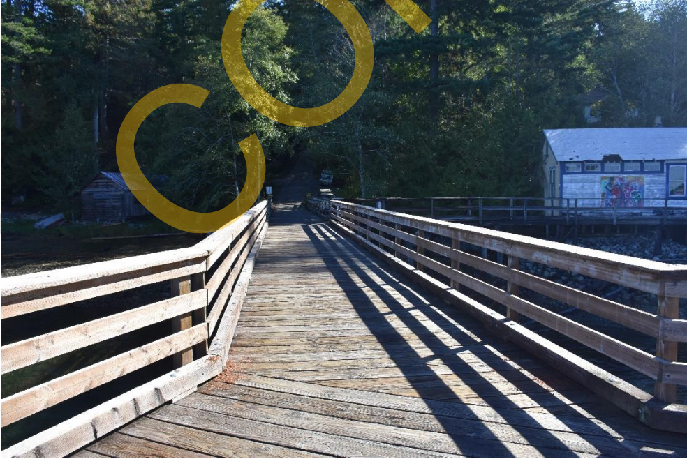
Photo 4 - Wharf Structure Handrails
