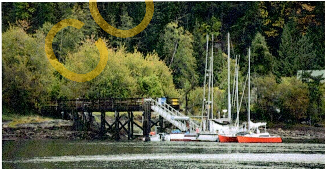
Figure 3 – Owen Bay wharf (McElhanney Engineering Ltd. 2019)
