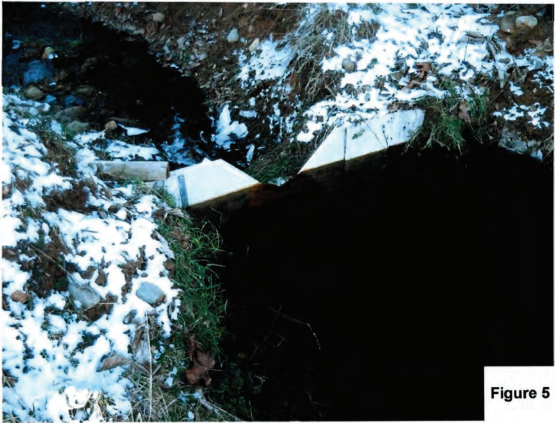
Wier on Drainage Ditch; Top of Brown stain Marks 6.125 inches
