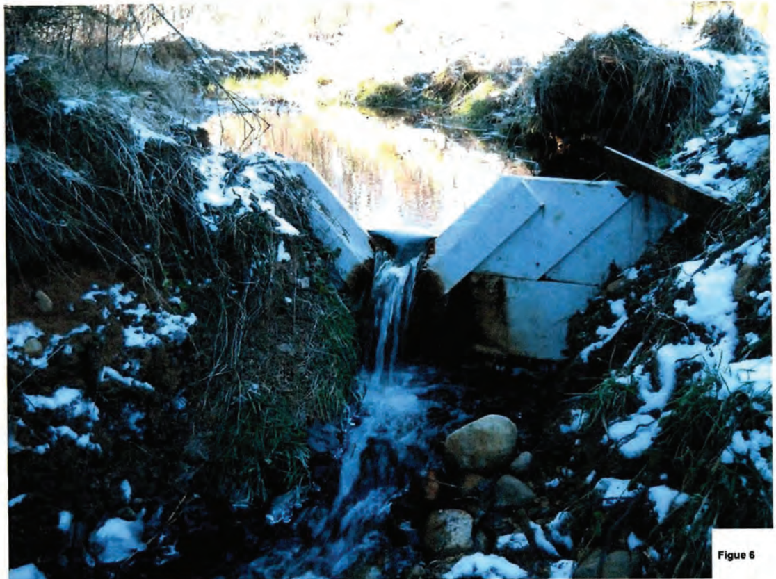
Wier Discharge of 190gpm; February 8, 2019
