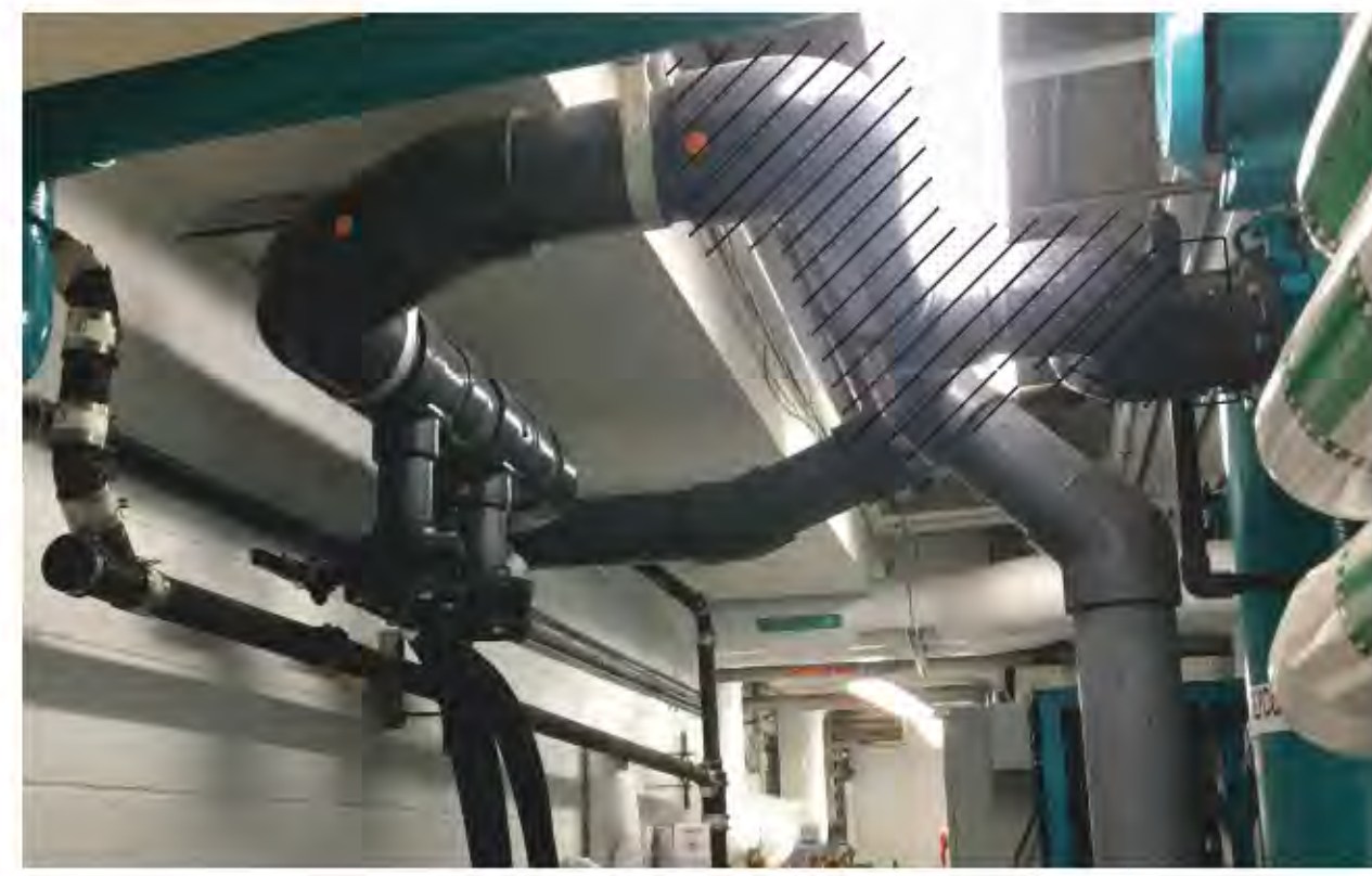
4 EXISTING HYDRONIC LOOP DEMO M4 SCALE: NTS
