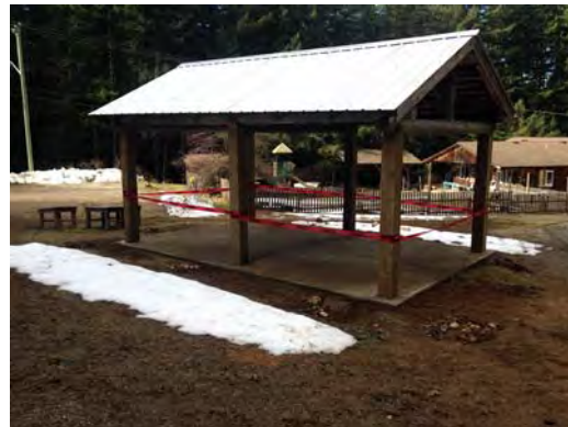
patio structure after
