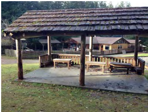
patio structure before
